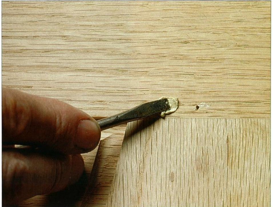
To apply wood putty , press it into the hole with a putty knife or dull screwdriver, leaving a little excess so a hollow won't occur as the putty dries and shrinks.
