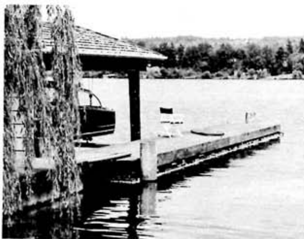
FLOATS ARE ECONOMICAL way to extend solid surface out to water deep enough for diving, boat handling.
