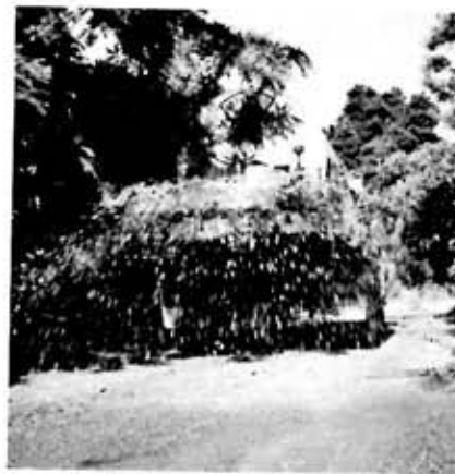
WATERING keeps dust down, softens hard spots during the grading.
