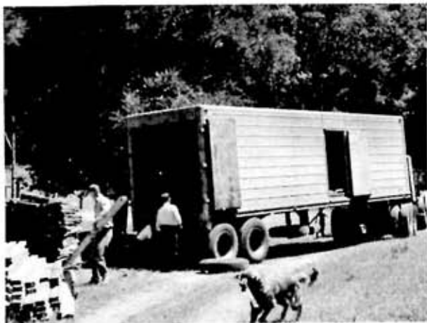
TRUCK UNLOADED pieces a half mile from cabin site. It took 15 loads with a pickup to move it into place. All pieces were in shipment; all fit together well.
