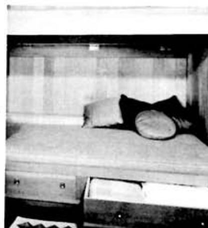
LEFT: When down, bunk is seven-foot lounge. RIGHT: Bunk in raised position is held to wall with heavy butt hinges, locked in place by two \frac{3}{4} by \frac{3}{4} -inch square spring bolts which fit into the wall. Top custom-built mattress is held in place with tabs attached to plywood base. Architect: Joseph Esherick.
