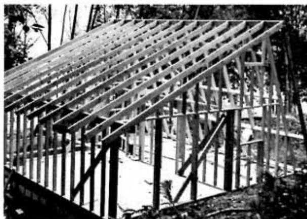
ROOF PITCH is steep. The roof joists are covered with an exterior type fir plywood sheathing.
