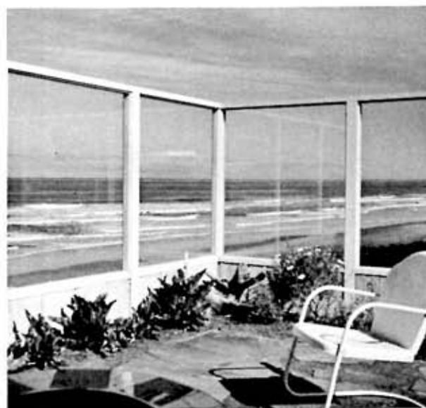
A GLASS wind-protection fence is a good idea for ocean beach cabins. This one is seven feet high.
