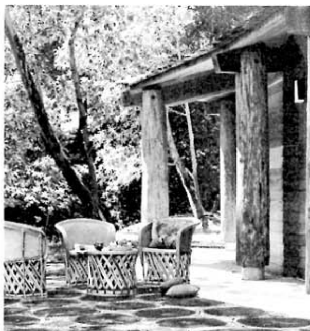
WOOD ROUNDS are the patio floor, set flush with the main slab. Columns on piers to avoid rot, termites.
