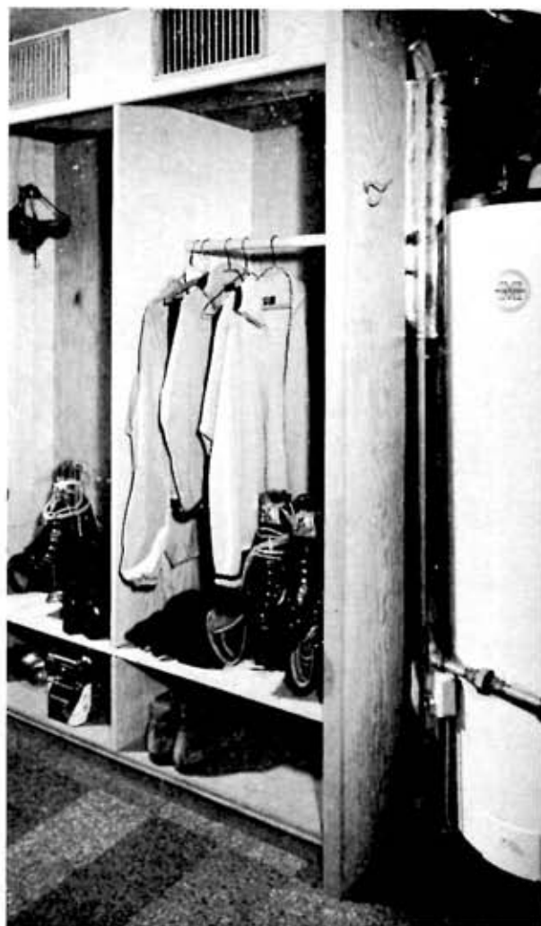
ENTRANCE HALL space next to hot water heater and furnace has built-in closets and shelves, utilizes heat from furnace registers to dry wet clothing.
