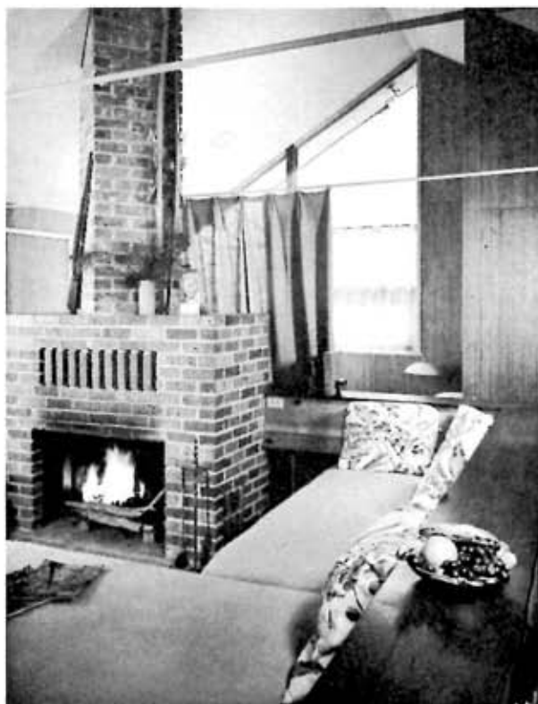
BRICK FIREPLACE set around heat-circulating form. Beds slide to living room to be daytime couches.
