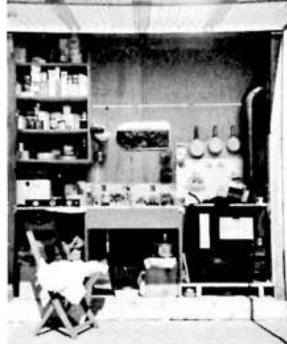
5:00 P.M., SUNDAY. The kitchen-pantry is equipped and ready to use. Corrugated plastic overhead is attached to top of frame with piano hinges.
