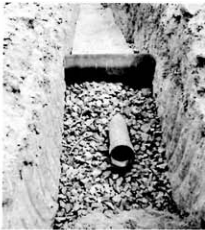
TILE COVERED with 3 inches of gravel, then asphalt paper goes in.
