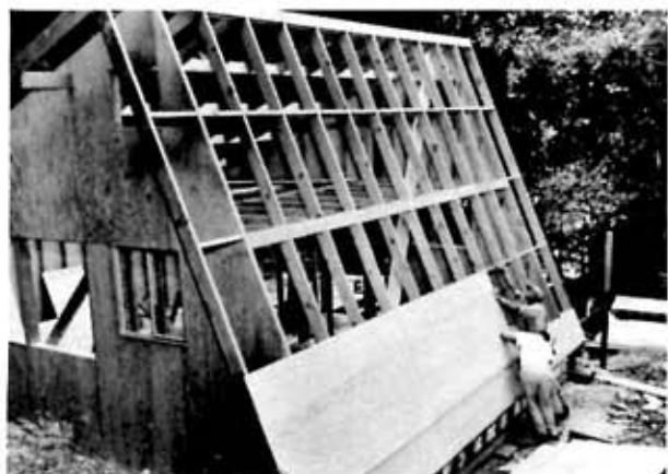
PANELS are lapped over lower sections. The simple design allows for some off-site fabrication.
