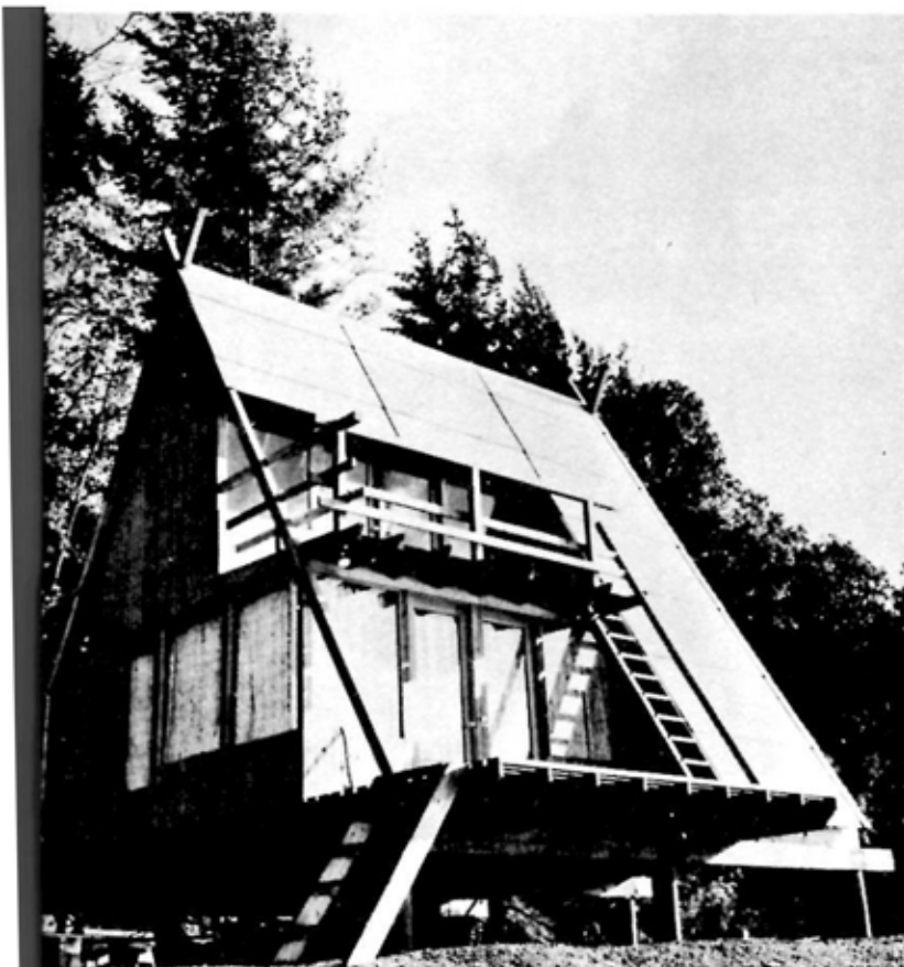
FRONT VIEW of cabin. Stairway at right of windows has hand rail for safety, leads from lower to upper deck.
