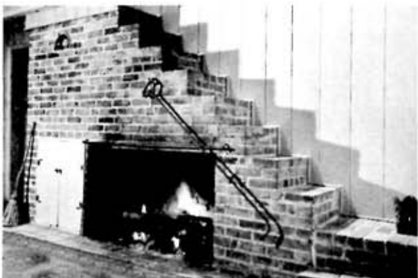
BRICK masonry is set in steps, used as stairway to sleeping quarters. Rod above opening for fire screen.
