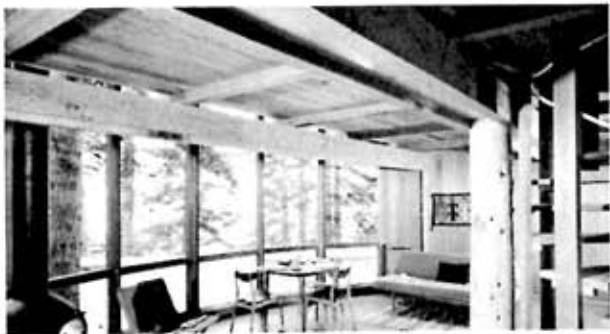
PEELED POST is central roof support. Stairs lead from living area to sleeping balcony.
