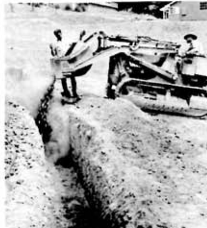
TRENCHES BACK-FILLED with gravel to a depth of a foot, leveled.
