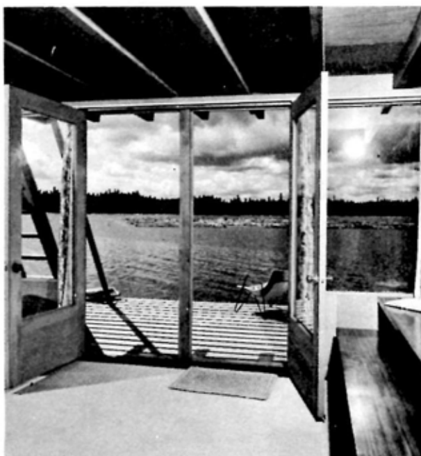
DECK EXTENDS nearly 9 feet past cabin door. Lumber for the 16-foot-wide deck is 2 by 6's, spaced \frac{1}{2} inch.
