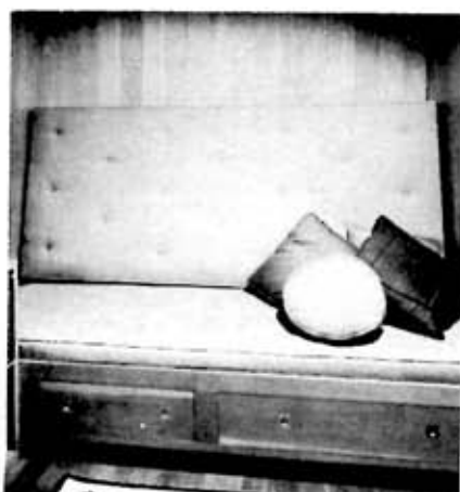
LEFT: When down, bunk is seven-foot lounge. RIGHT: Bunk in raised position is held to wall with heavy butt hinges, locked in place by two \frac{3}{4} by \frac{3}{4} -inch square spring bolts which fit into the wall. Top custom-built mattress is held in place with tabs attached to plywood base. Architect: Joseph Esherick.
