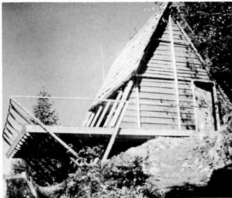
PUP-TENT shape was easy to frame. All uprights were cut from trees on the site. Cabin sleeps six.
