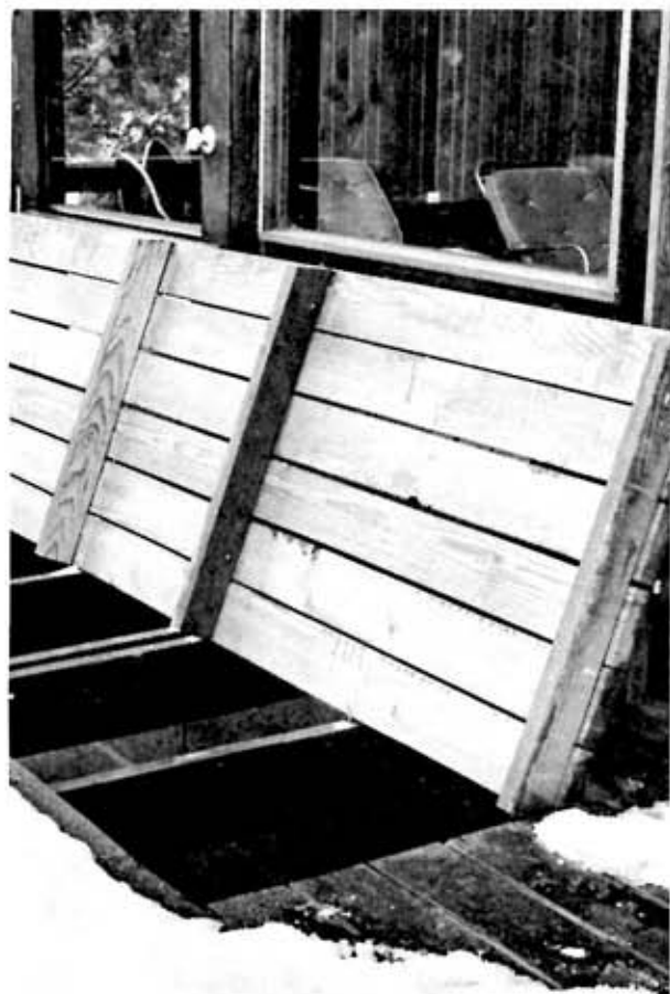
TIPPED UP deck section protects full length glass door and windows from weight of piled up snows and water seepage. Fold section down during the summer.
