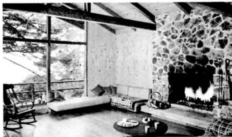
MASSIVE FIREPLACE has heat vents in sides, a major source of warmth in the cabin. Intakes are near floor level; outlet vents are just above damper level.
