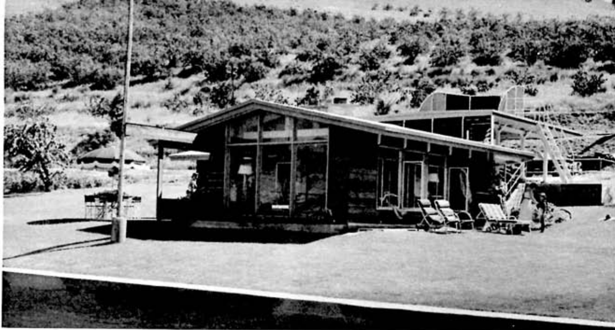
SUN DECK built at back of cabin, above car port, has canvas laced on a pipe frame for sun and wind control.
