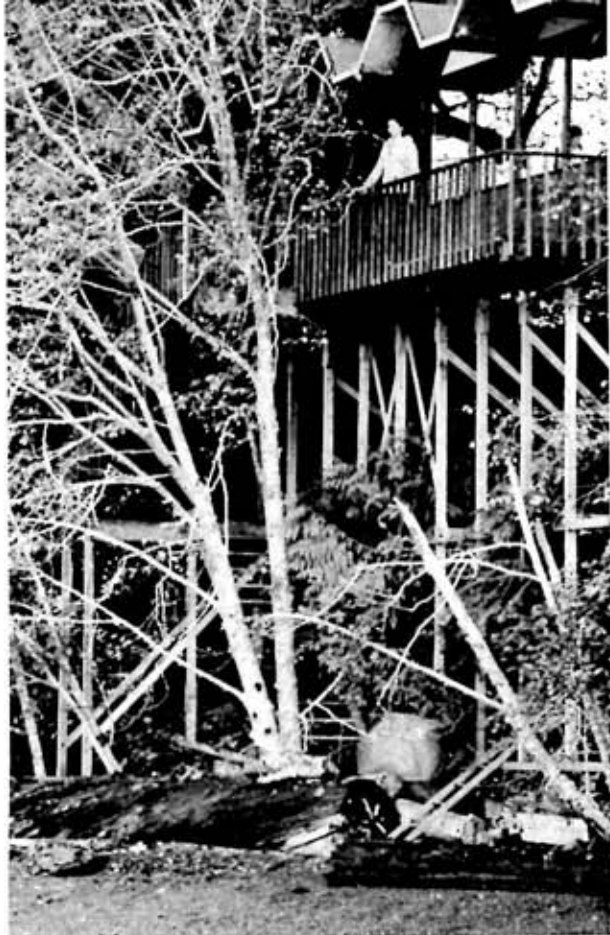
36-FOOT DECK runs along front of cabin. Underneath, hollow-box beams rest on stiltlike underpinning; at rear they rest on hillside. Note stairs at left.
