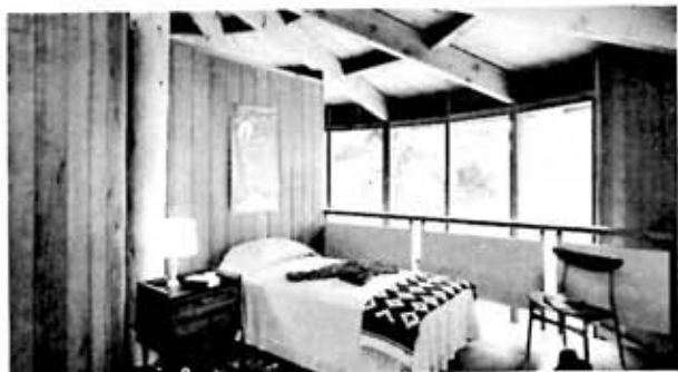
BALCONY BEDROOM privacy is enhanced by plywood panels set in rail. Wall (left) hides stair.
