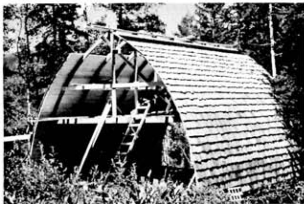
CONSTRUCTION: Curved glue-laminated arches form rigid trusses with floor joists. Interior walls optional.
