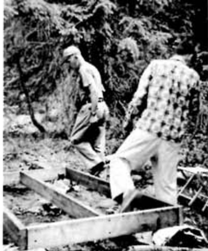
10:45 A.M., SATURDAY. The owners started with the cabin's simple wood foundations. A tent (not shown) was used as a "construction camp."
