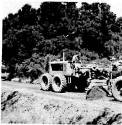
FIRST STEP is grading, best done with large equipment in most cases.
