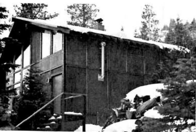
BIG PLYWOOD PANELS give air of snug solidness to the cabin. Cutback eaves lessen snow load on roof.
