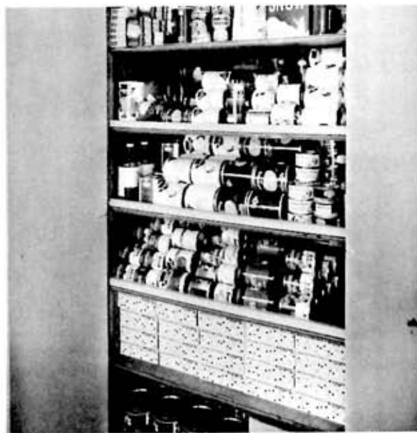
QUANTITY STORAGE for case lots of food is increased by stacking cans on sides. A lip on the shelves holds cans in. Architects: Hamlin and Martin.
