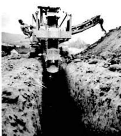
DRAIN FIELD trenches, 3\frac{1}{2} feet deep, are best dug with power.
