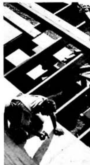
LEFT: Foundation has nine concrete piers in rows of three, 12 feet apart. Each row supports an 8 by 10-inch beam 28-feet long. Professional help is advised.
