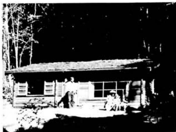
FINISHED CABIN —later a fireplace was added to end wall at right. Owners cut trees to make the clearing. Weed killer was used to keep stumps flush with ground.
