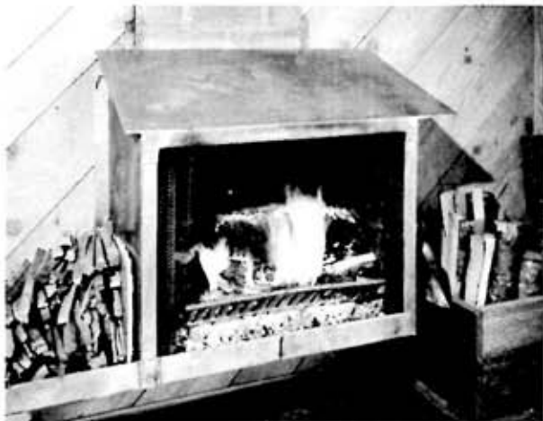
COPPER fireplace hangs from masonry chimney, keeps entire cabin warm most months. Design: Alan McRae.
