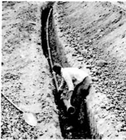
DRAIN TILE is laid atop gravel bed. Joints are just slipped together.
