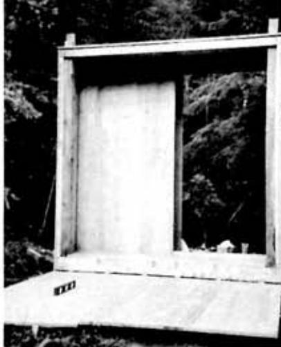
3:30 P.M., SATURDAY. Walls, ceiling are in place. Combination folding wall and deck hinged to bottom of frame which sits level on concrete blocks.
