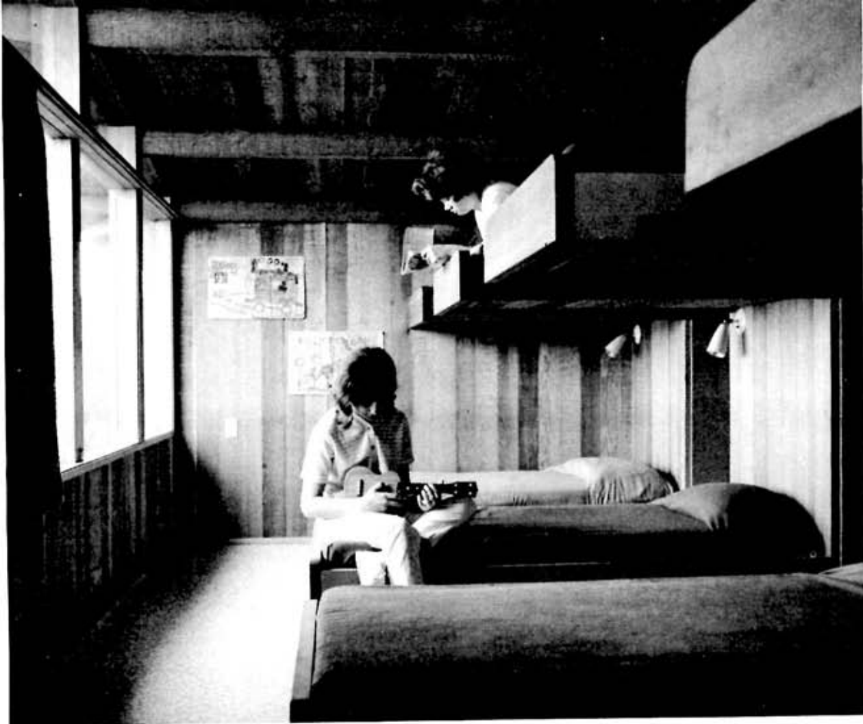
FOUR SETS of bunks provide dormitory-type sleeping accommodations. Upper bunks, cantilevered from tops of built-in closets, are set back from bunks below by a third of their length. No need for support posts.
