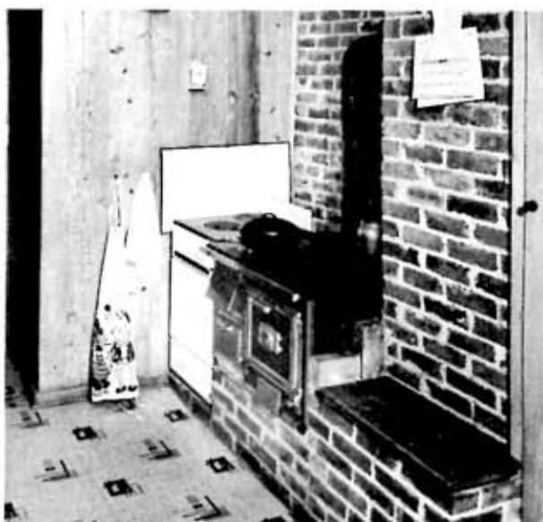
COMBINATION of wood stove and small electric unit provides quick emergency heat plus old-fashioned comfort. Wood storage is under hinged seat (right).
