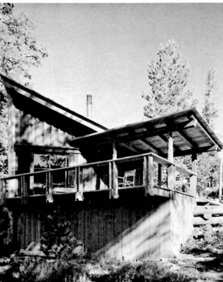
BOAT STORAGE area is under the deck. Timbers are extra heavy scale to support possible 18-foot snow load.
