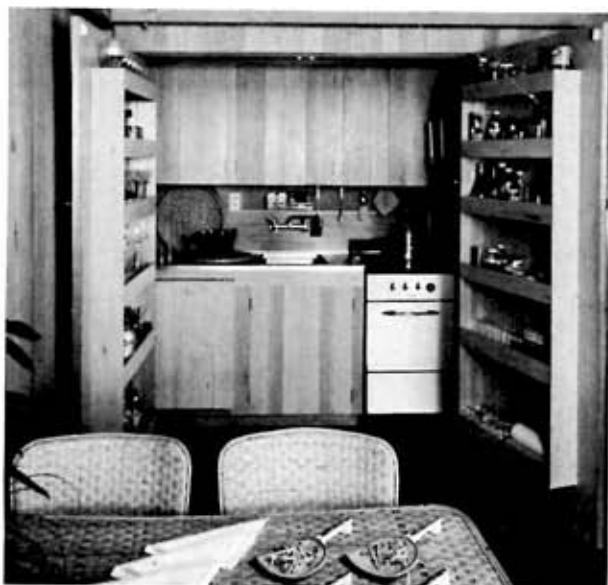
TWO LARGE DOORS with built-in shelves open off big room, revealing small kitchenette with sink and stove. Shelves are lipped so cans won't fall off.
