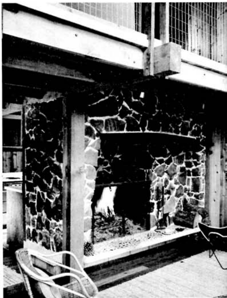
MASSIVE FIREPLACE , of stone from the site, with its cantilevered hearth, is winter gathering place.
