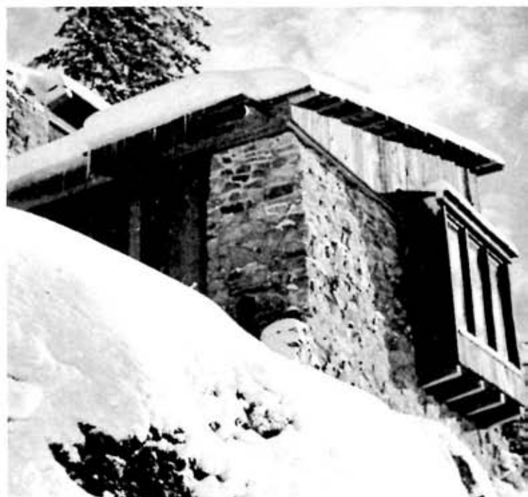
STONE WALLS have natural insulating properties that make a cabin warmer in winter and cooler in summer.
