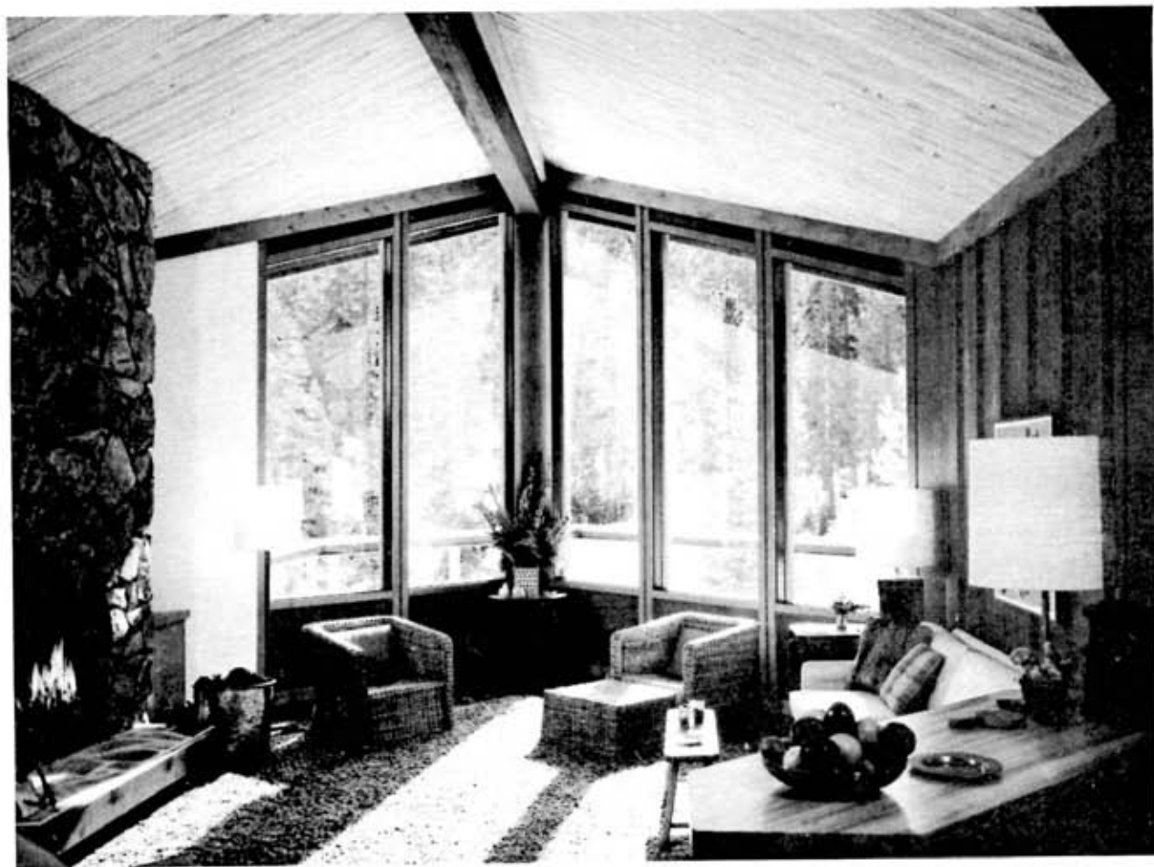
LIVING ROOM LOWER than rest of main floor by two steps to gain vertical space. Ceiling throughout is edge-laid 2 by 4's. All colors chosen to match rocks, plants, trees native to the beautiful site.
