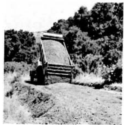
RED ROCK is spread 4 inches thick atop the graded road, then smoothed.
