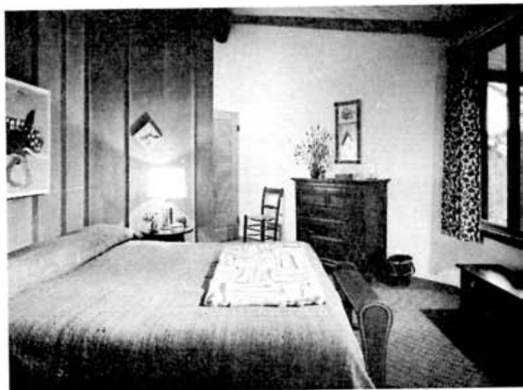
TRIANGULAR BATTENS on master bedroom inside wall match the exterior siding of the house.
