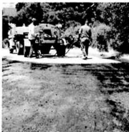
PENETRATING OIL or other surface is put down to finish road.
