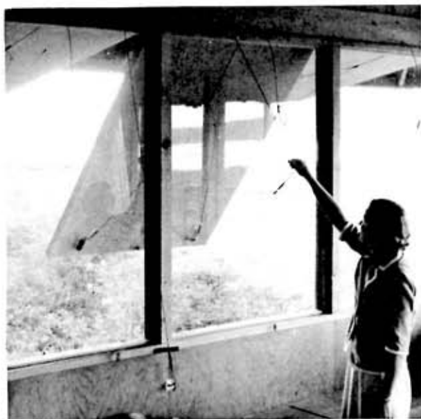
WOOD PANELS tuck under eaves when cabin is in use, are easily lowered to close vacant cabin tight.
