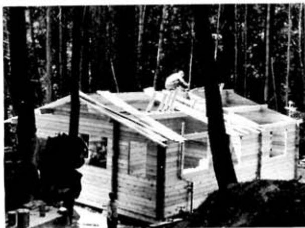
FINAL STAGE —as roof sheathing goes on. Pipes are on outside of single wall construction. Permanent camp was used while the cabin was being built.
