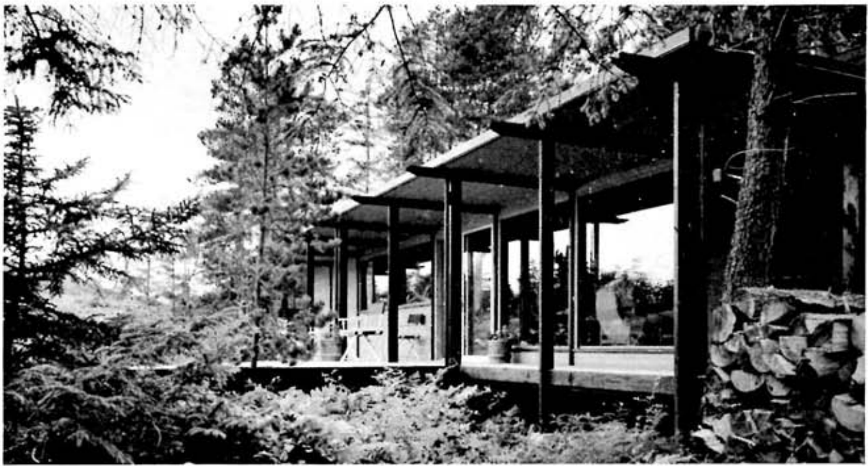
DECK ROOF SUPPORTS are paired 2 by 4's secured on either side of 2 by 6-inch vertical supports. The horizontal pieces pierce the walls, extend into rooms, as photo of living room (below) demonstrates.
