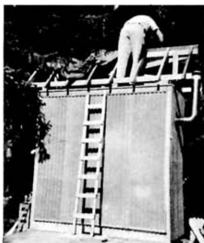
PLASTIC PANEL is folded down while the roof work is finished. Roof framing was all pre-cut and ready to put in place to speed up this task.
