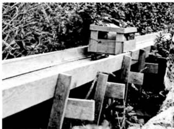
CABLE CART moves supplies down to cabin from road above. Box has wheels, is kept on track by sides of chute. Electric winch at top operates cart.
