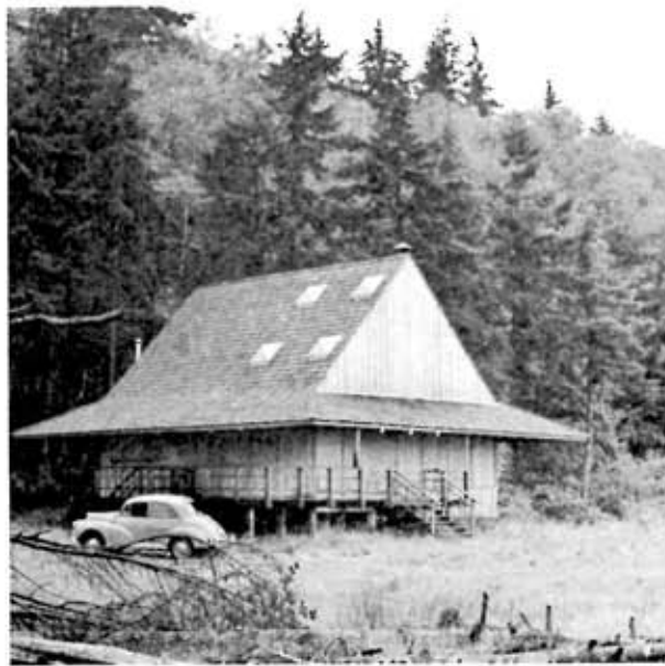
SKYLIGHTS in roof are visible in this view of cabin after owners have closed it before leaving.
