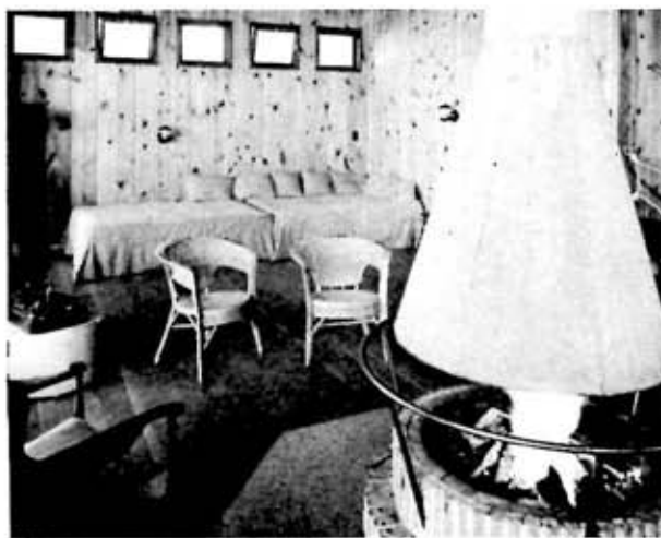
GALVANIZED HOOD of expanded shale block fire-place drops down to start fire and to contain coals at night.
