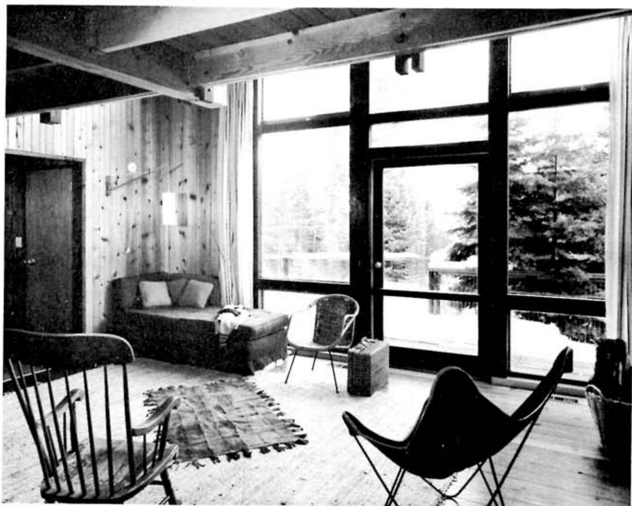
TWO-STORY WINDOWS open onto deck overlooking the lake. They provide light for living area, dormitory. Drapes conserve heat in winter. Small ventilation panels left and right of the door.
