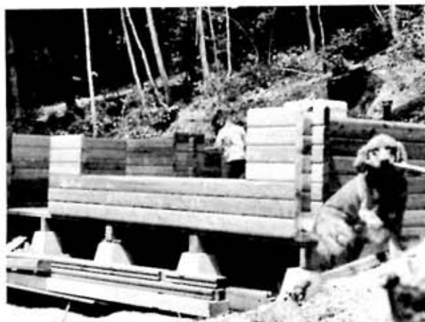
FOUNDATION is ready-made concrete piers set on concrete poured in holes dug down to a solid base. Note how corner pieces overlap. Dog was good tool carrier.
