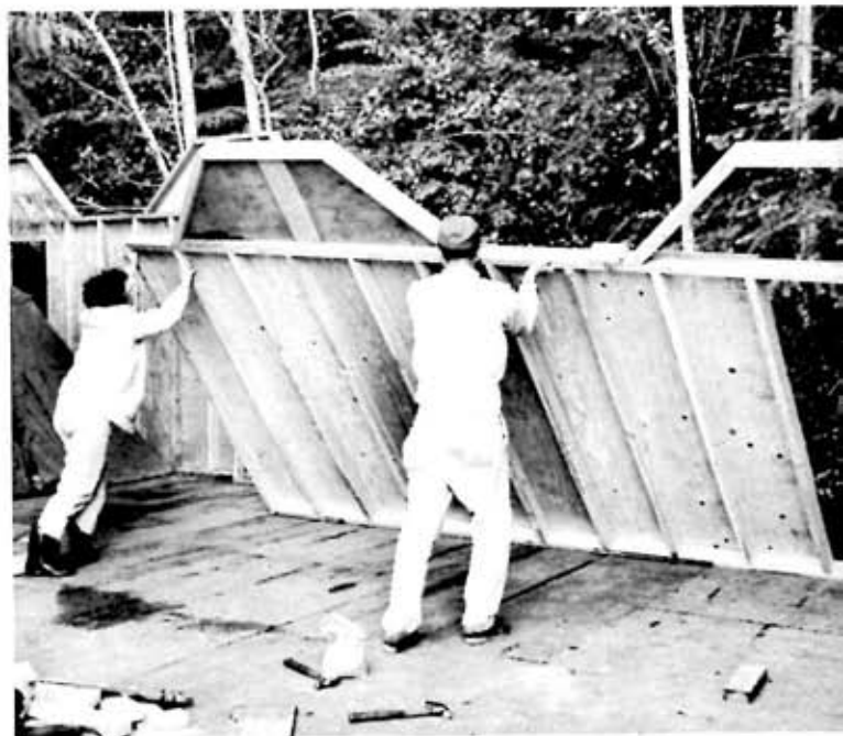
WALL SECTION components were nailed together on cabin floor, tilted up and propped in place for nailing. There was no electricity so power tools weren't used.
