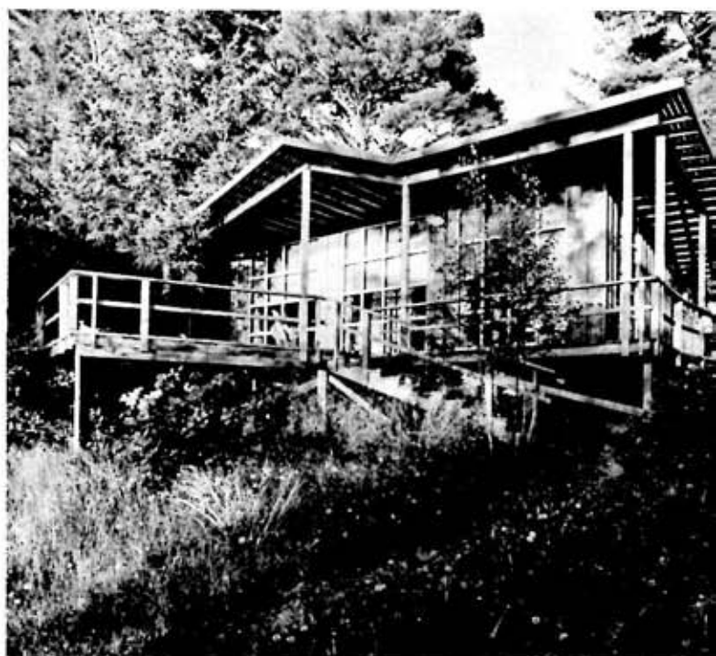
FROM THE LAKE side showing the deck. The latticed extension of the roof overhang helps shade the windows.
