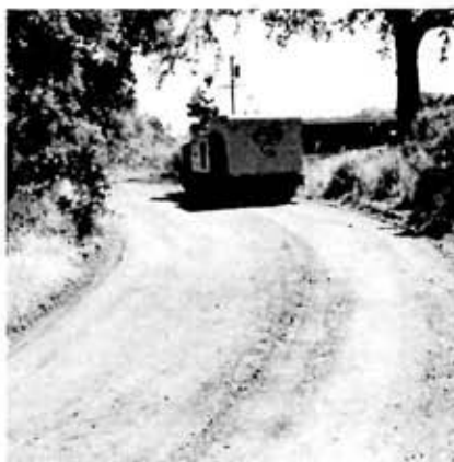
ROLLER COMPACTS rock, after which road is usable by automobiles.
