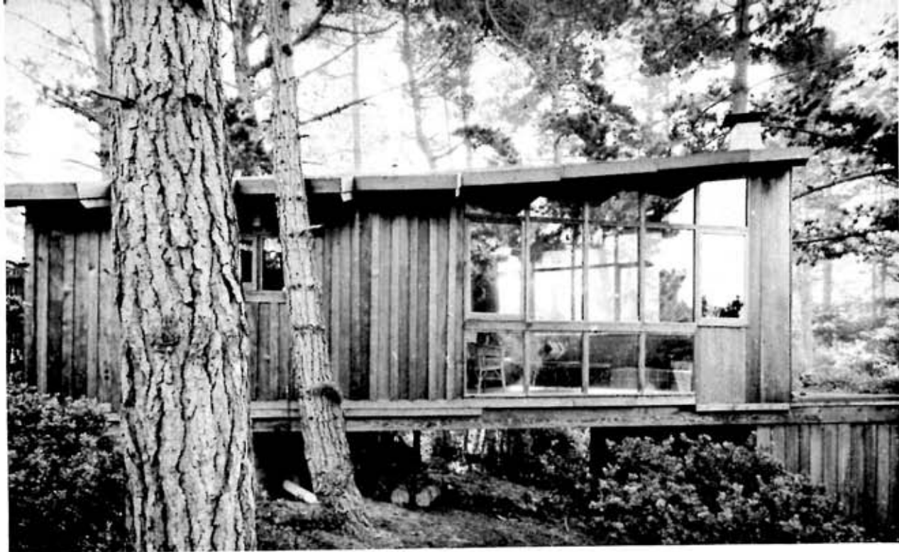
FIREWOOD is stored in open area under the cabin. Note enclosed storeroom at the far right, lower corner.
