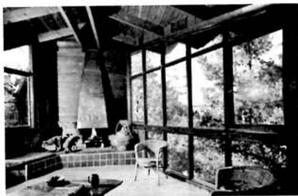
FIREPLACE has raised tile hearth that's also a seat.
