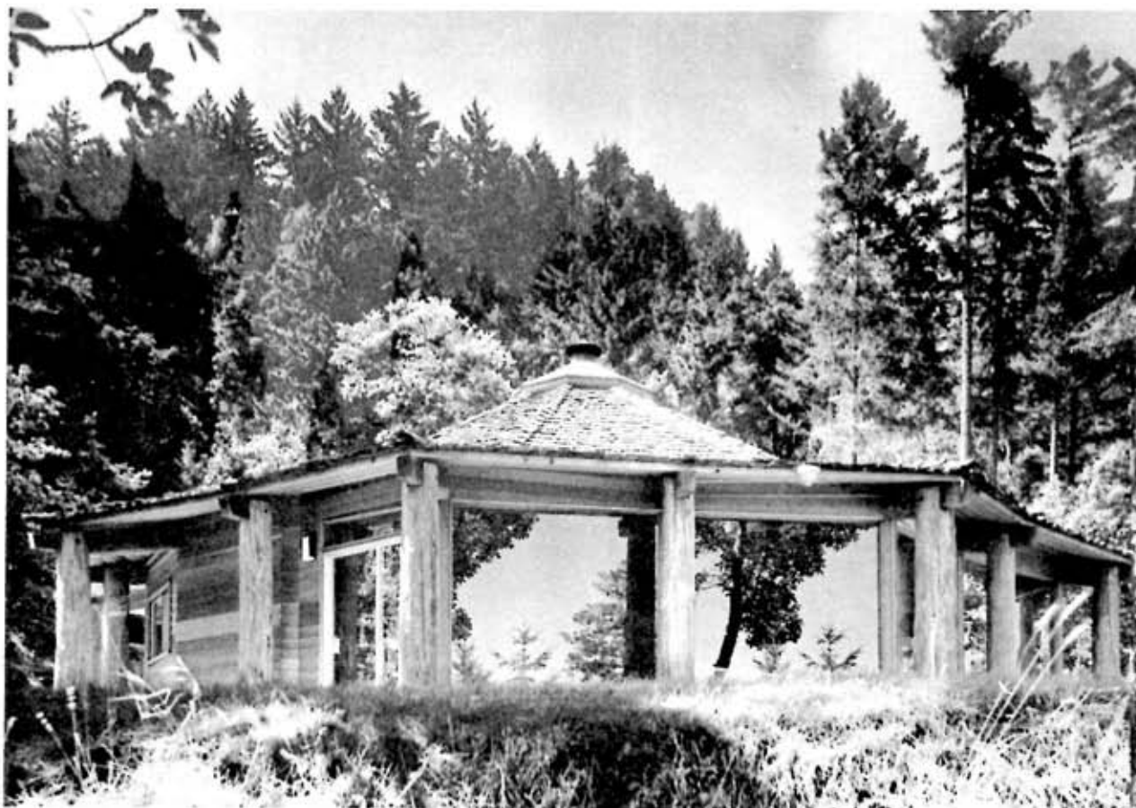
WIDE ROOF OVERHANG cools the house on warm summer days in the Round Valley area of California's Eel River basin. The major glass areas face east to minimize glare. A skylight balances light.
