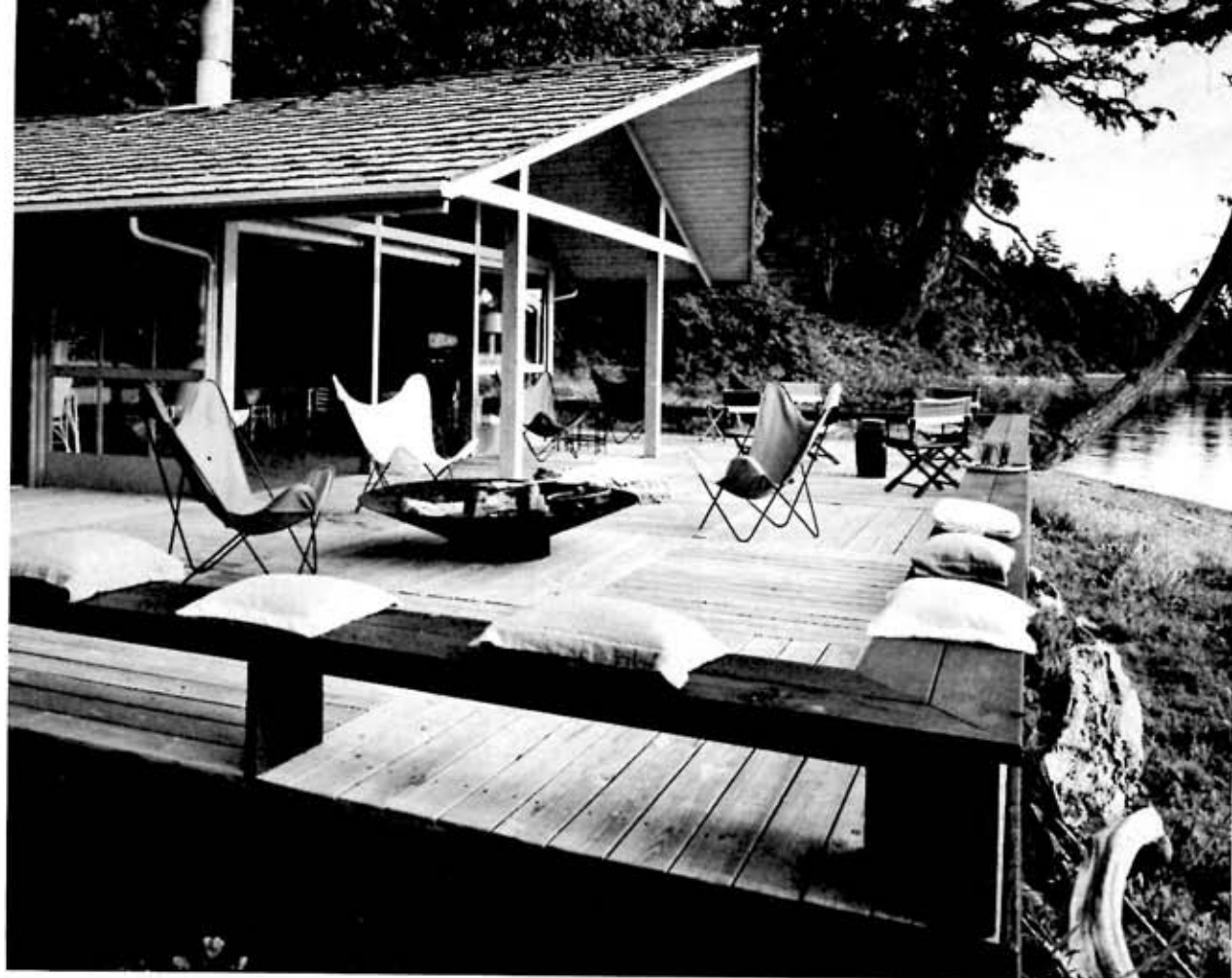
THE LARGE deck was laid parquet style in 3-foot squares. 15-inch-high seat rail is of 2 by 8-inch boards.
