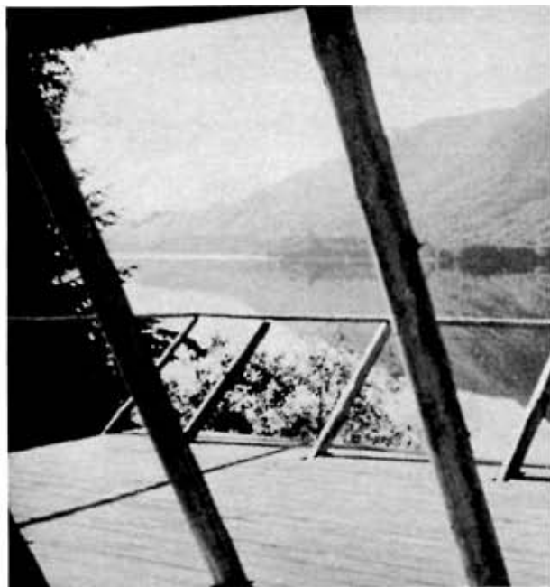
THE OPEN deck flooring drains water. Rail posts come up through the deck from the foundation below.
