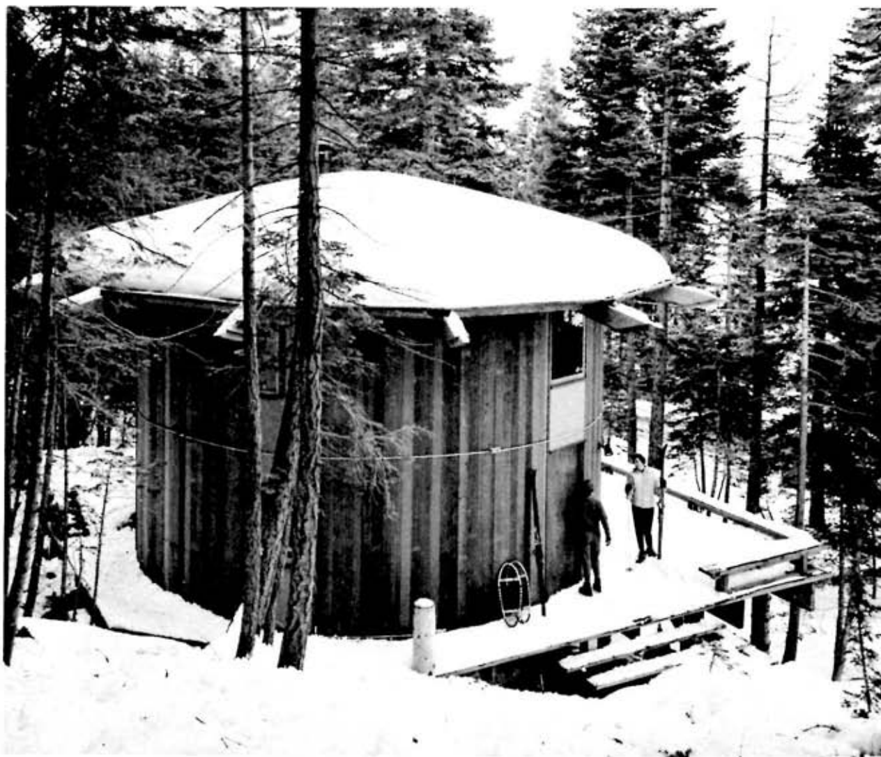
CABIN RESTS ON PLATFORM , its window wall faced to the view, its entry on the lee side during most storms. The redwood wine tank is thick enough to provide adequate insulation for winter use.
