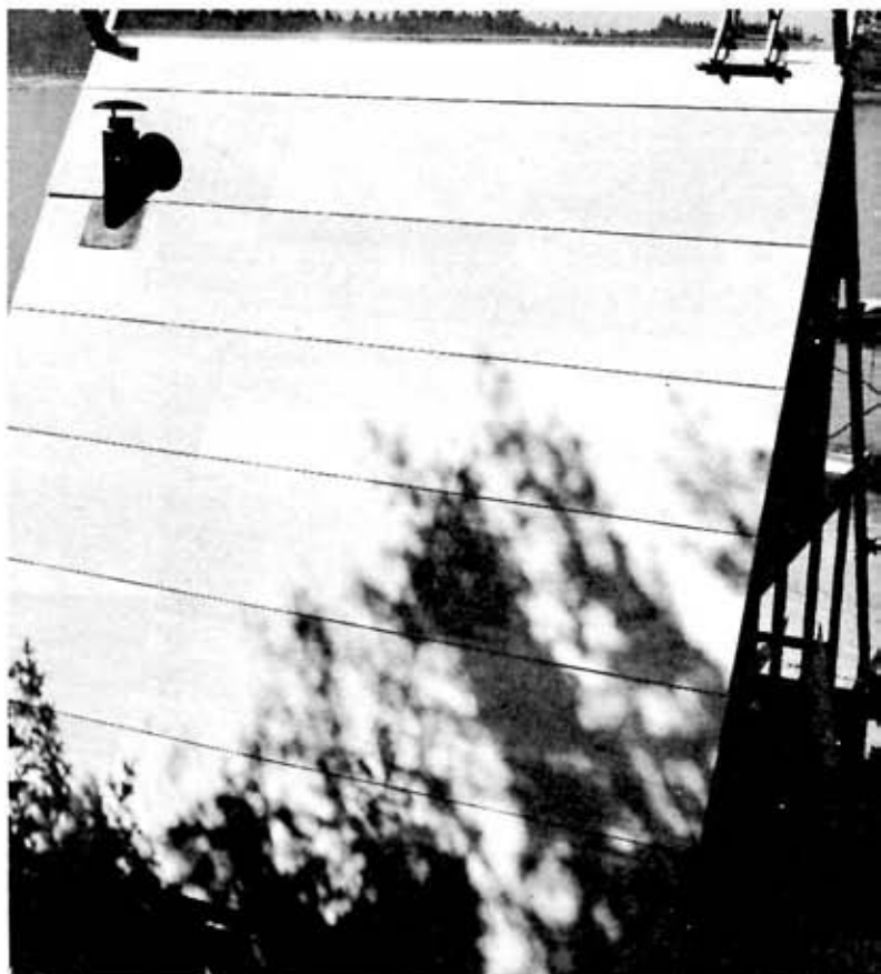
REAR VIEW shows roof of \frac{3}{8} -inch exterior type fir plywood panels lapped like giant shingles.
