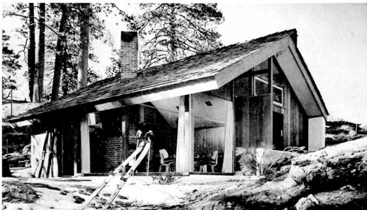
WOODED VALLEYS , pine covered hills and sky above San Bernardino mountains are three walls of this interesting cabin. Ceiling follows pitched roof and the glass disappears into the ceiling without interruption.
