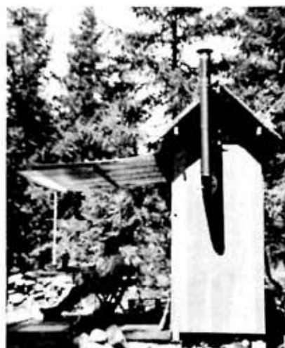
THE CABIN in action: Roof over the "front porch" is supported by two aluminum poles. Bedroom addition is identical but on other side of the frame.
