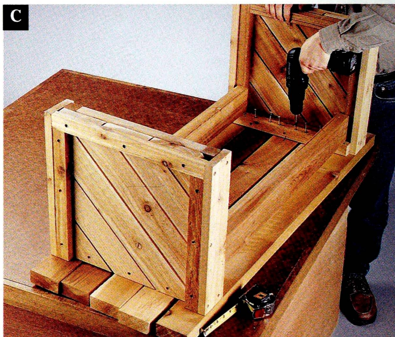
C Use shelf slats to set the correct distance between the end-frame assemblies, then attach the end frames to the bottoms of the seat slats.
