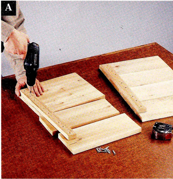
Attach the side cleats flush with the tops of the side boards.
