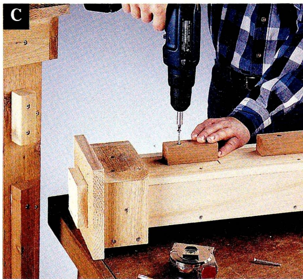
Attach the short post cleats 3\frac{3}{8} " up from the tops of the long post cleats. The top stringers on the panels fit between the cleats when installed.
