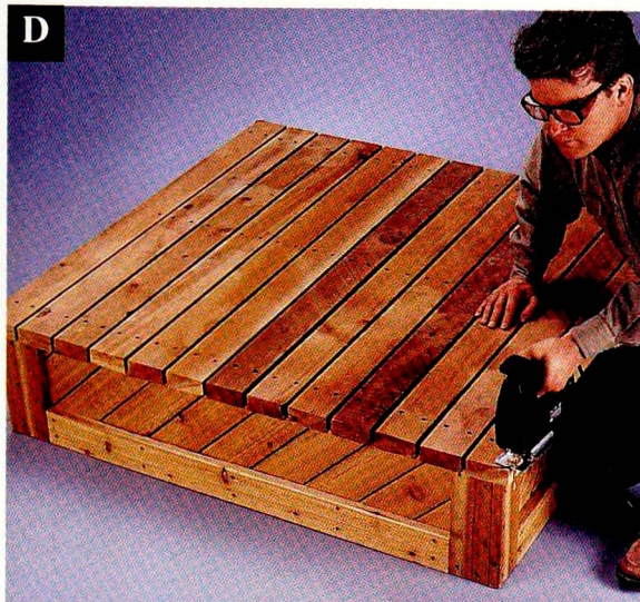
D Cut roundover curves at the corners of the outside deck slats, using a jig saw.
