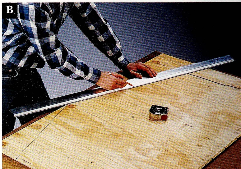
B Lay out the roof angle on the side panels using a straightedge.
