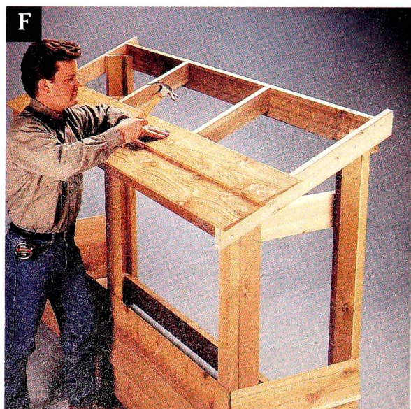
Attach the roof strips with siding nails, starting at the back edge and working your way forward.
