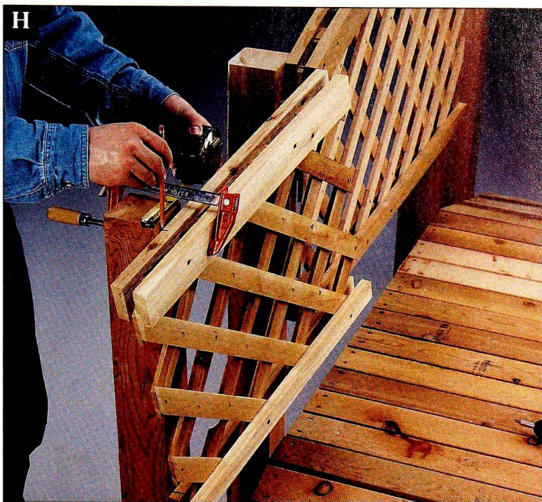
Clamp the rough end panels to the posts at the ends of the bridge, and draw alignment markers so you can trim them to fit exactly.
