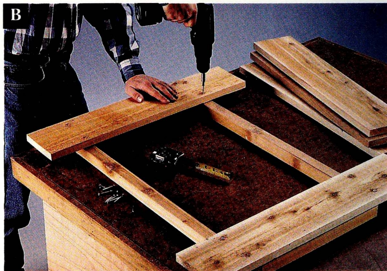
B Attach a slat at each end of the panel frame so the outer edges of the slats are flush with the outer edges of the frame.
