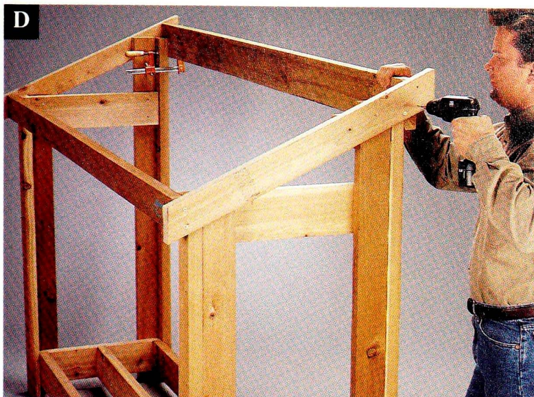
Attach the front rail by driving screws through the outer roof supports, making sure the top of the rail is flush with the tops of the supports.
