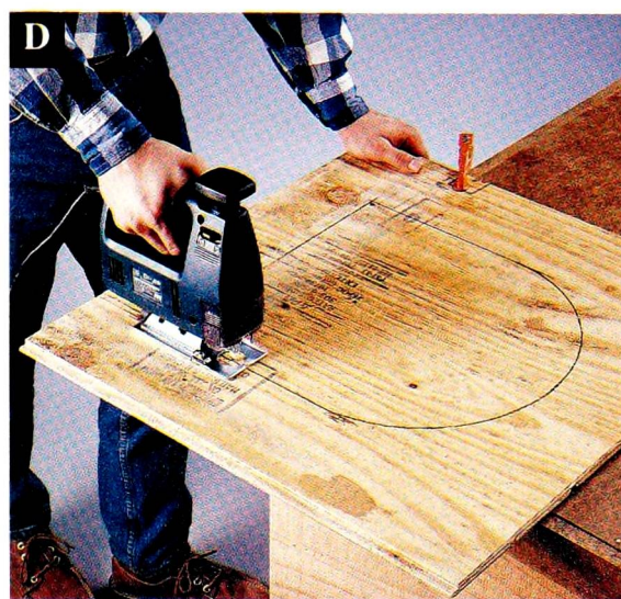
Cut out the openings in the panels with a jig saw.
