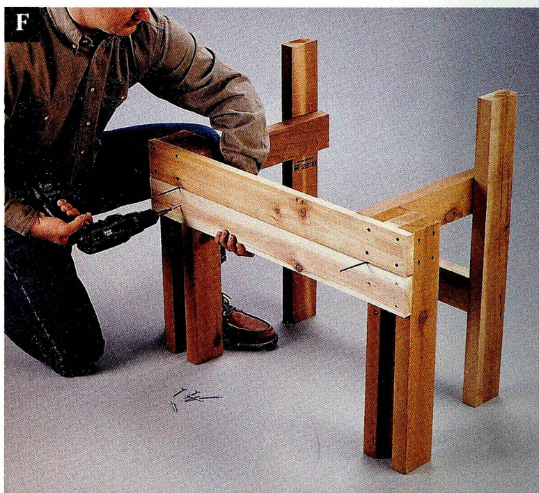
The shorter face boards for the tall benches are attached so the ends are flush with the outsides of the doubled posts.
