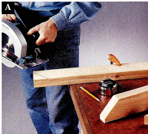
Make triangular cutoffs at the ends on the table stringers, using a circular saw.
