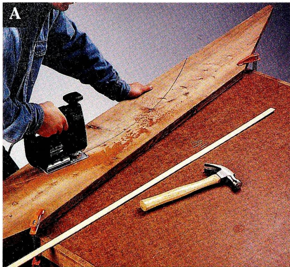
Use a jig saw to make the arched cutouts in the bottoms of the 2 × 10 stringers.
