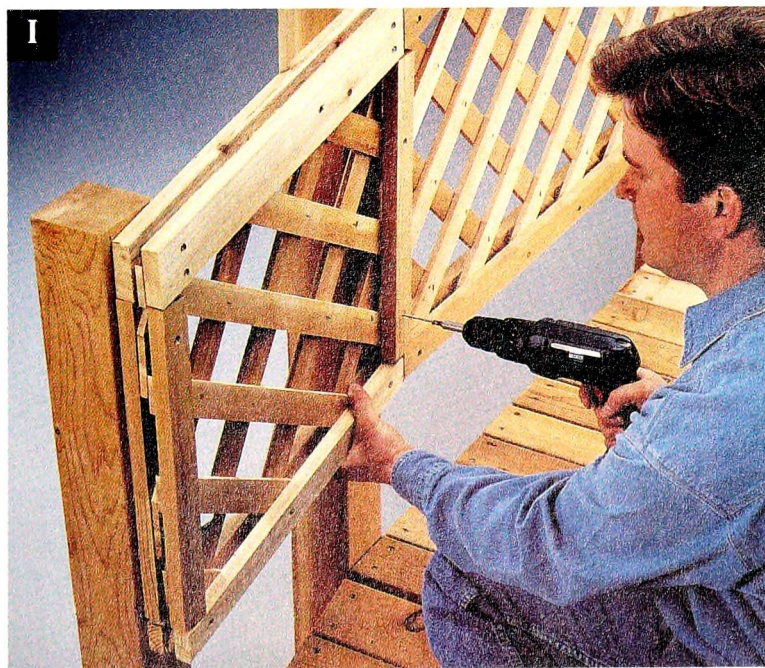
Use deck screws to attach a trim strip over each joint between the end panels and center panels.
