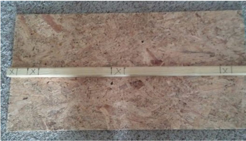
Figure 8: Layout: notice the beginning has two |X marks|. In between is where your filler block will go. Measure 15 \frac{1}{4} from the end of the board and then from the third |X| measure 16 for the rest of the wall.
