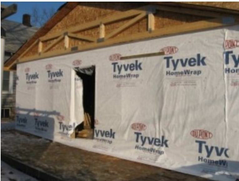
Image 8: Tyvek Door Opening (Master Touch Custom Homes)
