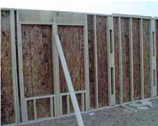
Image 6: See the 2x4s that have three 2x4s running perpendicular to the studs in the walls? That is the wall tie. (Reference Image 7 for creative commons license).
