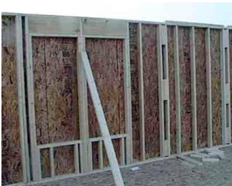
Image 7: Complete Header—Also shows a completed wall with rough opening for two windows. (Marshall Brian, How House Construction Works, April 1, 2000. Creative Commons License.)
