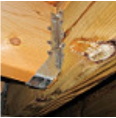
Image 5: Joist Hanger and Double Rim Joist (Creative Commons Credit: ArmchairBuilder.com)
