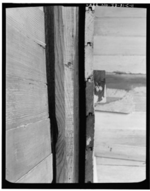
Image 9: Tongue and Groove Siding (NPS Public Domain License)
