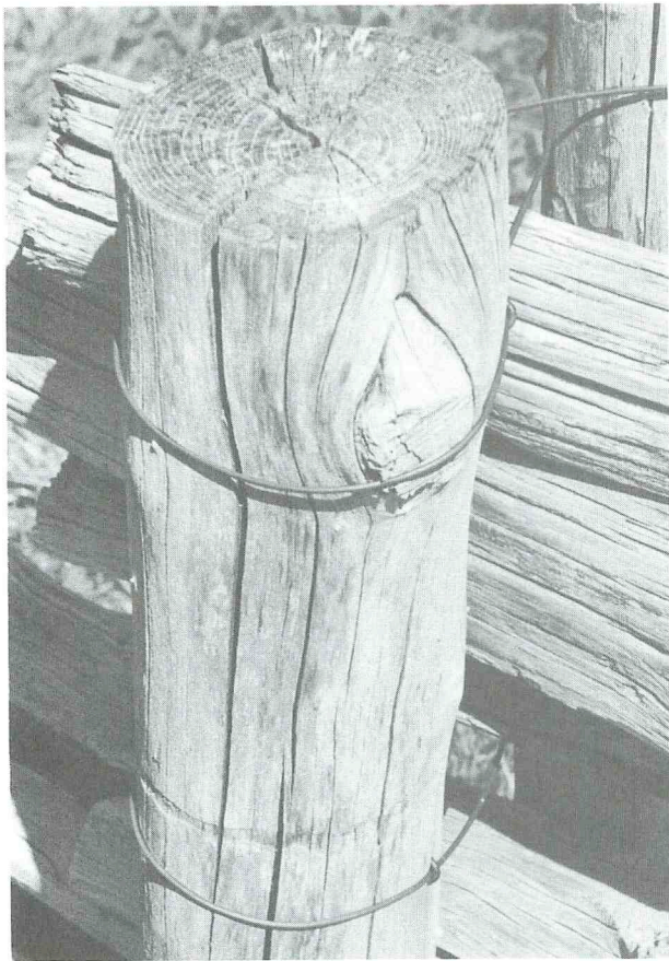
Illus. 60. Aluminum wire holds double posts firmly, forcing the rails to stay in place. Use a figure 8 loop, as shown, for best security. It is not really necessary to use such a loop at every row of rails, as is done here.
