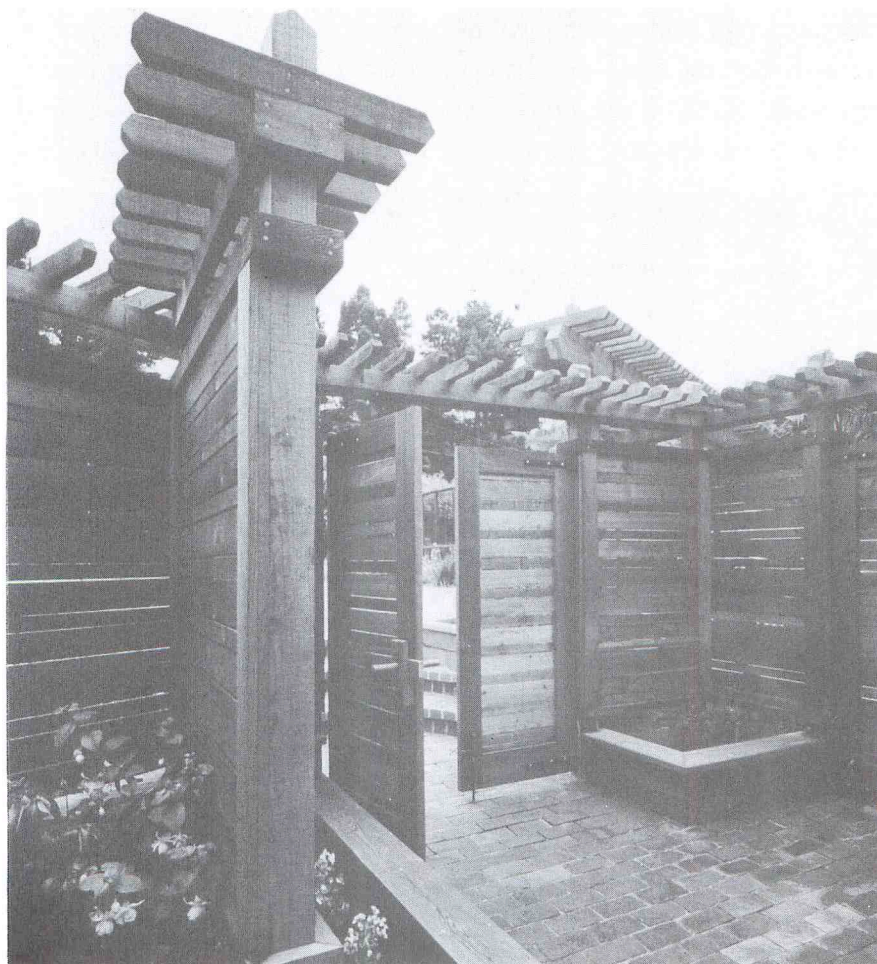
Illus. 5. This decorative fence provides shade, privacy, and wind protection. Built of a less expensive grade of redwood, Construction Heart, this fence is economical and easy to maintain because of its inherent resistance to insects and decay.
