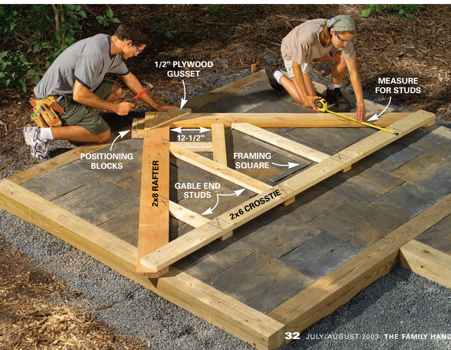
Figure C Rafter Details
