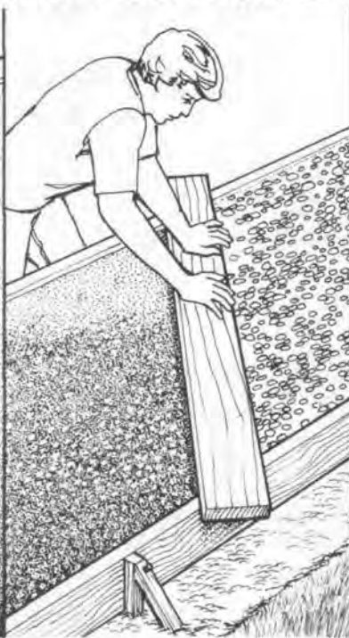
Embed stones flush or \frac{1}{16} " below surface
