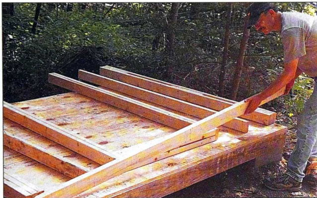
Fig. 7 With the back wall framing members cut to length and headers assembled, lay out the pieces on the shed floor and join them with nails.
