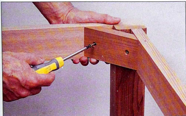
Fig. 19 A corner block is installed at each leg on the table and the benches. A pair of screws holds each block to the aprons.
