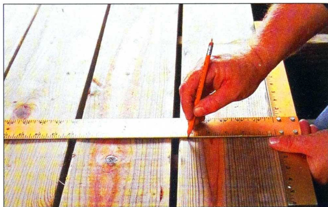
Fig. 11 To keep the screw rows straight, draw a line across the boards above each joist. We used a drywall square to do this.
