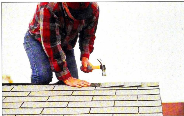
Fig. 14 Cut the shingles into three tab-size pieces and use the tabs to cap the peak. Be sure to space each piece 5 in. apart.
