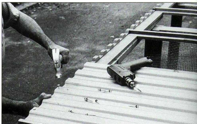
Fig. 20 Prebore the clearance holes in the panel ridges and molding. Attach the panels with aluminum nails that have rubber washers.
