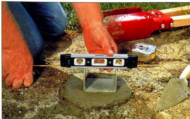
Fig. 2 Level the 4x4 brackets in both directions using a torpedo level, and let the concrete cure for at least a day before building on it.
