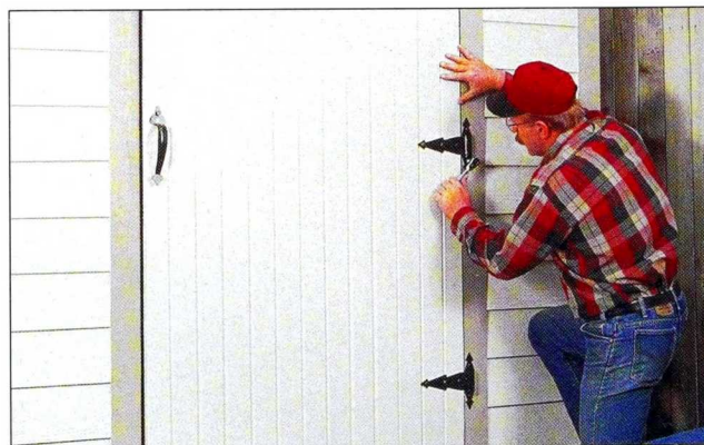
Fig. 16 Hang the door with three steel gate hinges. Secure it to the trim with lagbolts, then add the handle, bolt, and hasp.
