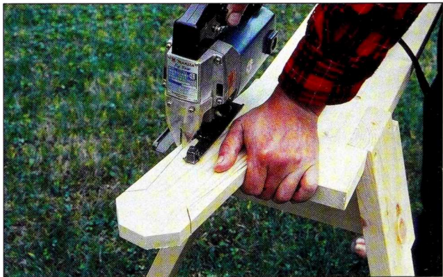
Fig. 2 Finish the rough picket outline by making the longer side cuts on individual pickets with a sabre saw. Cut one picket at a time.
