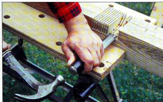
Fig. 8 Cut the 4x4 post notches by making a series of kerfs with a circular saw. Then remove the waste with a sharp chisel.
