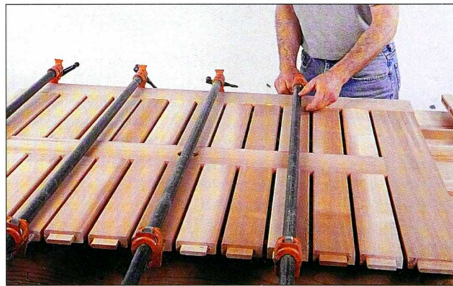
Fig. 18 Clamp one stile at each end of the top subassembly. Space the bar clamps evenly and at the center of each tenon.
