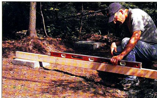
Fig. 3 Use a straight 2x4 and a 4-ft. level to check that the corner blocks are installed at the same height all the way around.
