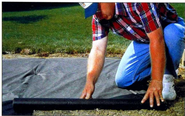
Fig. 3 Remove the sod on the site, then cover the soil beneath the deck with landscape fabric. This keeps weeds from growing.
