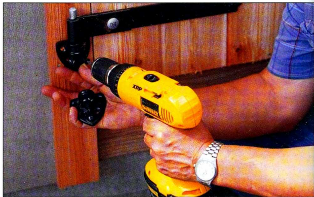
Fig. 14 Use tongue-and-groove cedar to build the doors. Then hang the doors with heavy-duty strap hinges and install the door handles.
