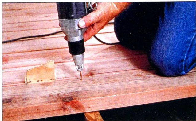
Fig. 9 Use a ¼-in. plywood spacer to maintain consistent gaps between the decking planks. Drive two screws through each board into each joist.
