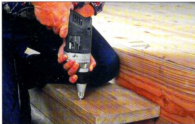
Fig. 15 Complete the step by installing a tread. Use at least three screws on the sides, and several along the front and back.
