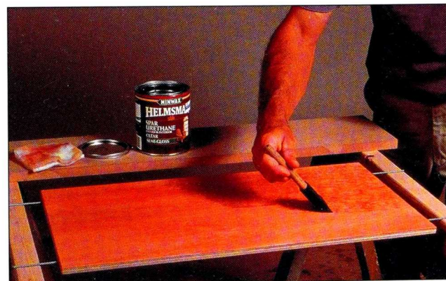
Fig. 2 Suspend the plywood panels between sawhorses. Apply the exterior polyurethane finish on the panels' faces and edges.
