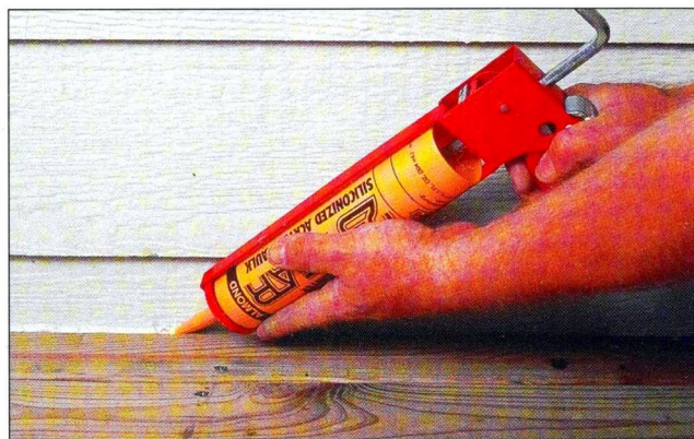
Fig. 16 To protect the siding behind the ledger from water exposure, seal the top joint with a bead of silicone caulk.
