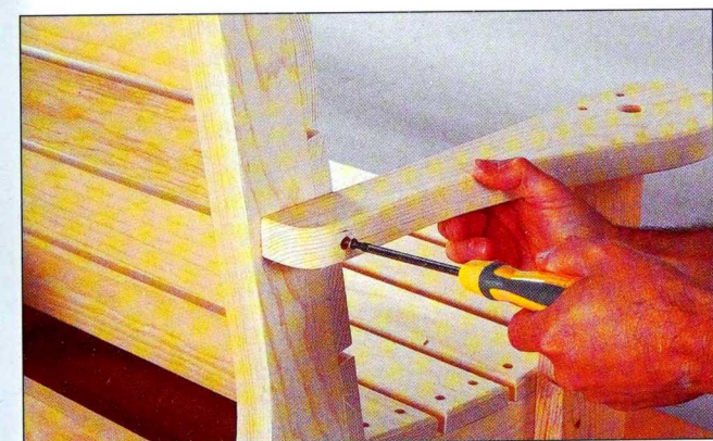
Fig. 14 Bore pilot holes through the edge of each armrest and its top. Fasten it to the armrest support first, then the back support.
