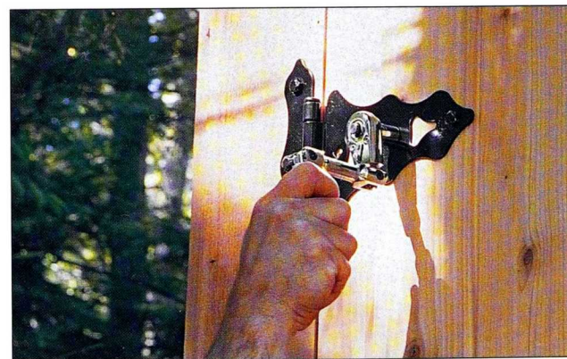
Fig. 17 Position the door in its opening with a \frac{1}{8} -in. space at the top and sides. Bore pilot holes for the hinge screws and secure the hinges.
