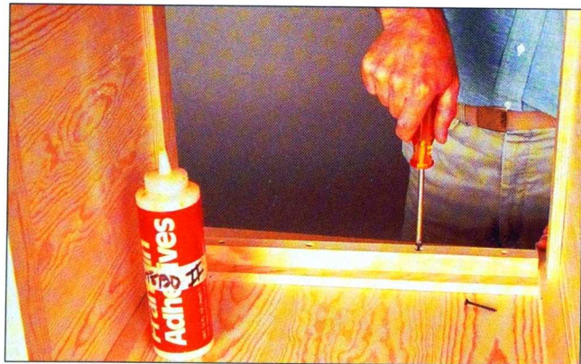
Fig. 8 Install the ledgers to two opposite lower rails with screws and glue. Countersink pilot holes for flathead screws.
