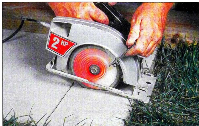
Fig. 1 Begin by laying out the deck location. If concrete must be cut, use a masonry blade in an old circular saw to score the surface.
