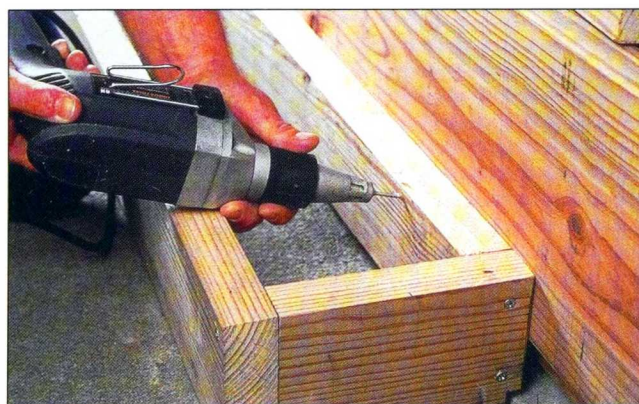
Fig. 14 Make sure the top of the step box is truly parallel to the top of the deck. Then attach it to the deck with screws.
