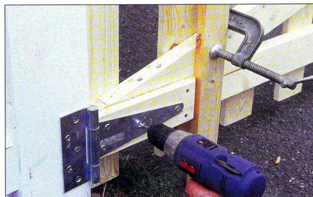
Fig. 10 Clamp support sticks to the gate to help align it with the fence. Use 2-in. screws to secure the hinges to the fence rails.
