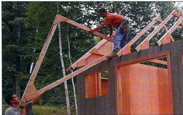
Fig. 10 Carefully slide the roof trusses onto the walls. Space them precisely 24 in. on center and secure them with 3-in. screws.
