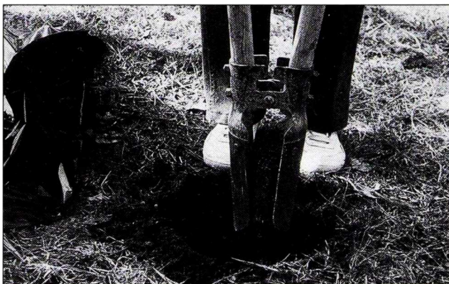
Fig. 1 Dig the fence post holes to about 30 in. deep with a post hole digger. This hand tool is available from most rental equipment dealers.
