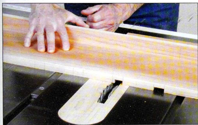
Fig. 1 After cutting the 1x8 lattice stock to length, lay out the half-lap joint notches and cut them with a dado blade in the table saw.
