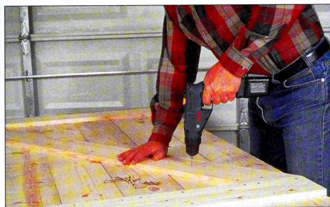
Fig. 15 Build the door by using tongue-and-groove pine. Attach the crossmembers and a diagonal brace with screws.
