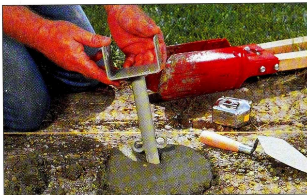
Fig. 1 After pouring concrete into each footing hole, set a metal 4x4 bracket into the wet concrete. Align the brackets with the string line.
