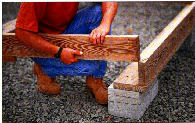
Fig. 2 Set the 2x6 floor joists on top of the 2x8 mudsills. These floor-frame members are cut from pressure-treated lumber.
