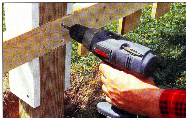
Fig. 9 With the posts resting in their holes, install the picket/rail assemblies. Screw the bottom rails to the 4x4 posts, then plumb and align the fence.
