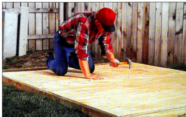
Fig. 2 Nail ½-in. tongue-and-groove plywood to the floor frame. After this is completed, coat the floor with an enamel porch paint.
