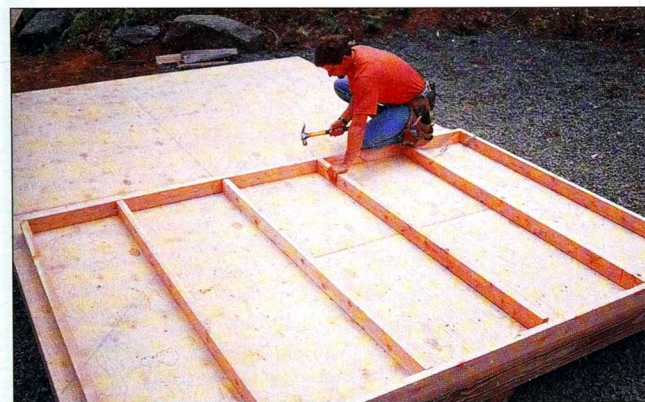
Fig. 6 Build the exterior walls on the floor. Assemble the 2x4s with 16d nails and then add the plywood sheathing.
