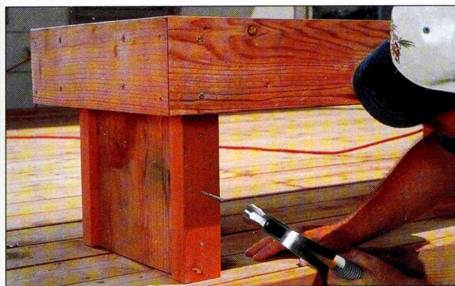
Fig. 16 Finish the legs with 2x3 vertical trim pieces. These pieces hide the leg screws and give the benches a more substantial feel.
