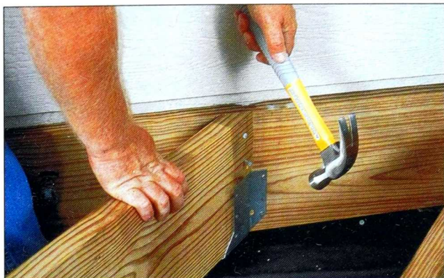
Fig. 7 Use 45° joist hangers to attach the joists to the angled ledger. Nail the top half of the joist directly into the ledger for stability.
