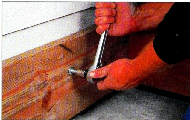
Fig. 5 Slide a lagbolt and washer into each ledger hole and tap the bolt with a hammer. Then drive it into the rim joist with a wrench.
