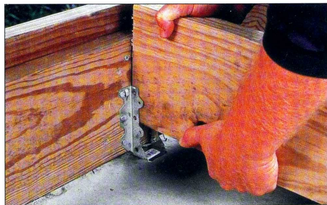
Fig. 9 Lay out the outside rim joist for the deck joists and install a joist hanger at each mark. Slide the joists into place.
