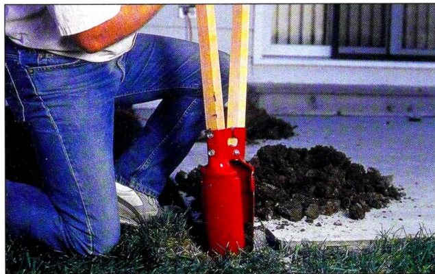
Fig. 2 Use a post-hole digger to dig pier footing holes below the frost line. Square off the bottoms of the holes in preparation for the posts.
