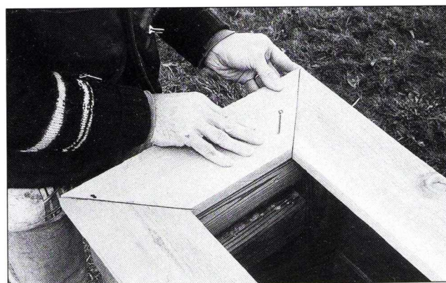
Fig. 17 Finish the top of the walls with \frac{3}{4} x 4 \frac{3}{4} -in.-wide rough-sawn cedar. Fasten the cedar trim with 6d galvanized finishing nails.
