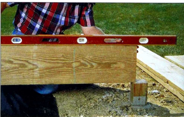
Fig. 5 Use a straight joist to level between the ledger and the support posts. Mark and cut the posts, then check the level again.
