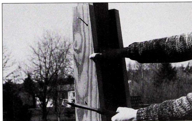
Fig. 1 After the posts are set in their holes, plumb and brace them in place. Then begin the benches by nailing the back braces to the post sides.
