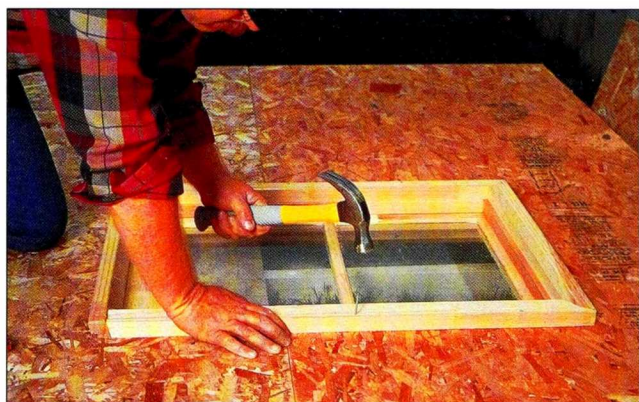
Fig. 4 After sheathing the wall, cut the window opening and use 10d galvanized casing nails to secure the window to the wall.
