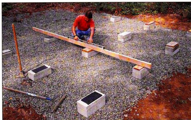
Fig. 1 Use a 4-ft. level and a long, straight 2x4 to ensure that the concrete foundation blocks are level. Add shims to build up any low blocks.
