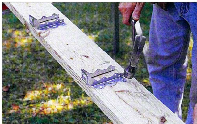
Fig. 4 After marking the joist locations on the long front and rear rim joists, install metal hangers with 1½-in. joist hanger nails.
