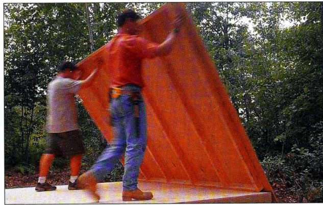
Fig. 7 Carefully raise the end wall into position. Note how the plywood siding hangs down to cover the floor framing.
