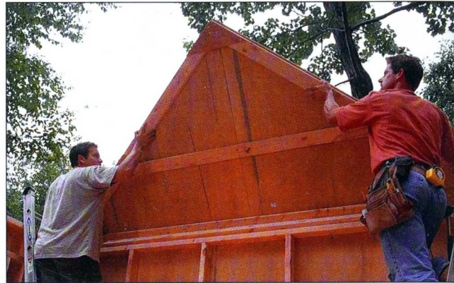
Fig. 9 Start the roof by installing the end trusses. The plywood siding is nailed on before the truss is raised. A central 2x4 chord stiffens the sheathing.
