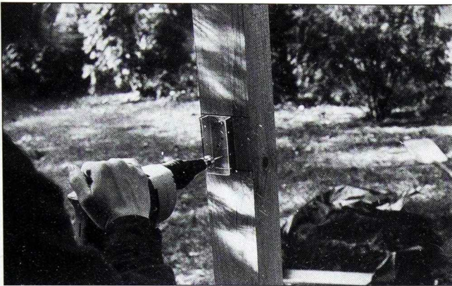
Fig. 5 Mount the brackets to the posts with 1 \frac{1}{4} -in. galvanized screws. An electric screw gun provides a no-sweat way to drive screws.
