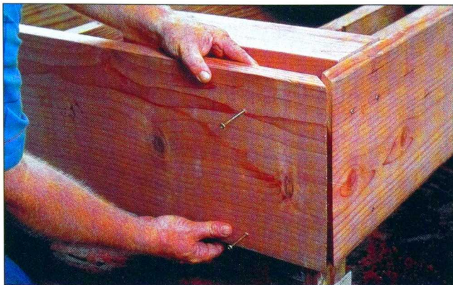
Fig. 10 Trim the perimeter of the deck with 2x12 redwood boards. Screw these boards into the rim joists and also into the deck planks.
