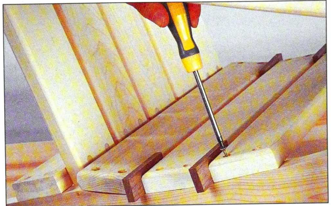
Fig. 18 Fasten the seat slats with screws. Again, note the use of \frac{3}{8} -in.-thick blocks to ensure uniform spacing between slats.
