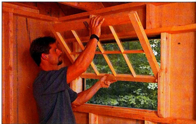
Fig. 15 Slip the barn-sash window into the window frame and set it down on the sill. A simple barrel bolt holds it closed.
