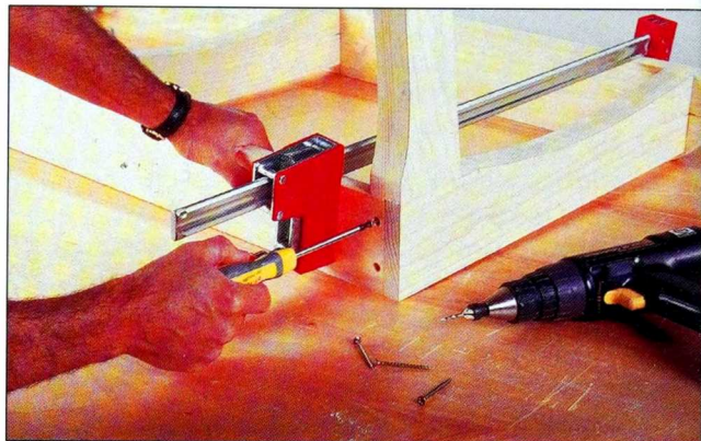
Fig. 9 Clamp the rear rail to the seat supports, and bore pilot holes into each support. Fasten the rail with galvanized screws.
