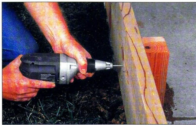
Fig. 7 After setting the 4x4 posts, plumb them in place. Then screw the rim joists to them with three or four long screws.
