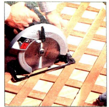
Figure 5: Support lattice panels with scrap plywood for cutting. A carbide blade will cut through the staples without dulling.
