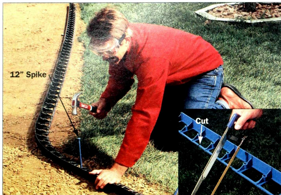
Figure 6: Install the edging on the tamped subbase using 12-inch spikes. Inset: Cut the webbing on the edging's back side to make it flex for curves.
