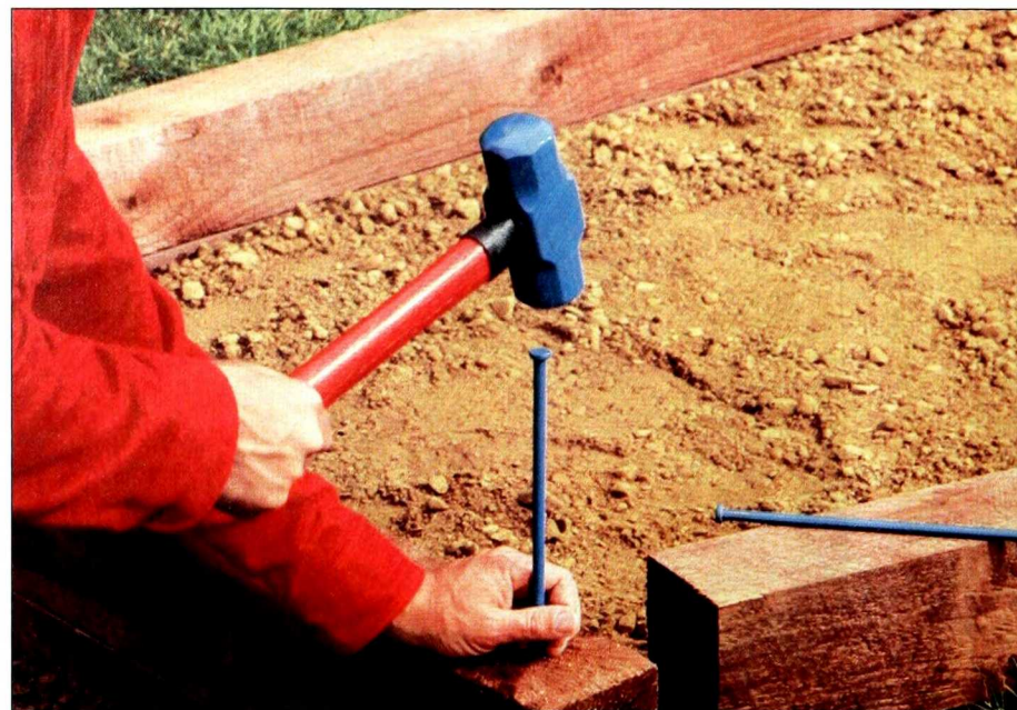
Figure 7: Install landscape timbers for edging in areas where you need to change levels or step down. Be certain to overlap corners.
