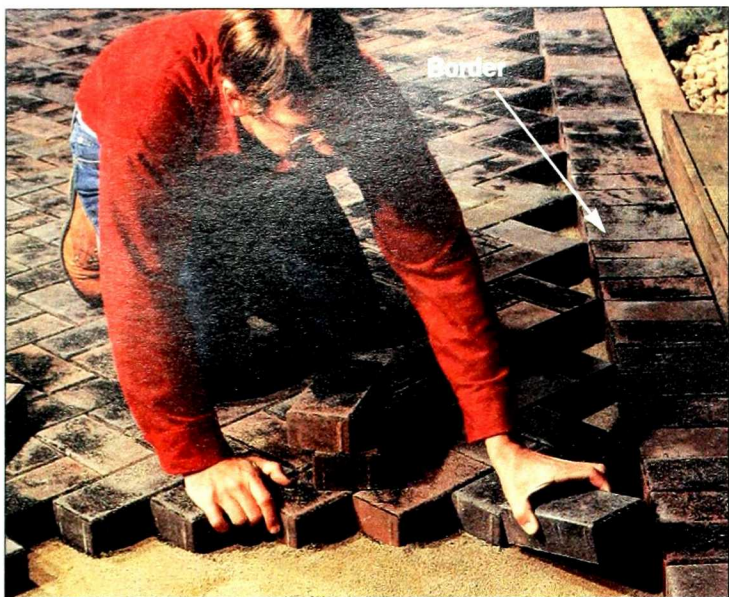
Figure 9: Install the pavers starting along the longest, straightest edge. Border pavers provide a crisp finished edge, especially along curved portions of the patio.
