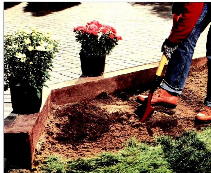
Figure 16: Landscape around the completed patio with flowers, shrubs, and grass. Grass will root through the open spaces in flexible edging and help anchor the edging in place.
