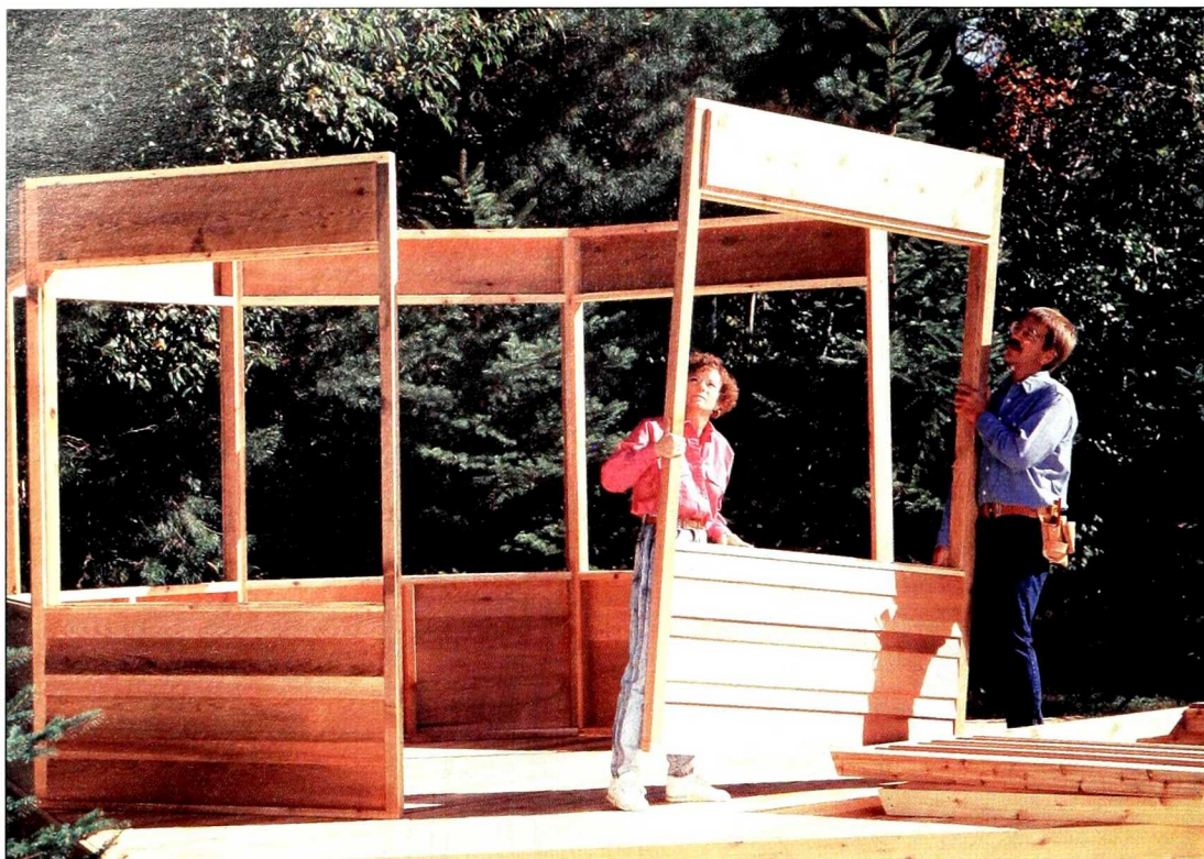
Figure 9: Set up wall sections, fastening them to the deck and to each other. A 14-foot-diameter circle acts as a guide for the corners.
