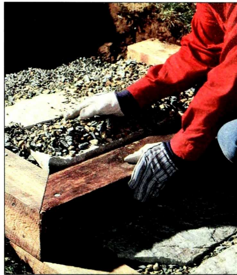
Figure 12: Fill the gaps between the treads and the timbers with another layer of fill rock; \frac{3}{4} -inch rock is easiest to spread and comfortable to walk on.
