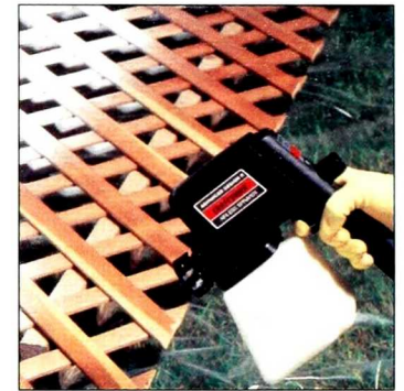
Figure 6: Paint lattice panels with a paint sprayer. You can paint on the ground or paint the whole arbor after completion.
