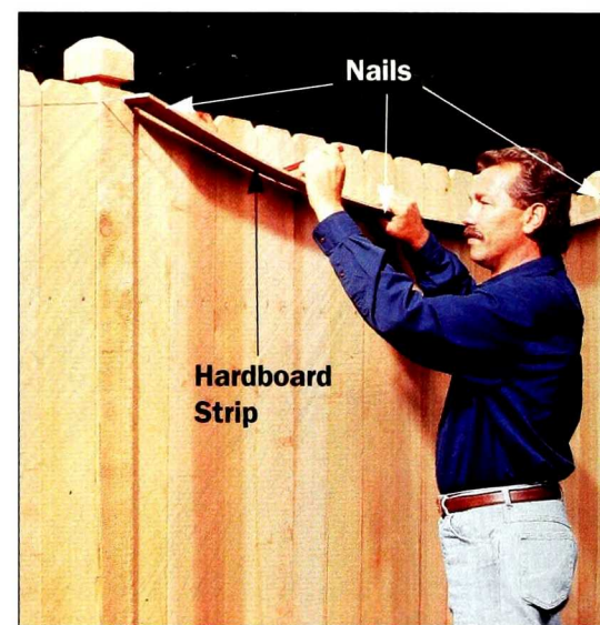
Figure 12: Trace the curve for the top of the fence boards using a thin strip of 1/4-inch hardboard bent between three nails.
