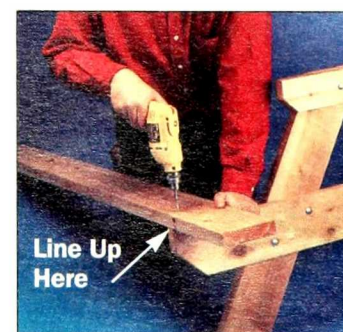
Figure 3: Start with the outer seats when assembling the table, lining them up flush with the ends of their supports. Then add the other boards, spacing them evenly.
