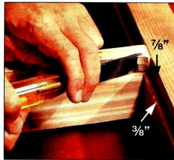
Figure 5: Square the corners of the rabbet using a sharp chisel. Then check the edges of the wall for square.
