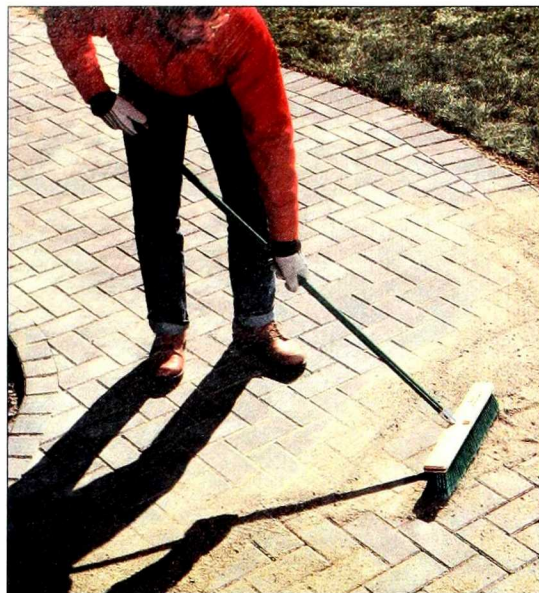
Figure 15: Sweep coarse, dry sand between the cracks of the pavers to lock them together and fill voids. Repeat with more dry sand in a few days.
