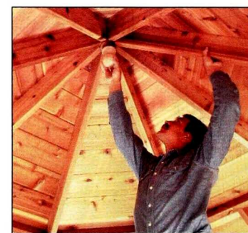
Figure 22: Screw a finial to the hub and you're done.
