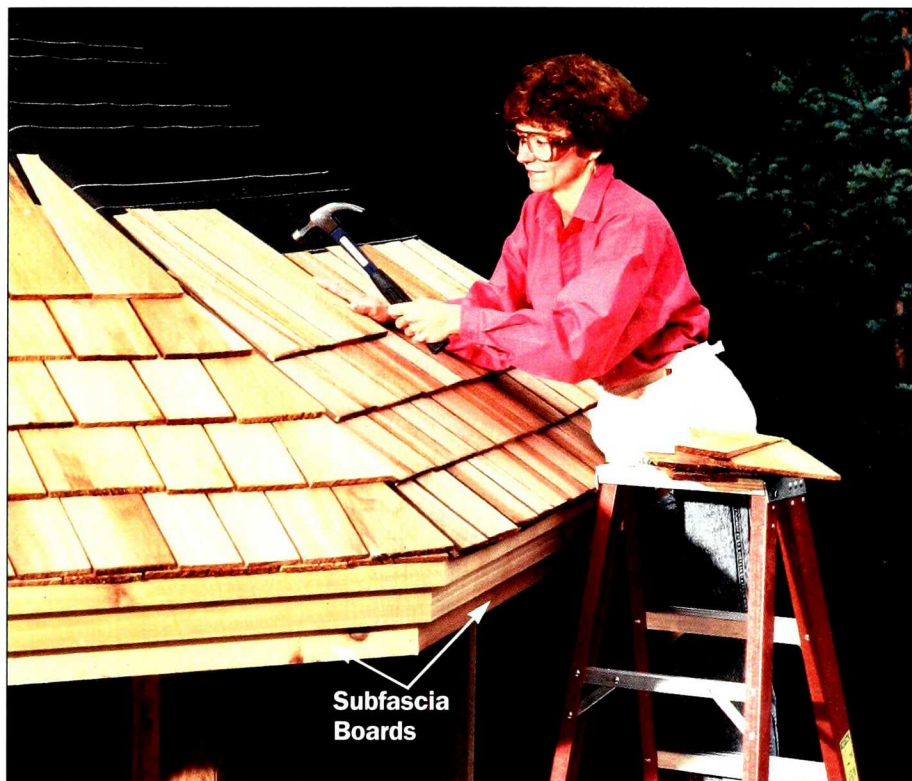
Figure 16: Lay cedar shingles over the tarpaper. Use 1 inch nails to attach the shingles so the points won't come through on the inside of the gazebo.
