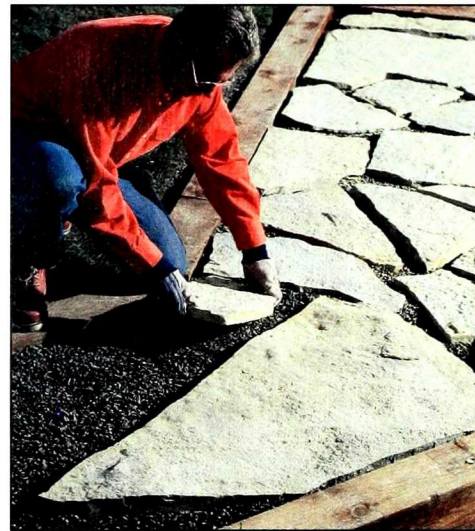
Figure 15: Place the flagstones on the fill rock. Don't be afraid to move them around or to use large pieces. Have some fun with the pattern, but try not to leave more than 2 to 4 inches between pieces.
