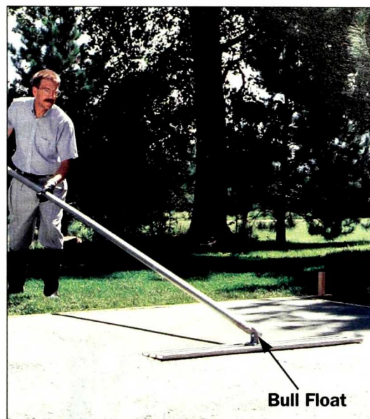
Figure 4: Float the concrete to even out high and low spots and further smooth the surface. Remove small ridges that may remain with a hand trowel.
