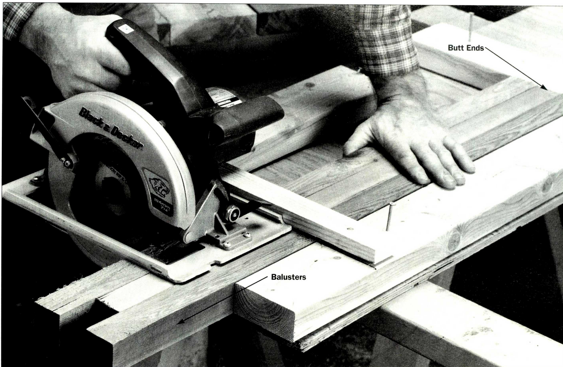
Figure 3: Slip lengths of baluster stock under the guide, hold them tightly against the 2x4 stops, and cut them off. To prevent excess splintering and to save time, cut
