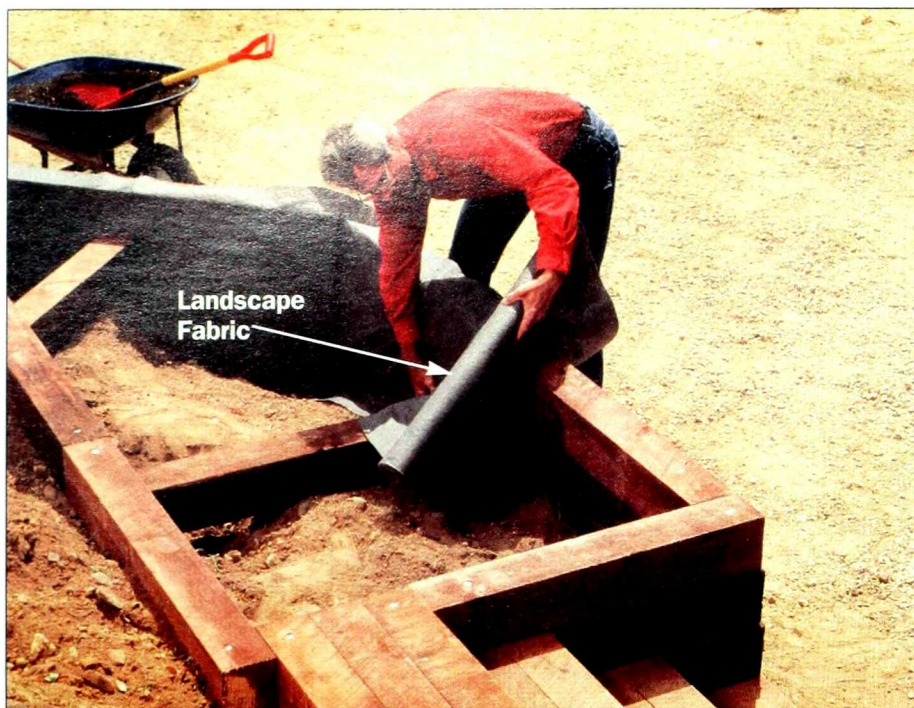
Figure 12: Install landscape fabric on the back side of the retaining wall to prevent soil from washing through cracks and gaps.
