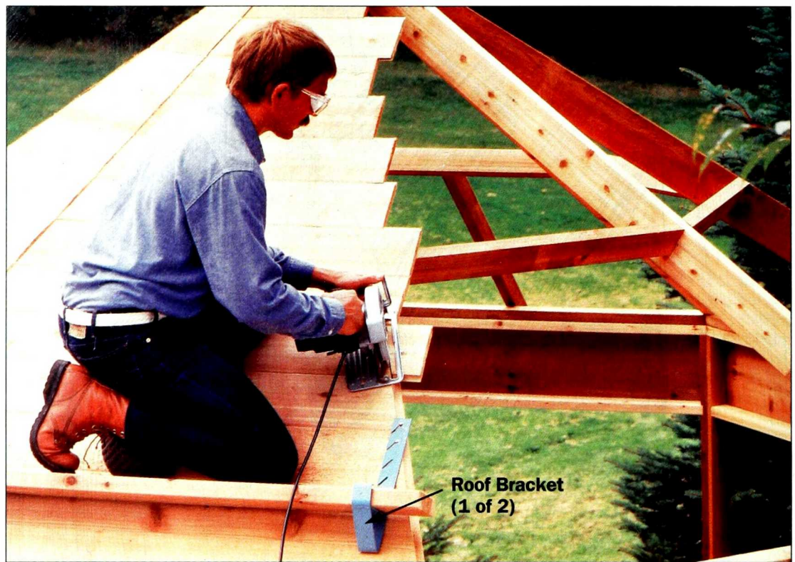
Figure 15: Install roof decking one section at a time. Let the boards run long at one end, then trim them after nailing. Note the roof brackets used for comfort and safety.
