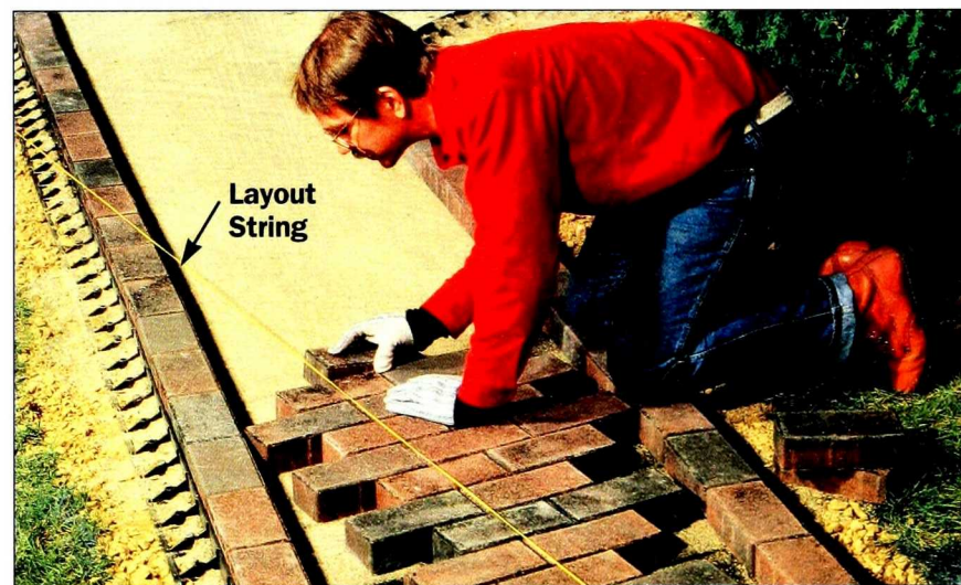
Figure C: Lay the pavers using a string for a guideline. Cut and install pieces that butt up to the border later.
