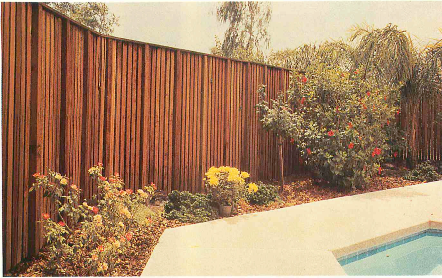
Illus. B1. This redwood fence separates pool and entry court. Rugged, knot-textured redwood Garden grades have natural beauty and outstanding weatherability.
