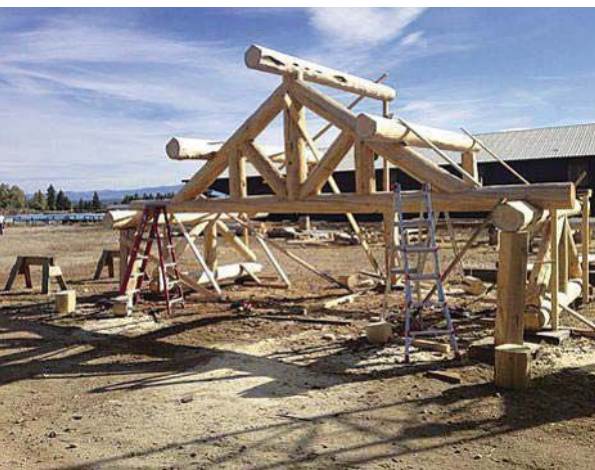
The Murphys' log package is pre-assembled in BVL's log yard before shipping.
