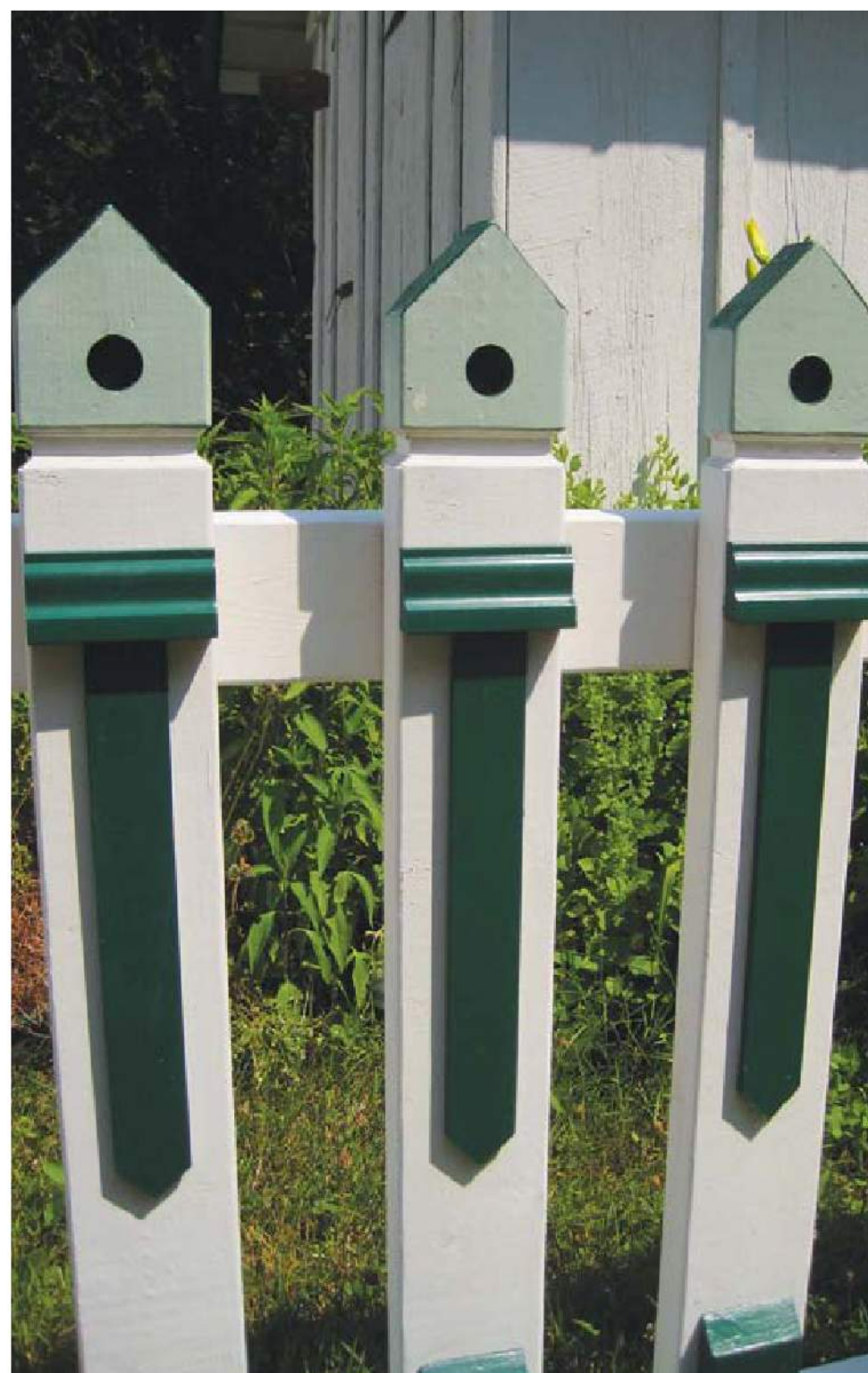
The collar and necktie appliqués on this picket fence are made from cellular PVC that has been painted with house paint. Cellular PVC holds paint well with a bit of sanding to roughen the surface.
