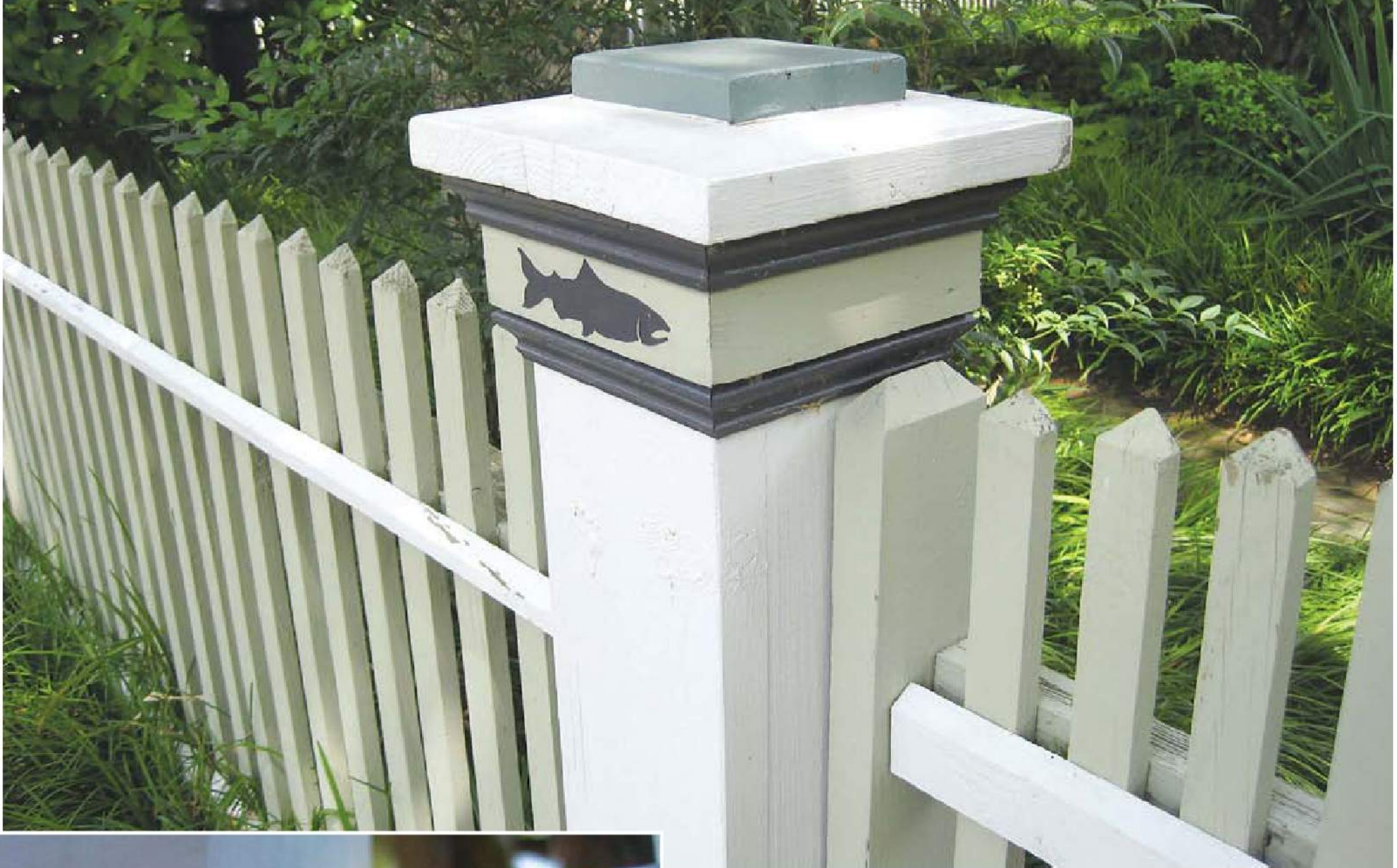
Above: A stile to support the infill is fastened to the post with nails.
