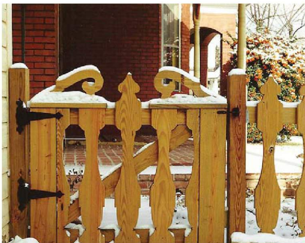
This fence was made using decking lumber for the pickets. Full-sized patterns for the picket and gate scroll are included in the Patterns chapter.
