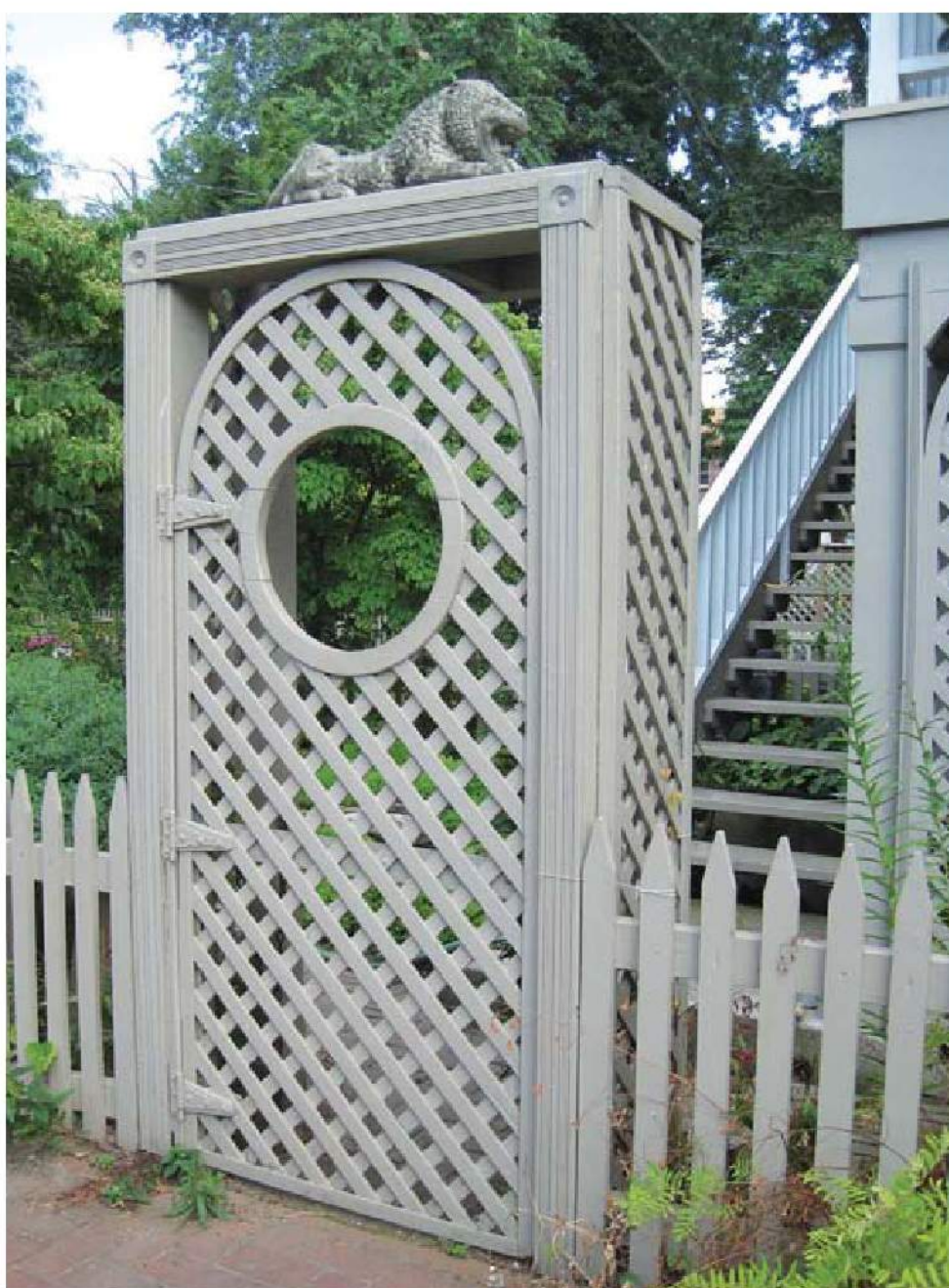
Above: Diagonal infill can be used for support and decoration. Right: Blocking between the pickets and sturdy hinges held on with bolts rather than screws keep this gate in good form without the use of diagonal bracing.
