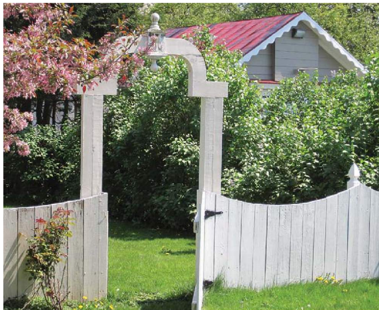
Gates, especially large and heavy ones, can cause the holding post to start leaning. Bracing the post at the top prevents this. Braces can be utilitarian bars or decorative arches.
