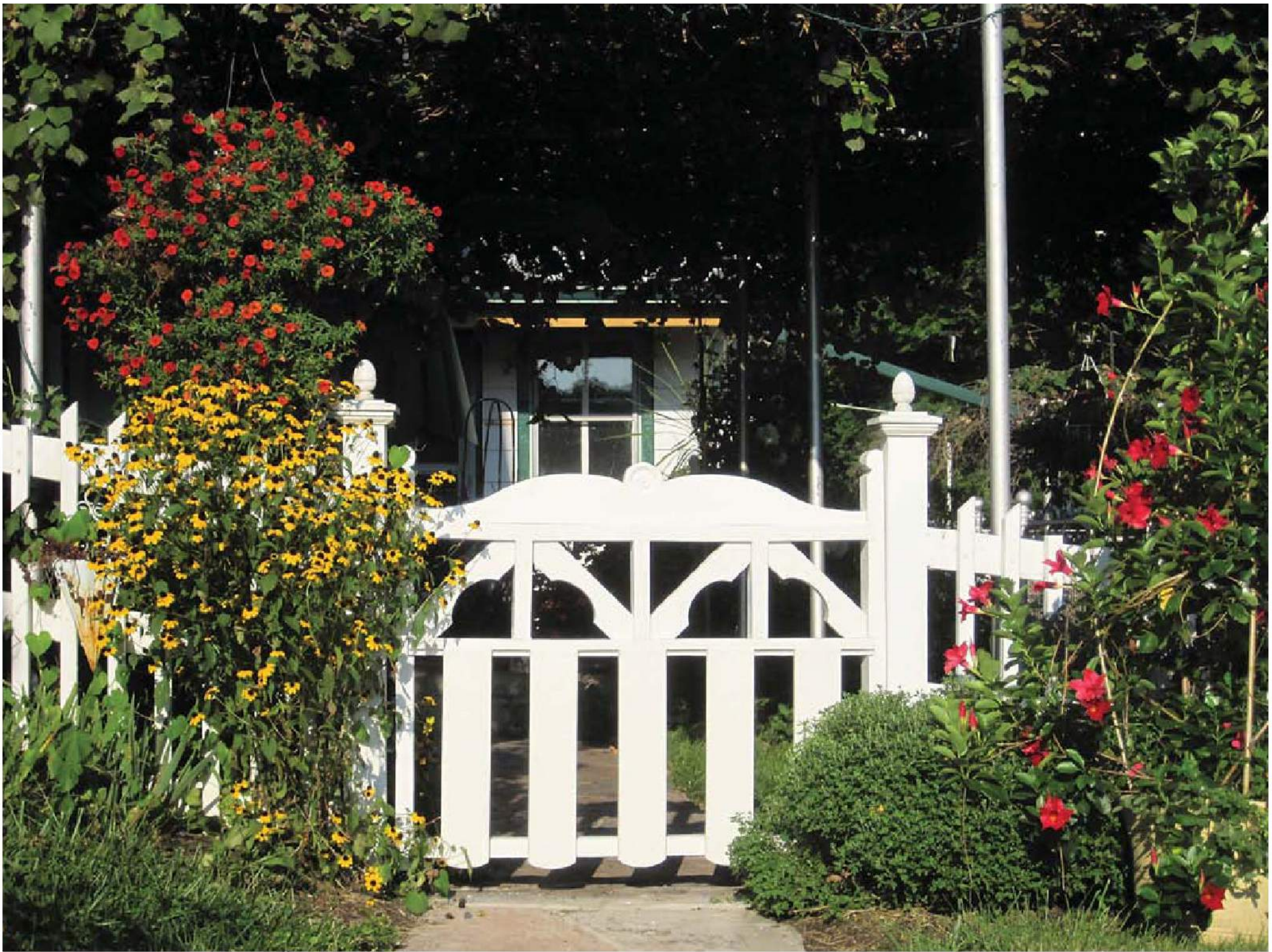
Here is the completed gate. Its decorative braces and broad pickets contrast beautifully against the slender pales of the picket fence.
