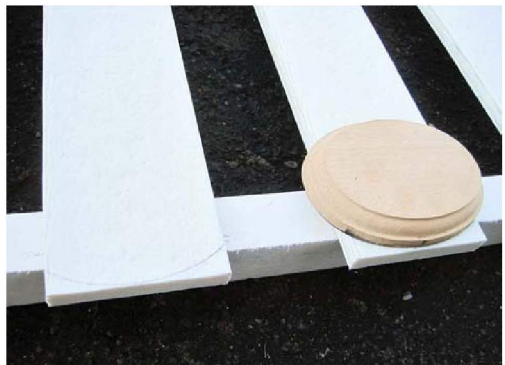
Cut five pickets from 1 x 4 stock to 18 inches in length. Make a decorative scallop on the bottom of the pickets using an object that has a pattern that you like.
