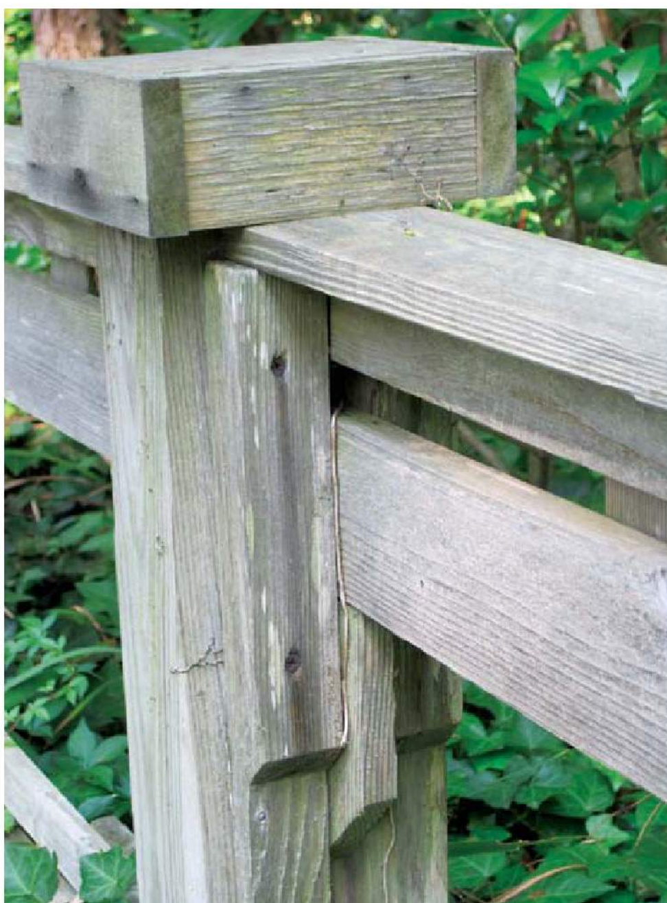
Above top: Cleats are used to support the weight of the rails. Above bottom: Attachment with cleats.
