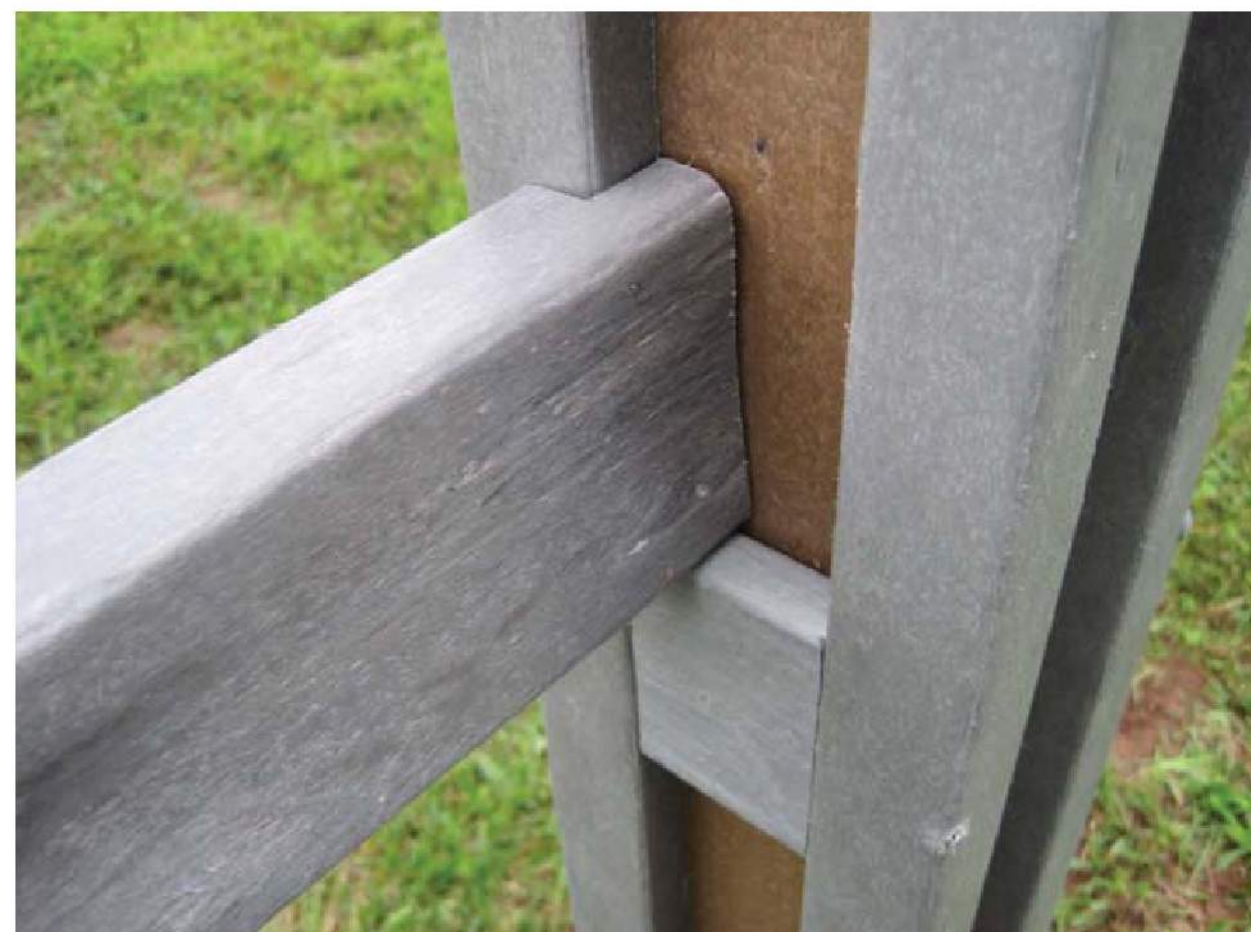
Above: Post belts support the rail and are also decorative. Right: This stringer has had a rabbet joint cut on the end so that it securely fastens to the post corner stile and rests on the post's panel rail.
