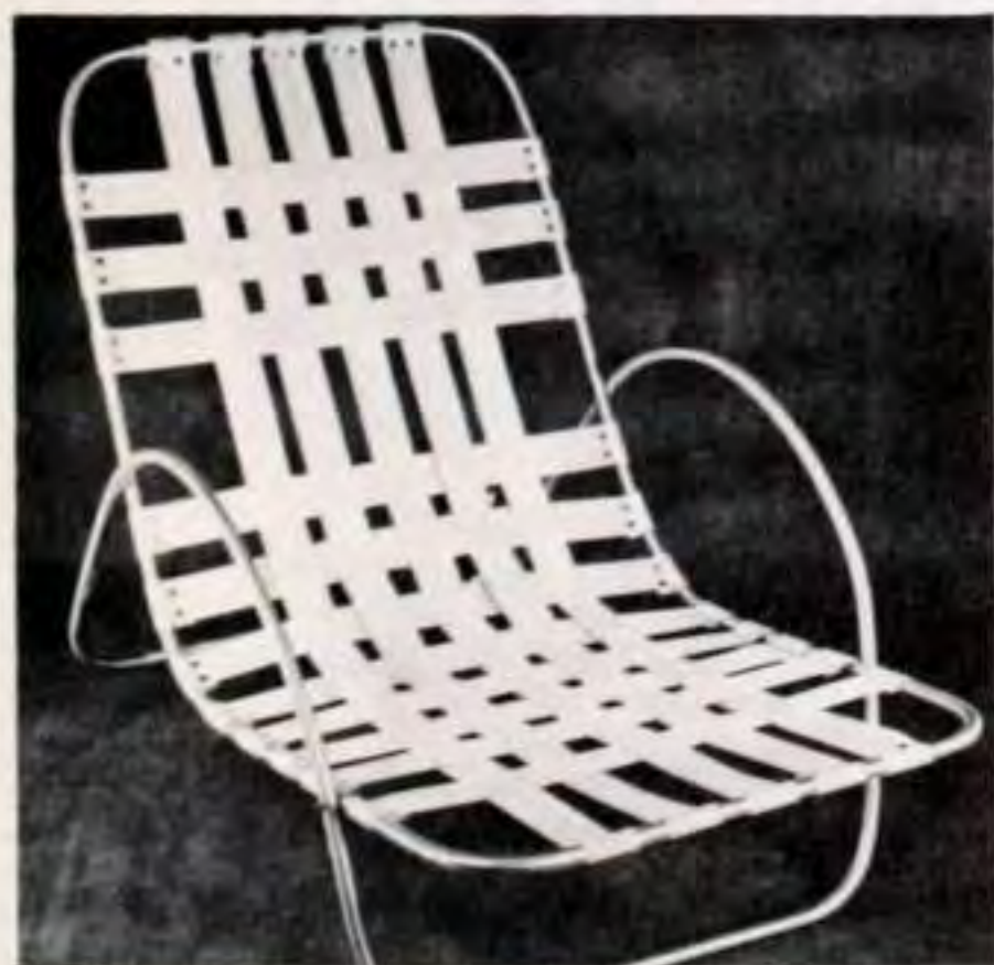
Lace with webbing to support cushions. Rivet webbing loops around the frame
