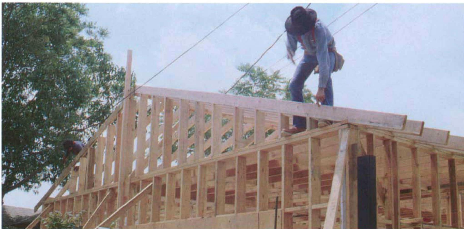
Be sure to nail the gable-end studs in plumb, trusting your eye or using a level. (Photo by Robert Wedemeyer.)
