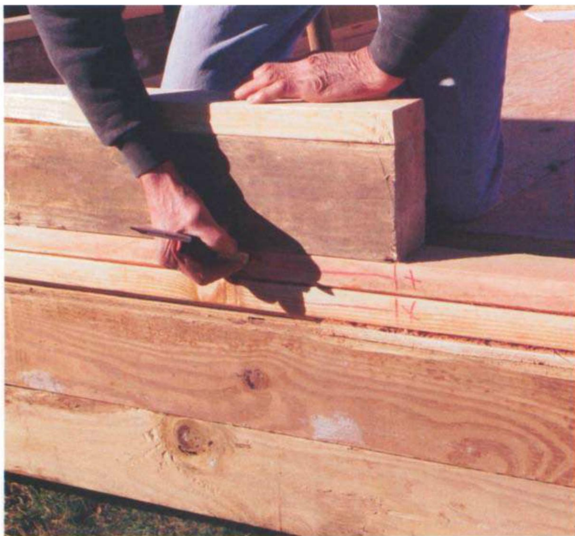
Position each header on the plates and mark down from the header ends across both plates. Mark an X on both plates to indicate the location of the king stud. On the other side of the X, mark a long, straight line to indicate that there will be an opening for a door or window. (Photo by Roe A. Osborn.)
