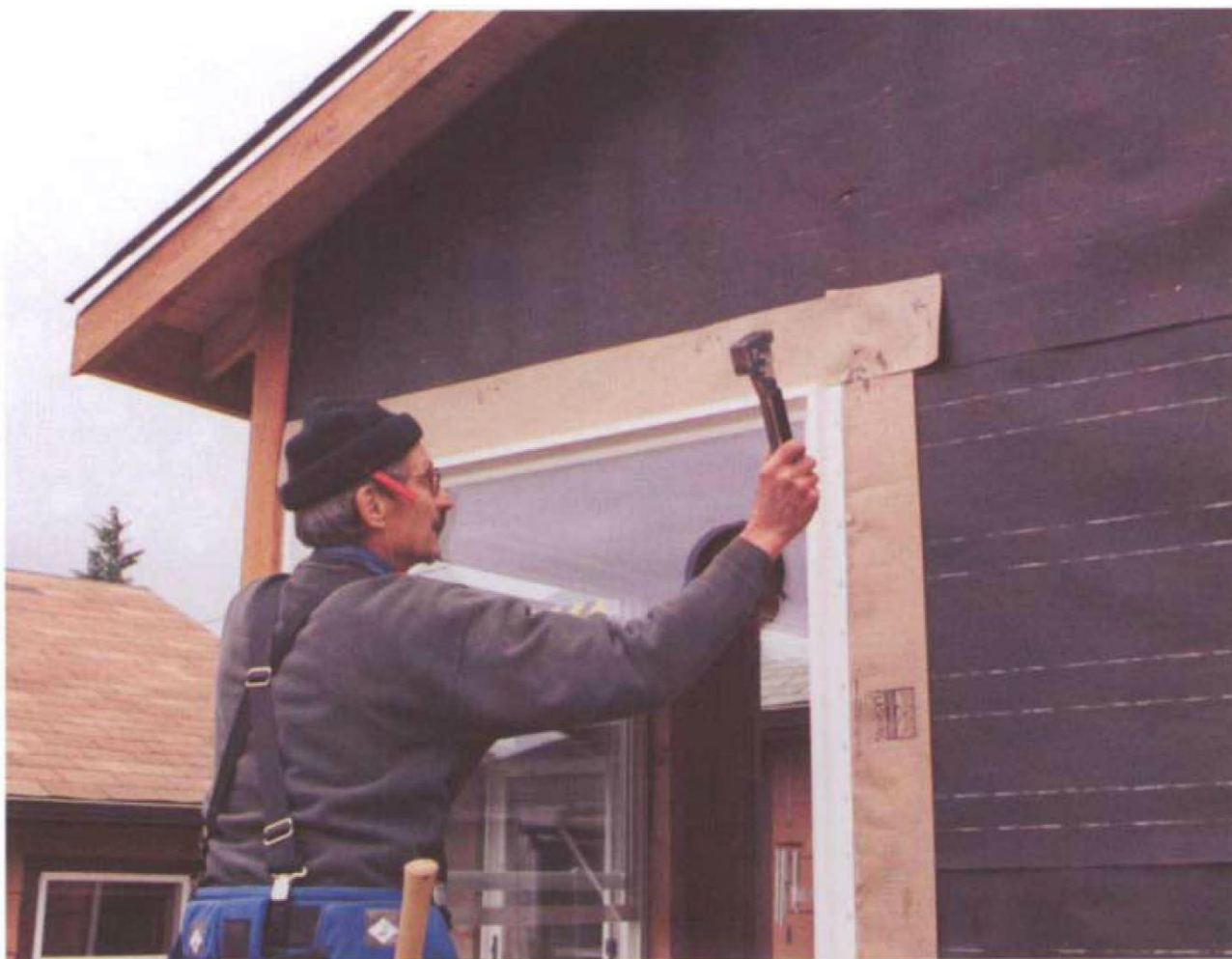
After nailing the window in place, run another bead of caulk at the top of the flange, then staple the last strip of felt paper. (Photo by Roe A. Osborn.)
