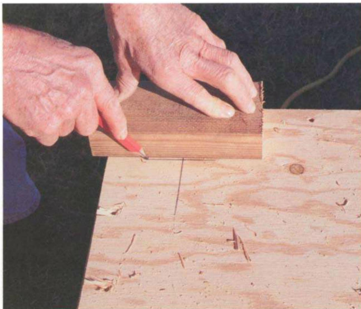
To lay out the wall locations at a corner, place a 2x4 or 2x6 block flush with the outside of the building and mark on the inside with a pencil. (Photo by Roe A. Osborn.)
