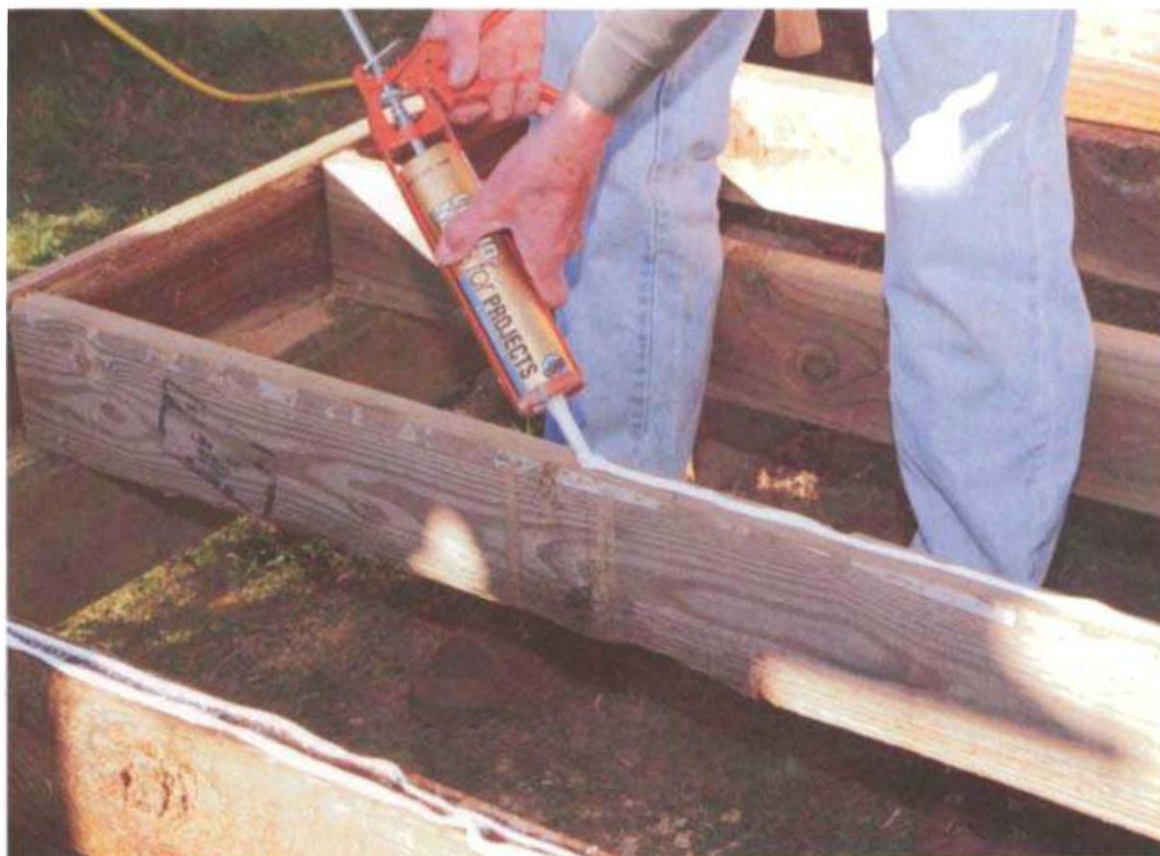
Construction adhesive helps secure sheathing tight to the joists and reduce floor squeaks. Place a \frac{1}{4} -in. bead on each joist. (Photo by Roe A. Osborn.)
