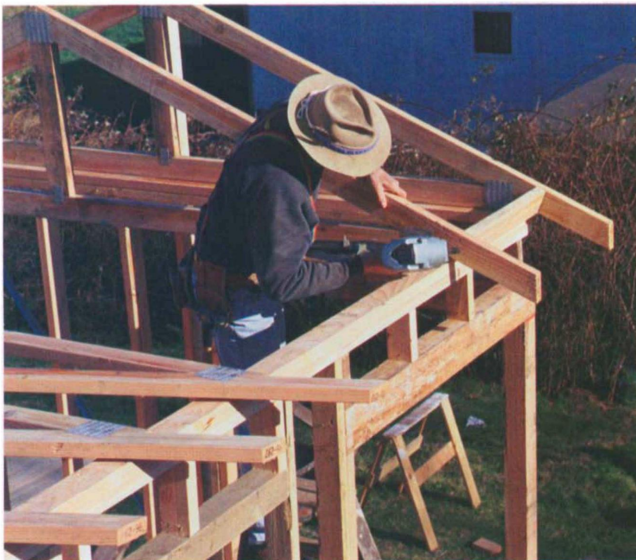
Toenail the joist chord to the top plate with two 16d nails, then drive two more through the rafter chord into the frieze block. (Photo by Roe A. Osborn.)
