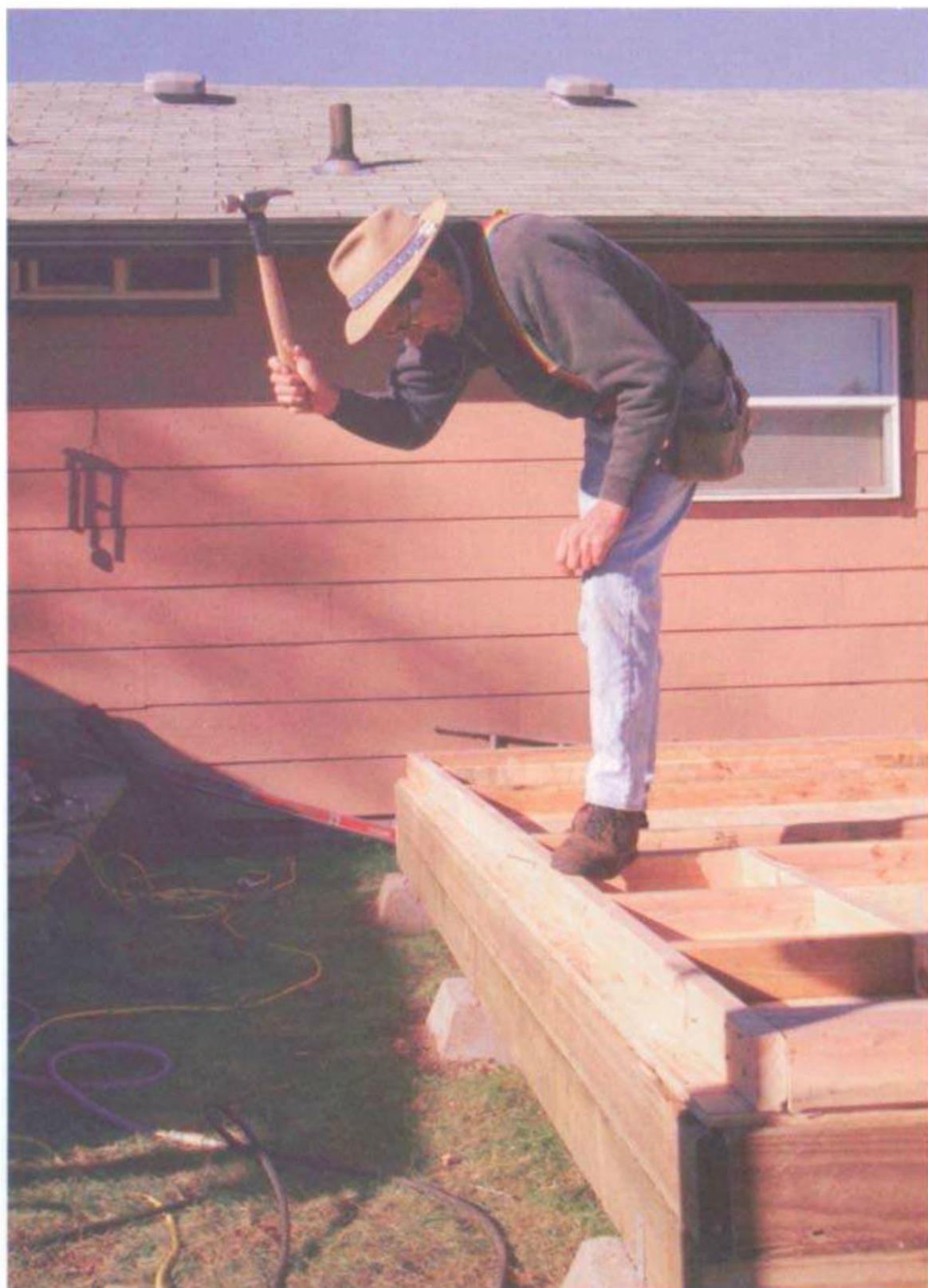
Begin nailing in studs at an outside corner, working either left to right or right to left, whichever feels the most natural to you. (Photo by Roe A. Osborn.)
