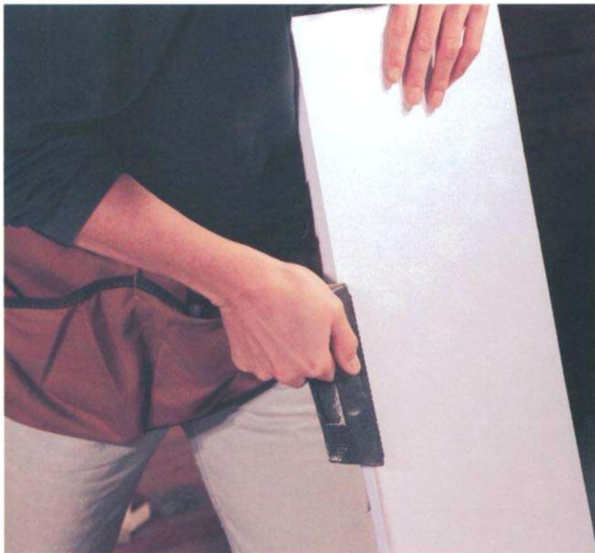
The Surform works well to trim a piece of drywall that doesn't quite fit.
