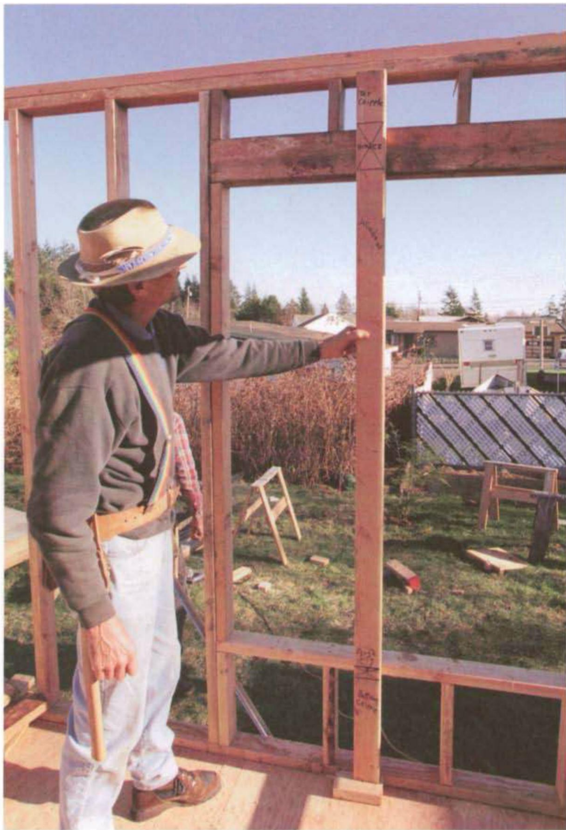
A story pole shows locations of headers and sills and the lengths of cripples and trimmers. (Photo by Roe A. Osborn.)
