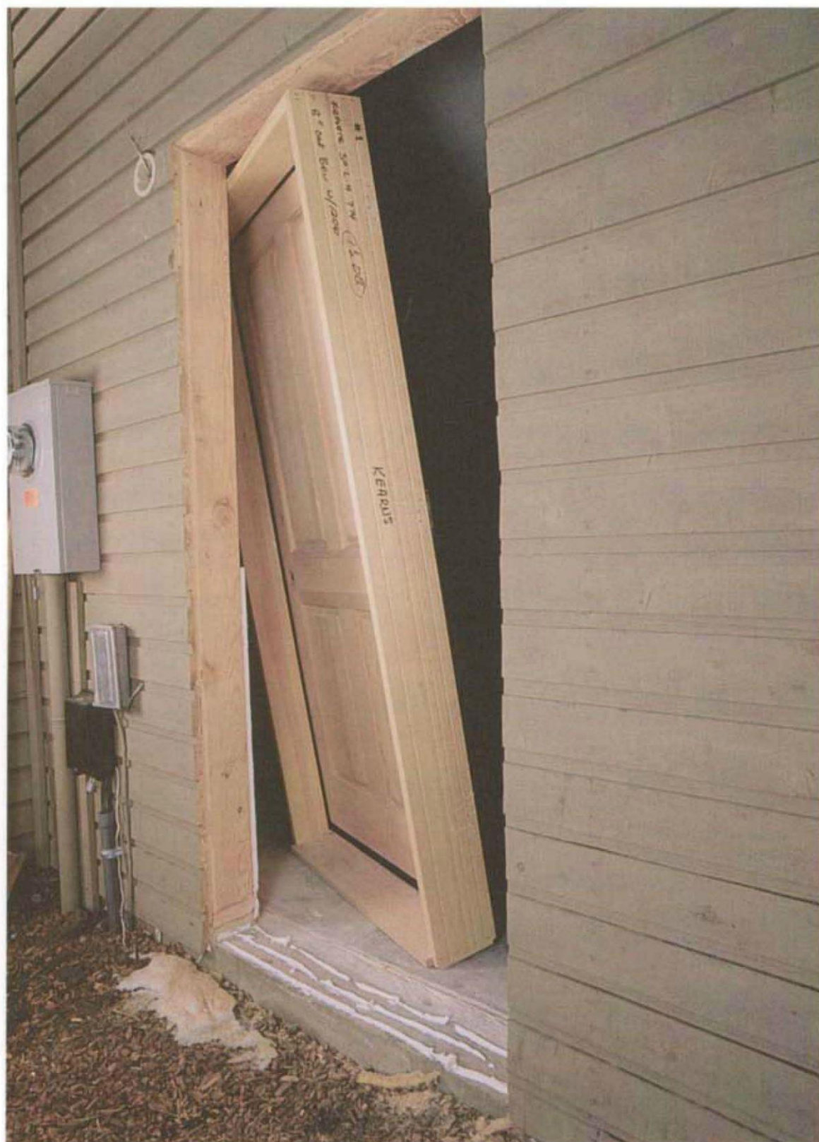
Part of the job of installing a prehung door is to lay a good-sized bead of silicone caulk under the door sill and around the opening under the factory-applied trim. (Photo by Charles Miller.)
