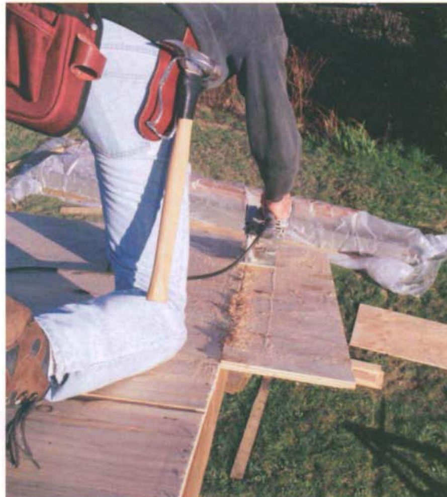
A last step in the roof-sheathing process is to trim the sheathing flush with the barge rafters at the gable ends. (Photo by Roe A. Osborn.)
