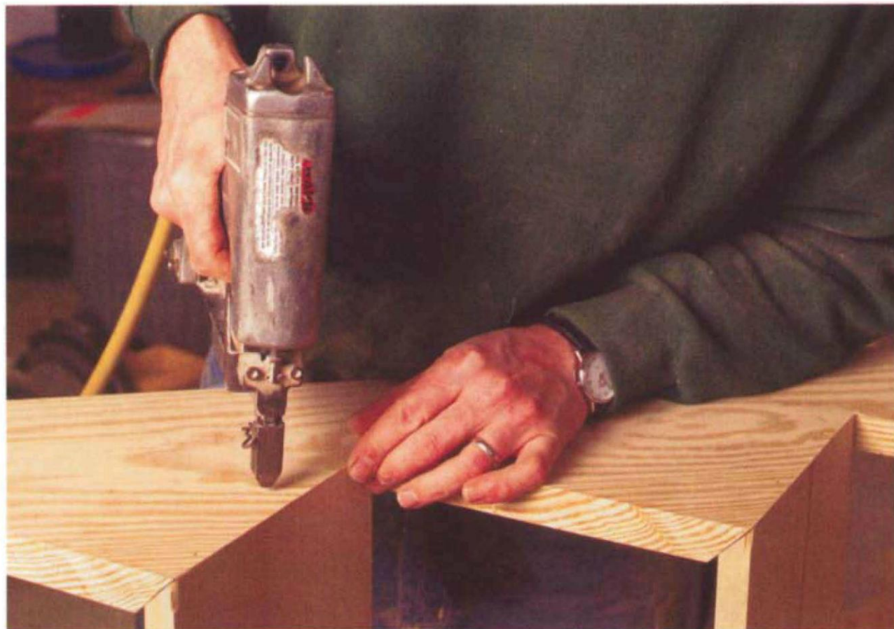
Before nailing on the treads, first nail on the risers, driving two 8d nails through the stringer into each riser board. (Photo by Scott Phillips.)
