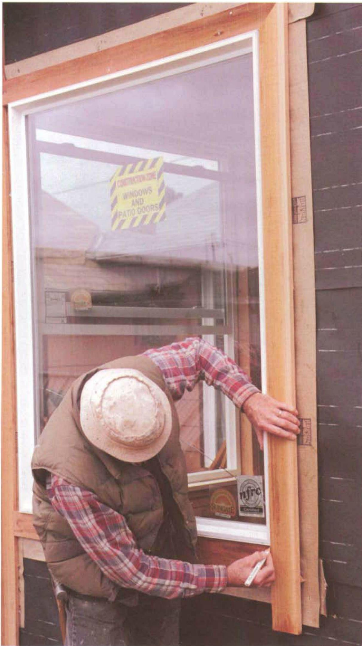
After fitting the miter joint at the top, scribe the miter on the bottom. Mark the miter cut at the window corner and make the cut. (Photo by Roe A. Osborn.)
