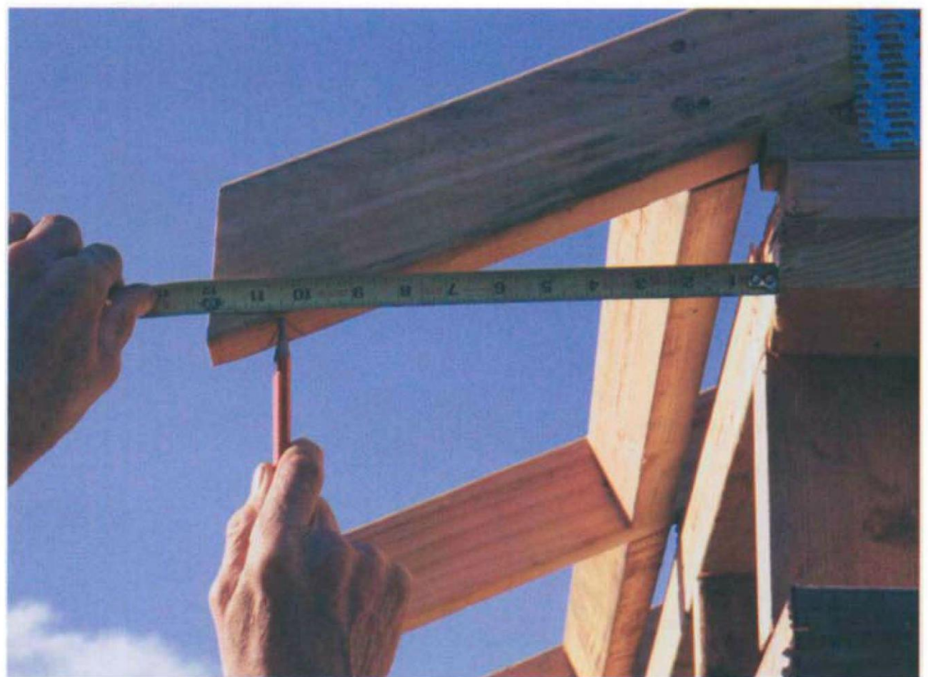
Measure straight out from the building on the gable-end rafters 10½ in. and make a mark. This will be the cut line. (Photo by Roe A. Osborn.)
