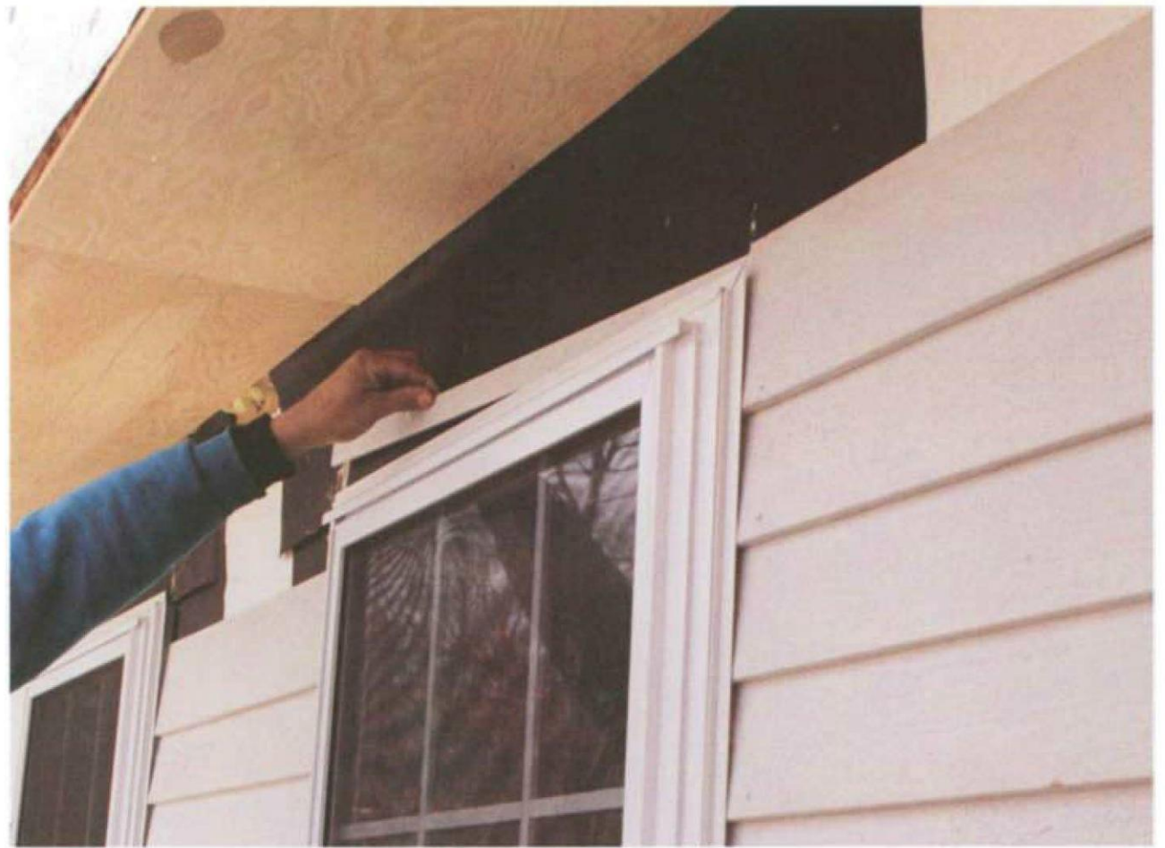
Above openings, install a filler strip to prevent the next course of siding from tipping inward when nailed. It's also a good idea to caulk the tops and sides of window and door openings before nailing on the siding. (Photo by Andrew Engel.)
