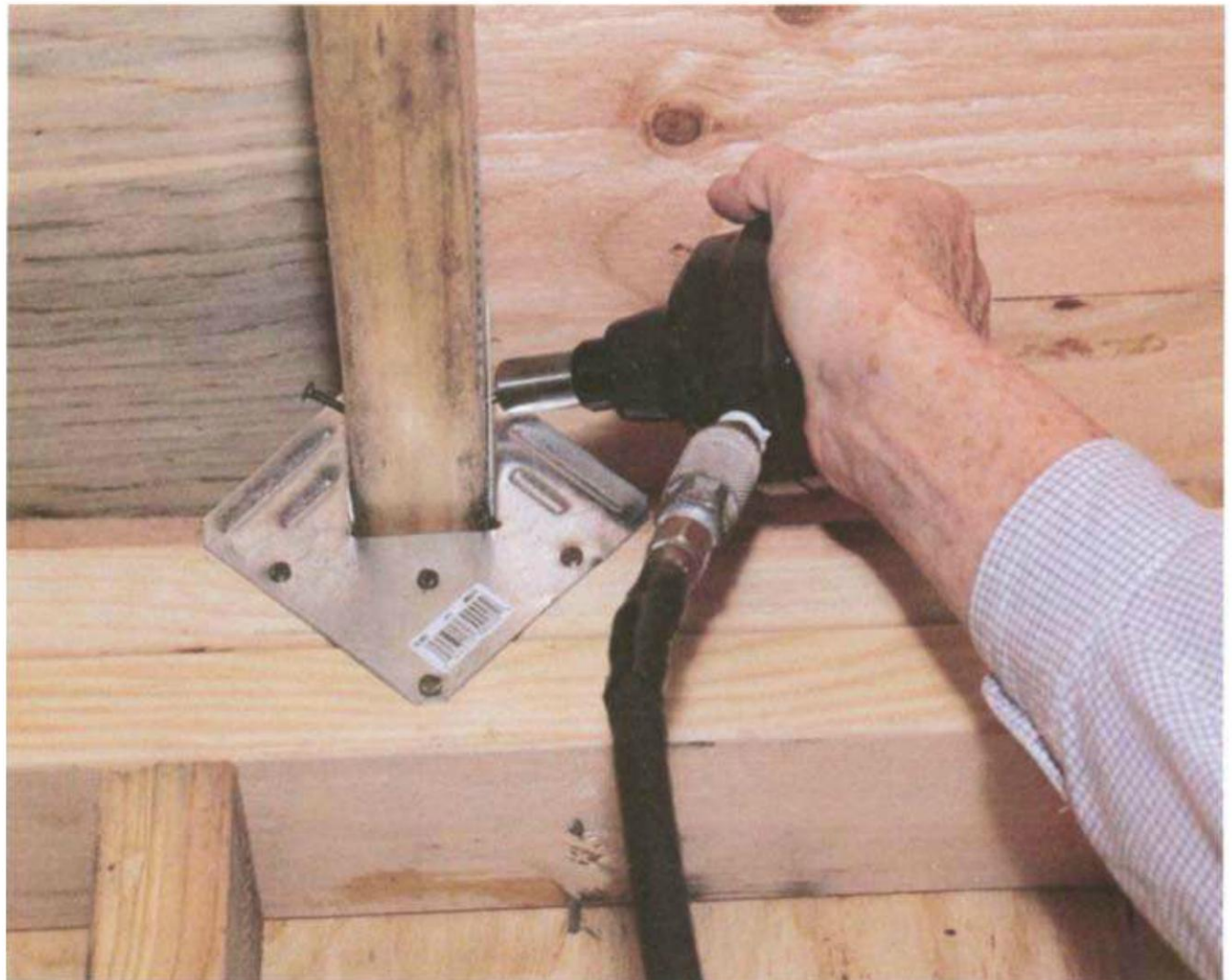
A palm nailer can drive nails in tight places, as when installing a joist hanger. (Photo by Roe A. Osborn.)
