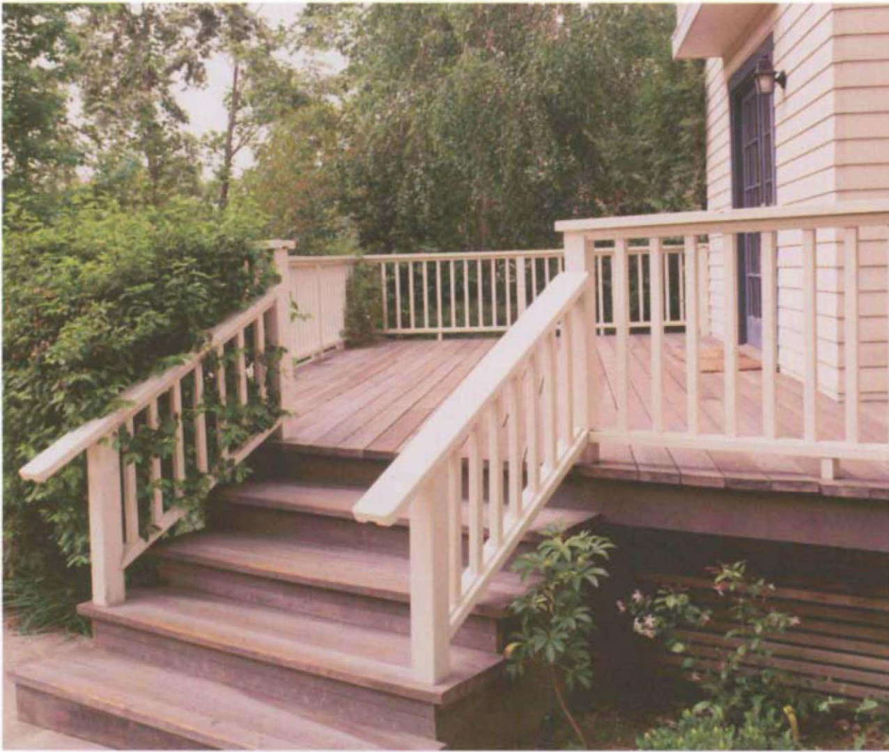
A simple outdoor handrail or guardrail for stairs and decks can be made of naturally rot-resistant wood, such as cedar or redwood, or pressure-treated wood. (Photo by Dean Della Ventura.)
