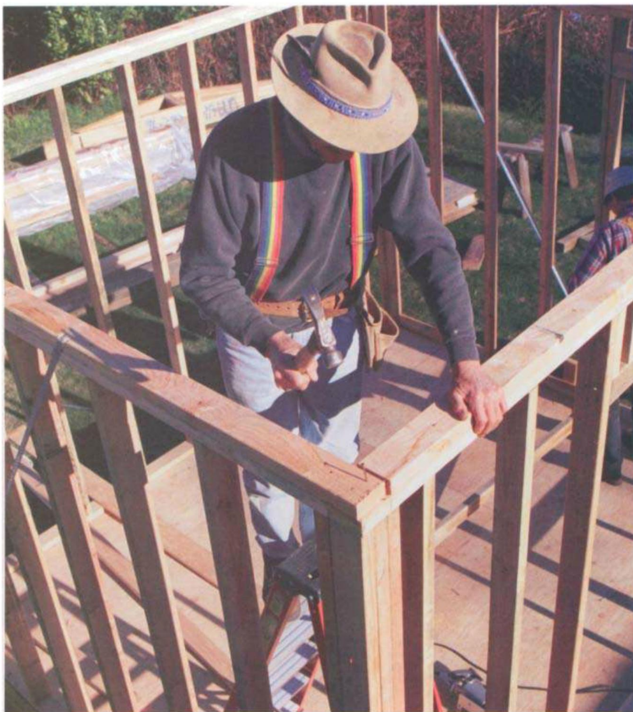
Drive two 16d nails through the overlapping double top plate of the butt wall into the top plate of the through wall. (Photo by Roe A. Osborn.)
