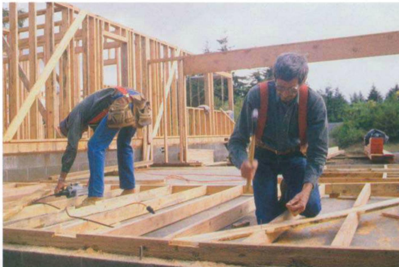
Studs are the vertical members that make up the frame of a wall and usually are spaced 16 in. o.c. or 24 in. o.c. (Photo by Roger Turk.)
