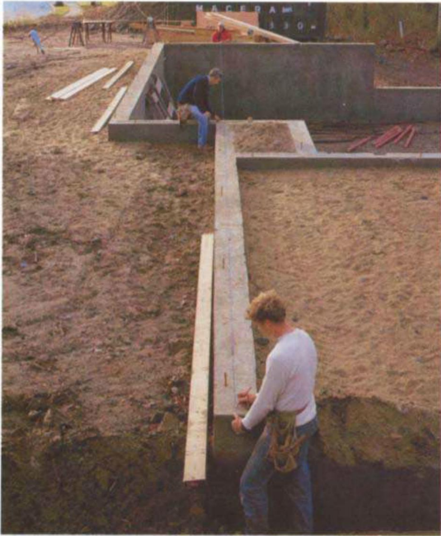
A house foundation can be a combination of full concrete basement and concrete stemwalls enclosing a crawl space, such as shown here, or just stemwalls with a crawl space, a concrete slab, or concrete piers on footings. (Photo by Roe A. Osborn.)
