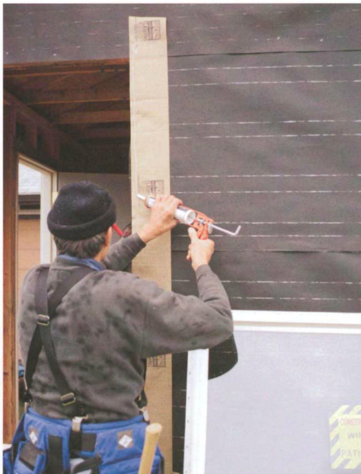
Before nailing the window in place, lay down a good bead of silicone caulk around the entire opening under the window flange. This helps keep water from entering around the window frame. (Photo by Roe A. Osborn.)
