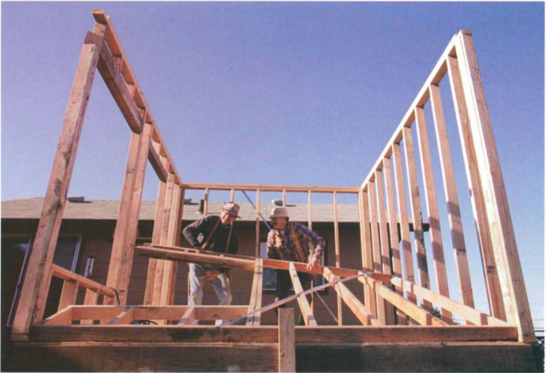
After the first wall is done, nail together another outside through wall, raise it, and brace it. Then build and raise the butt walls. (Photo by Roe A. Osborn.)
