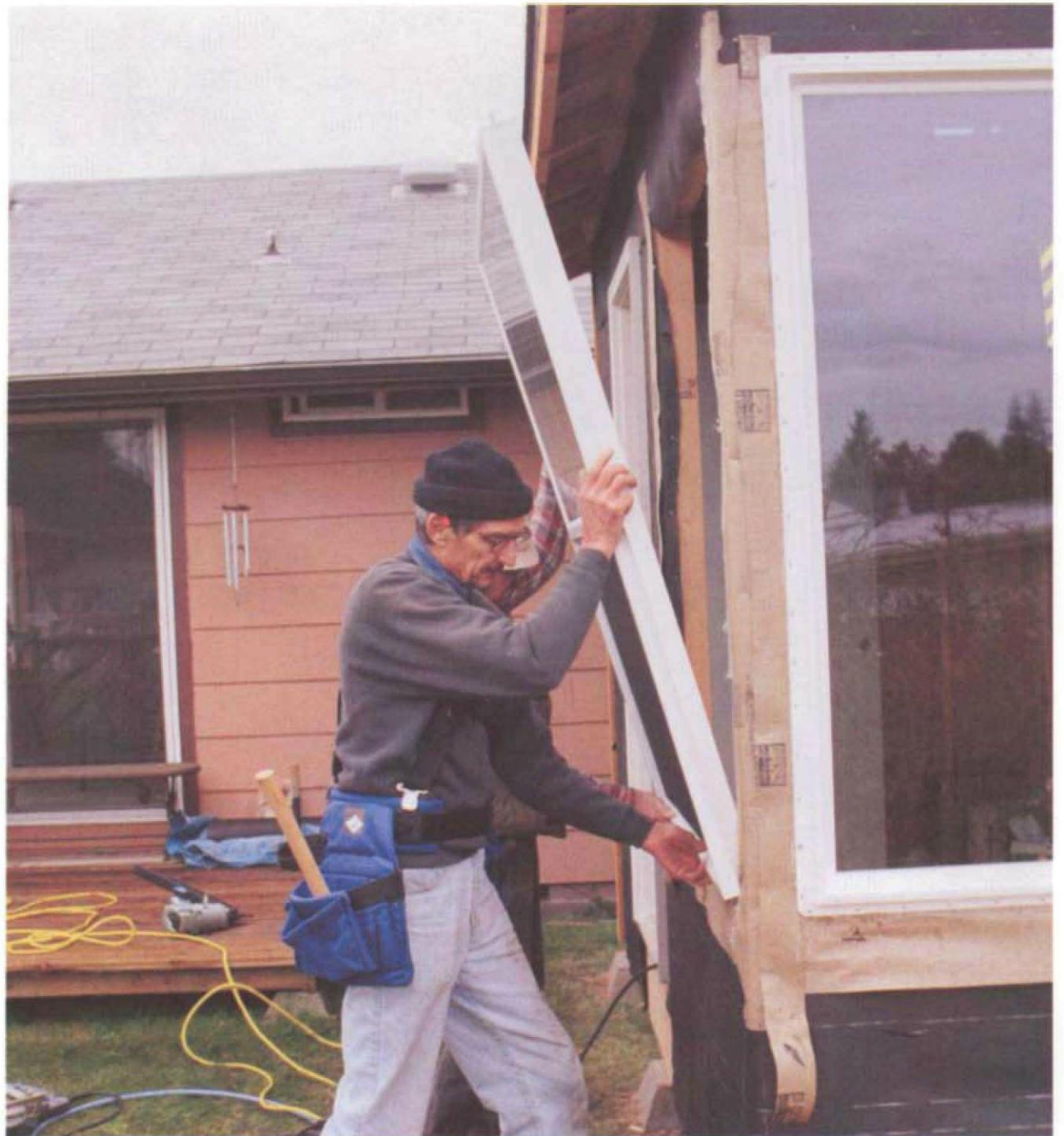
If the framing is correct, a window should fit easily in its rough opening. (Photo by Roe A. Osborn.)
