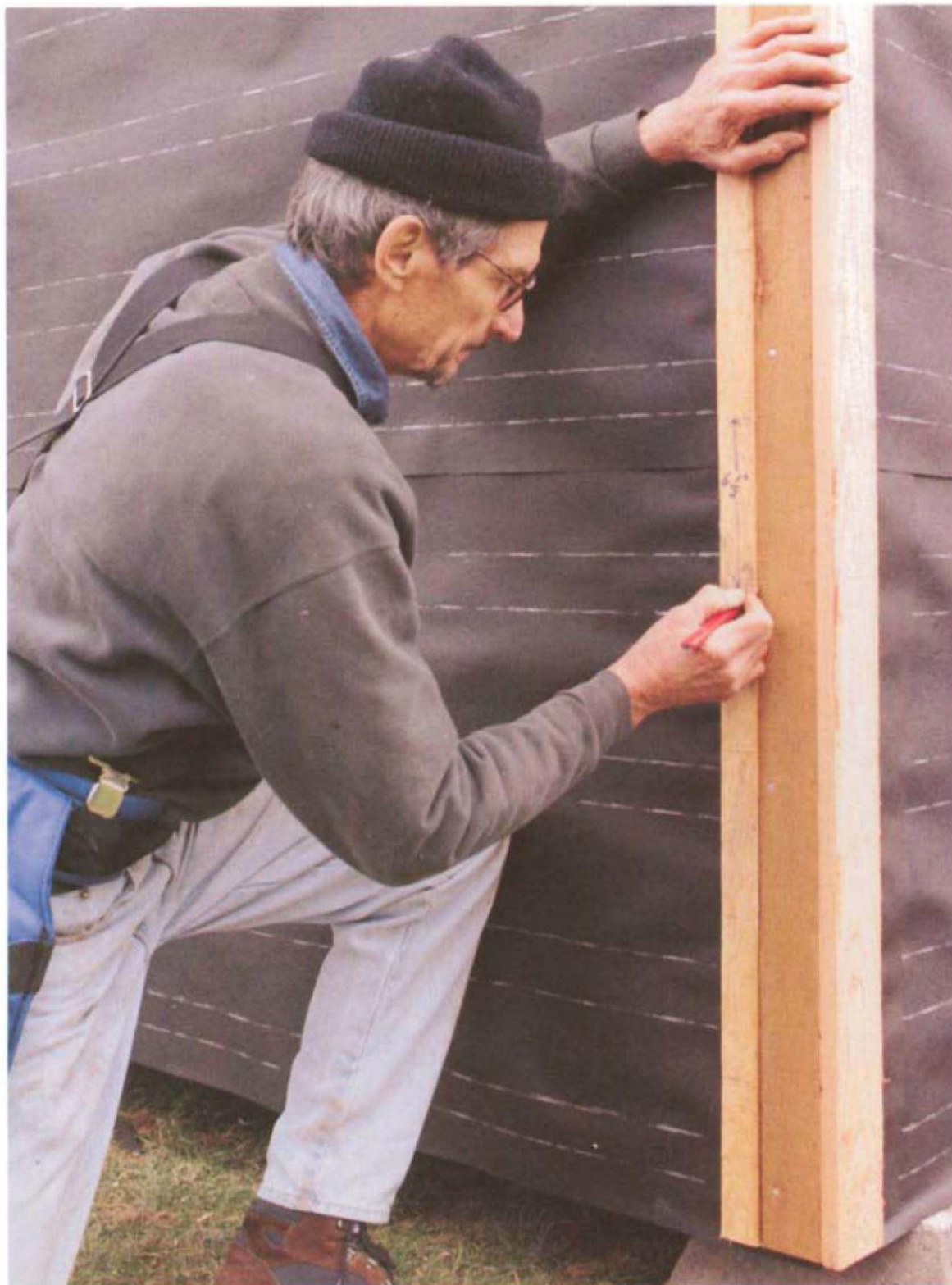
Transfer the marks on the story pole to each piece of vertical house trim. The marks will ensure that the siding will be the same height on all sides of the house. (Photo by Roe A. Osborn.)
