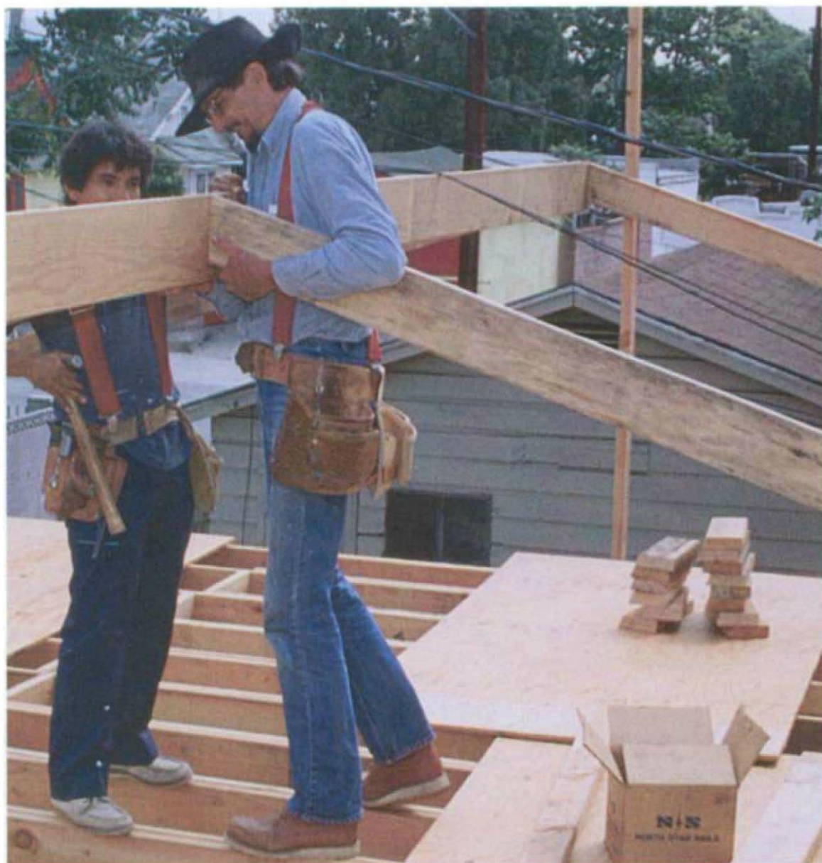
Toenail a pair of rafters to the top plates, then raise the ridge board between the rafters. Nail the rafters to the ridge board with 16d nails. (Photo by Robert Wedemeyer.)
