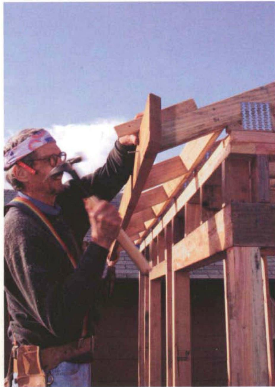
Place a piece of scrap wood on the top edge of a rafter extending beyond the rafter tail. Put the fascia snug against this scrap and drive one 16d galvanized nail high and another low. (Photo by Roe A. Osborn.)
