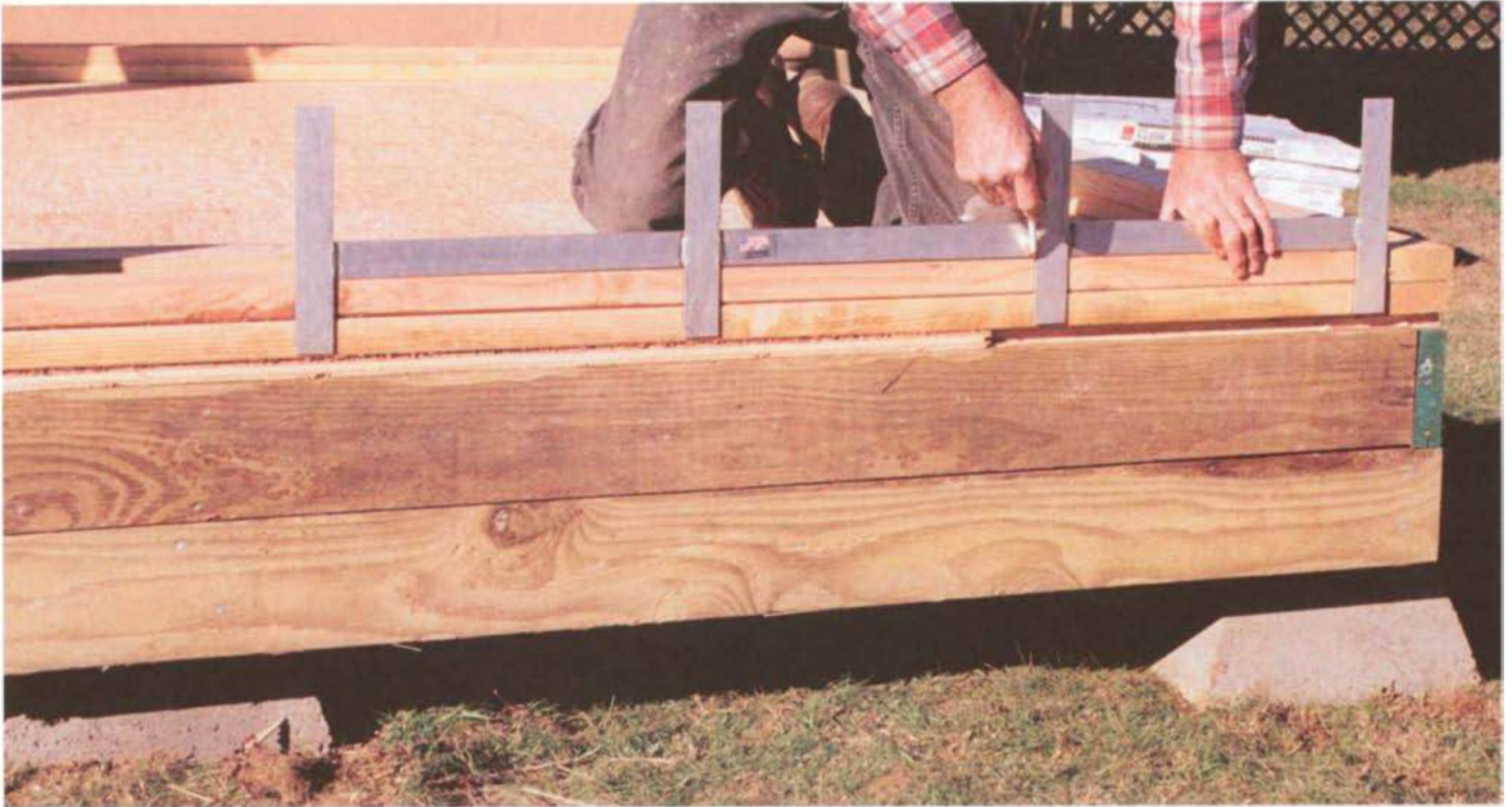
Use a layout stick to mark stud locations on wall plates. (Photo by Roe A.Osborn.)
