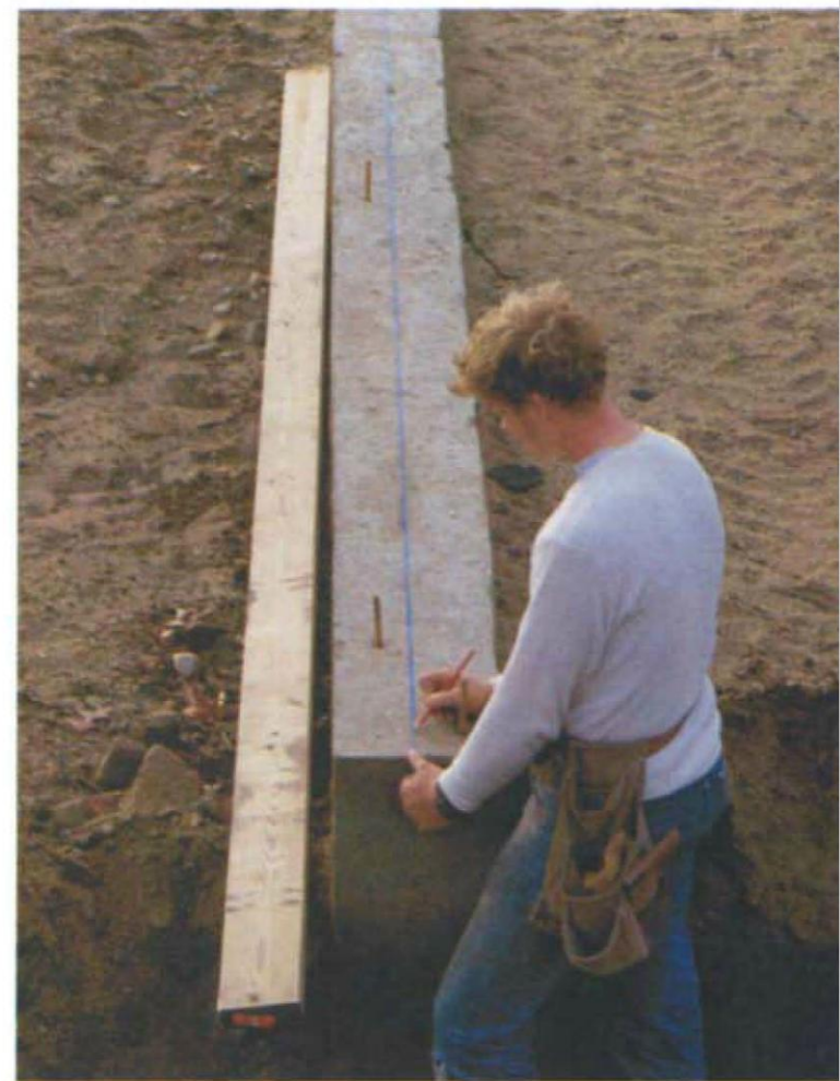
Chalklines on top of the concrete foundation indicate the position of the sill plates. (Photo by Roe A. Osborn.)
