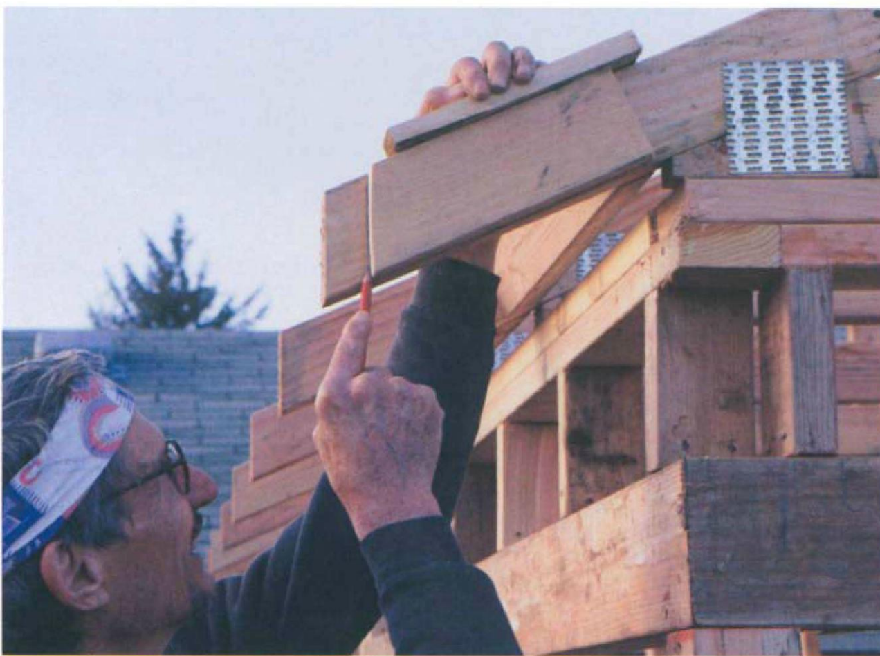
Place the fence of the rafter-cutting template on each rafter and scribe a plumb-cut line at the mark. (Photo by Roe A. Osborn.)
