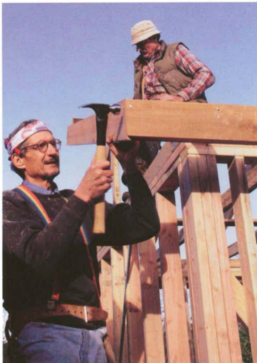
Drive two 16d hot-dipped galvanized nails through the barge rafter and into the fascia. Make sure the miter joint is tight because it will be seen. (Photo by Roe A. Osborn.)
