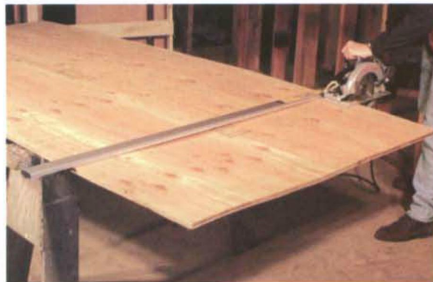
A straightedge ensures a straight crosscut.
