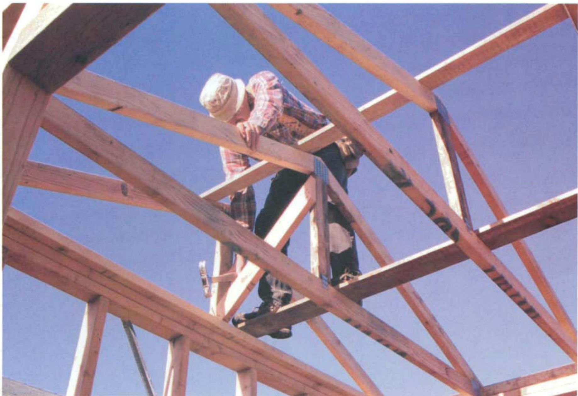
Sway braces at the gable ends and a catwalk on the joist chords help brace the roof. The 1x6 along the top of the rafters helps maintain the truss spacing until the sheathing is installed. (Photo by Roe A. Osborn.)
