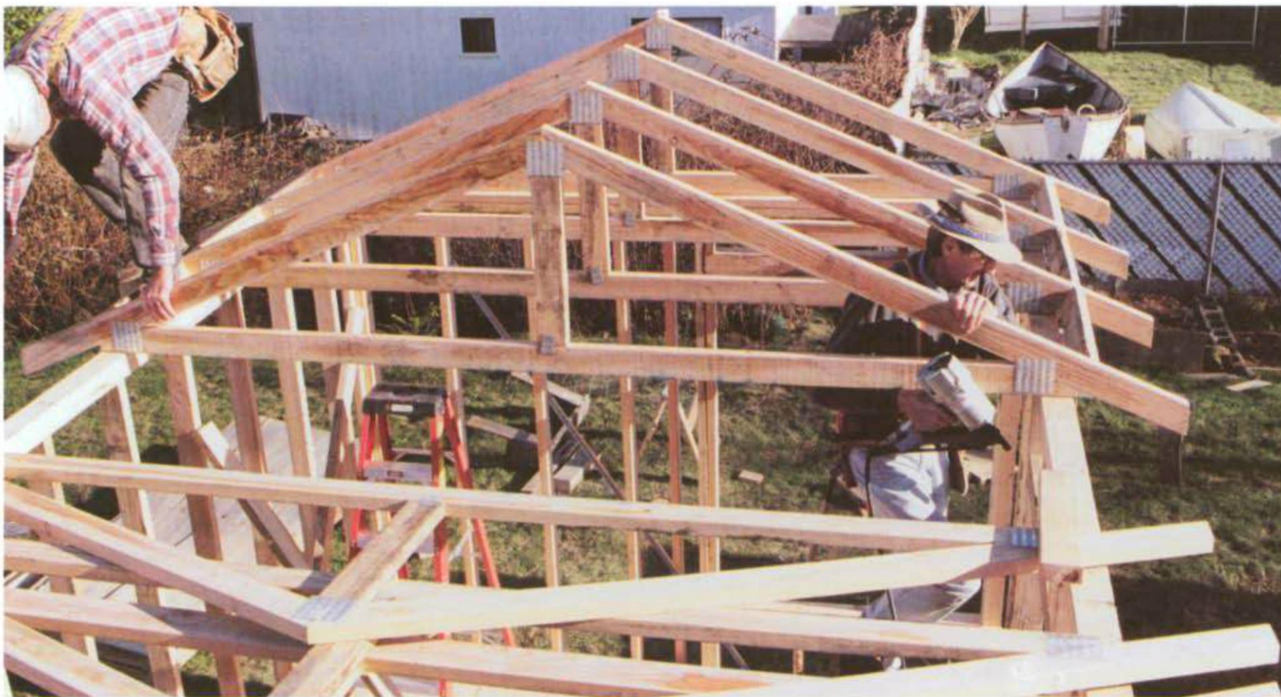
Roof trusses, which are delivered to the site fully assembled, simplify roof construction. Notice the frieze blocks (on right) between these king-post trusses, which help tie the whole roof together. (Photo by Roe A. Osborn.)
