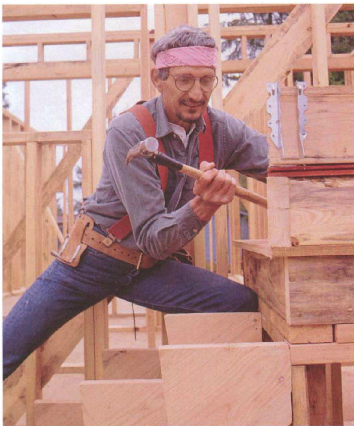
Even complicated stairs become easy when broken down into simple tasks. (Photo by Roger Turk.)
