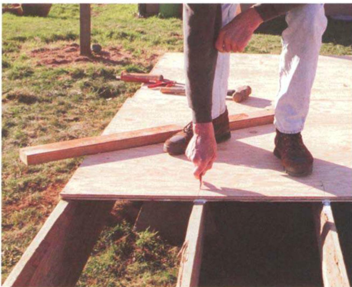
After each row of sheathing has been installed, mark the joist location on top at the leading edge so you will know where to drive the nails. (Photo by Roe A. Osborn.)
