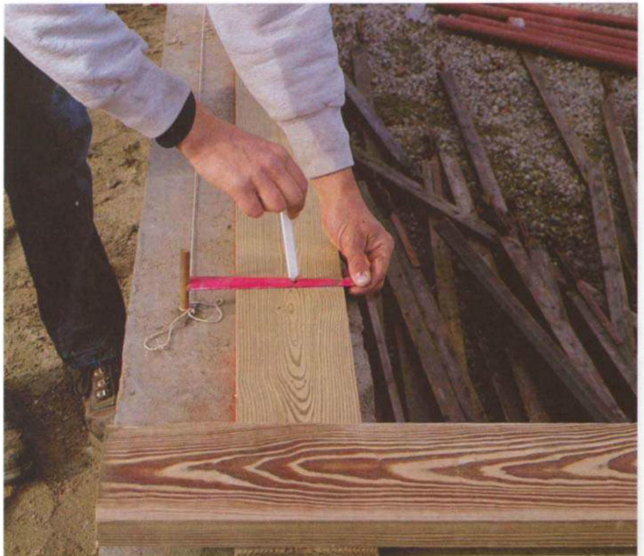
A simple measuring device called a bolt marker can be used to locate the bolt holes. With the sill plate lined up on the inside of the chalkline, hold the end of the marker against the bolt and mark the bolt hole. (Photo by Roe A. Osborn.)
