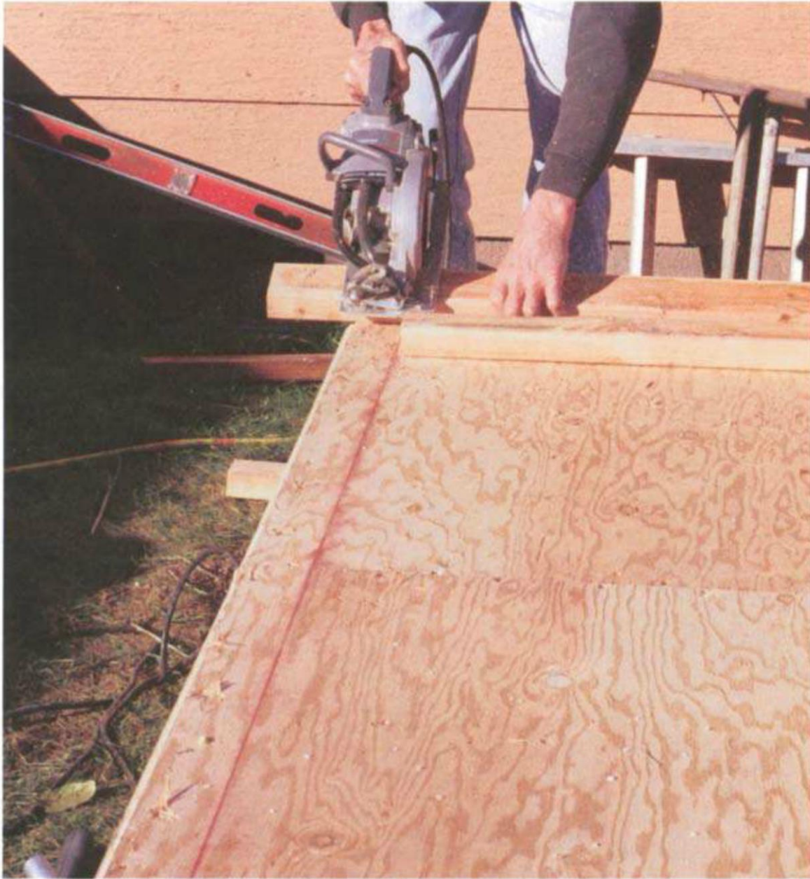
Once the wall layout is complete, it's time to lay down top and bottom plates. Eventually, when you frame the wall, a third plate will be nailed to the top plate. Here I'm cutting a bottom plate to length. (Photo by Roe A. Osborn.)
