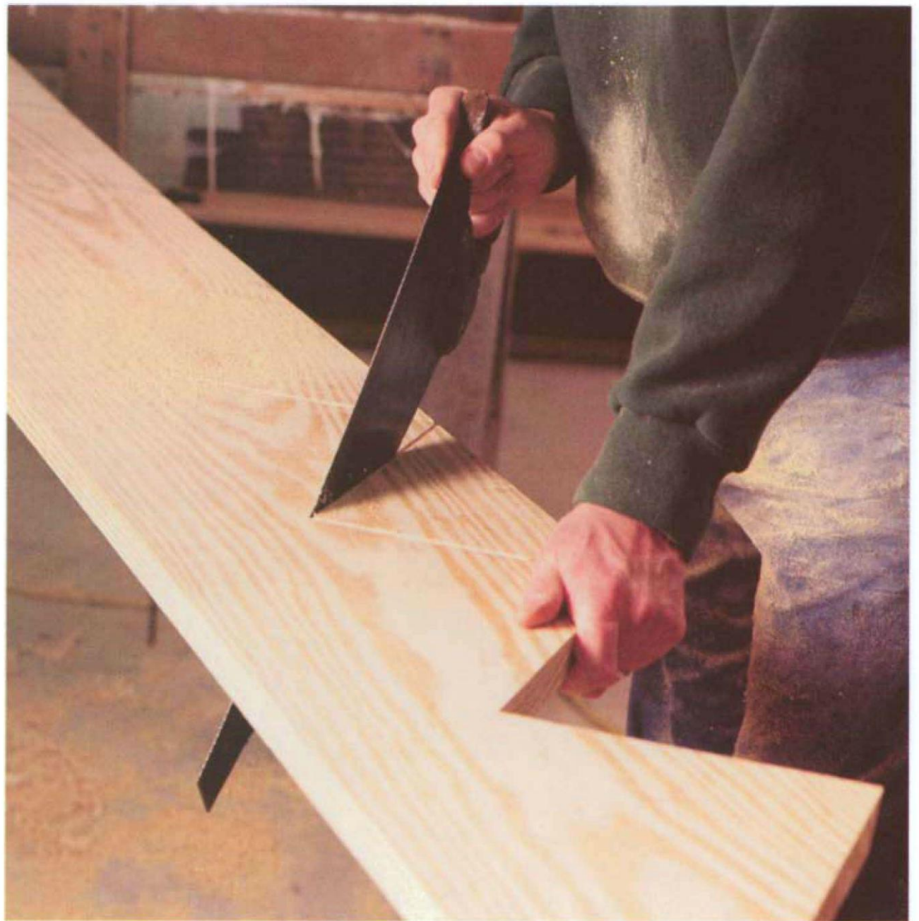
The notch in the rough stringers can be overcut with a circular saw. If the stringers are exposed, finish the cut with a handsaw or jigsaw. (Photo by Scott Phillips.)
