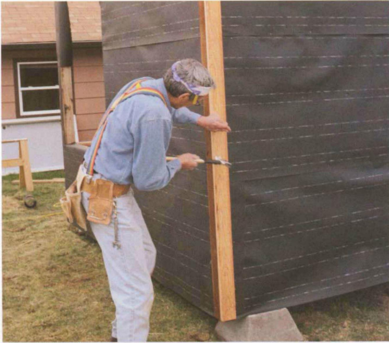
At the corners, I often nail a 1x3 on one side and install a 1x4 on the opposite side so that it laps the 1x3. Once lapped, both trim pieces look like a 1x4. (Photo by Roe A. Osborn.)
