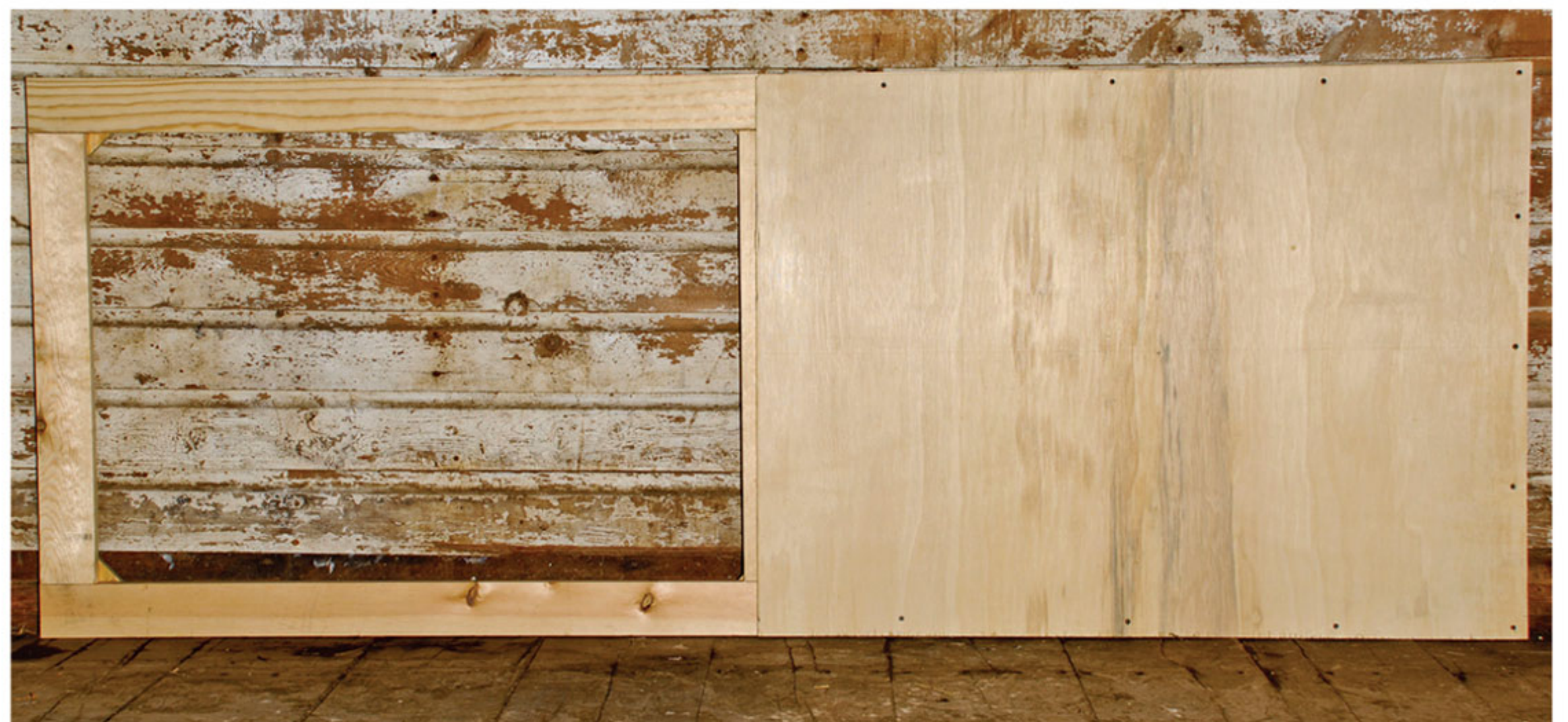
Exterior of a side panel, ready for paint. Note that the design accounts for shade and protection from harsh elements as well as fresh air and ventilation.
