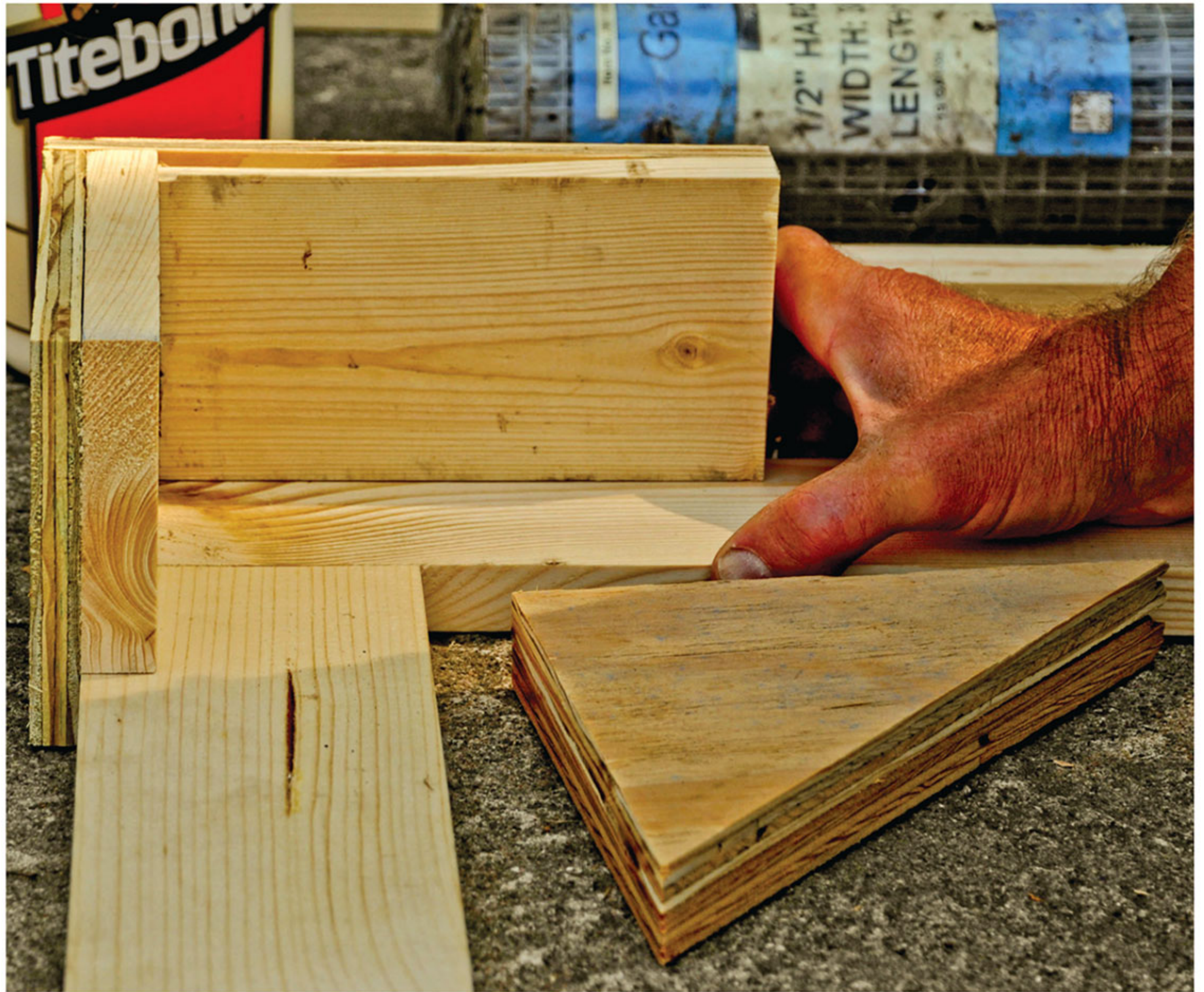
Constructing a corner jig ensures that all frame pieces will end up square, and it can also help with construction of the J gussets.
