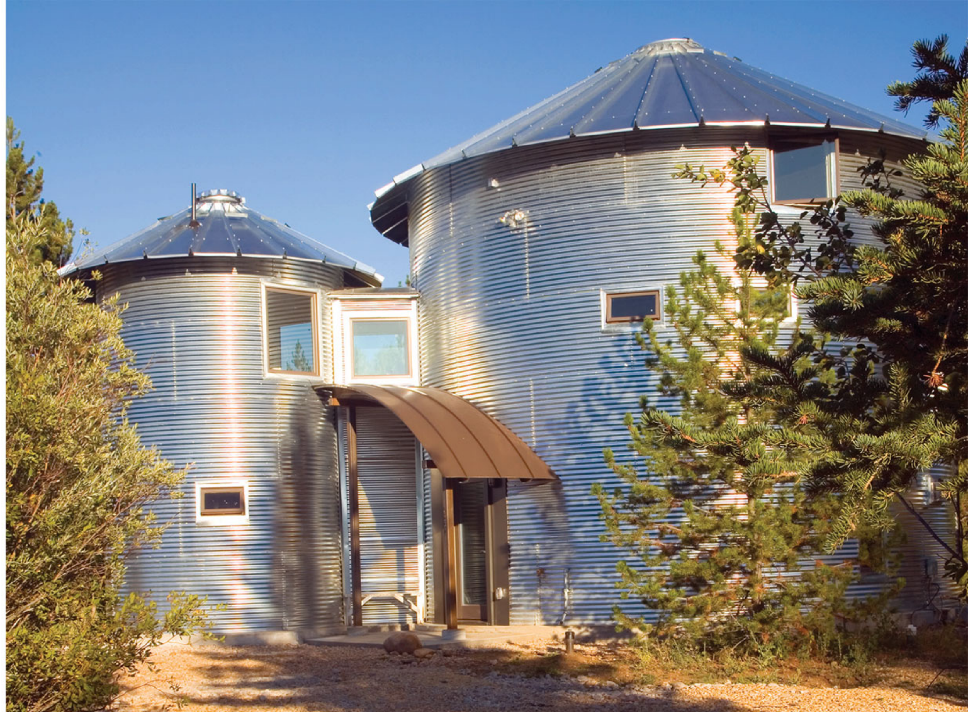
Two bins create this home in the Uinta Mountains of Utah. OPPOSITE: An energy-efficient grain bin house uses foam and fiberglass insulation, plus computer-assisted passive solar heating.
