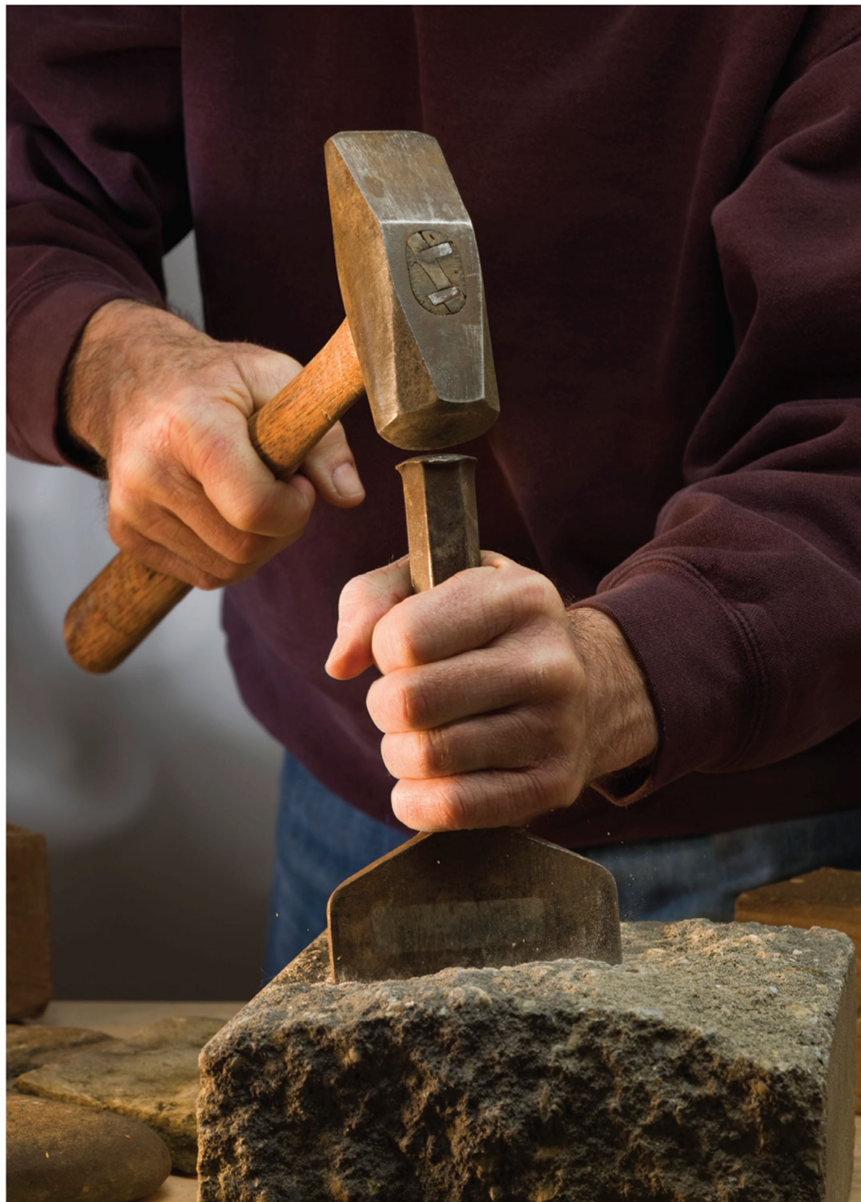
A stone mason uses a hammer and chisel to shape stone. OPPOSITE: David Reed's completed stone culvert with flared wing walls.
