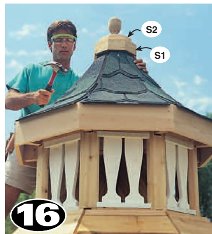
16 SHINGLE THE CUPOLA before shingling the lower roof. Otherwise, you'll damage the lower shingles when you go up and down.
