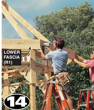
14 NAIL THE LOWER FASCIA (R1) to the rafter tail ends. Miter the ends with the saw set at 22-1/2 degrees.
