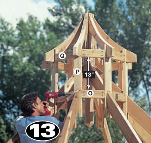
13 SCREW THE HORIZONTAL RAFTER TIES to the sides of each outer vertical rafter tie.
