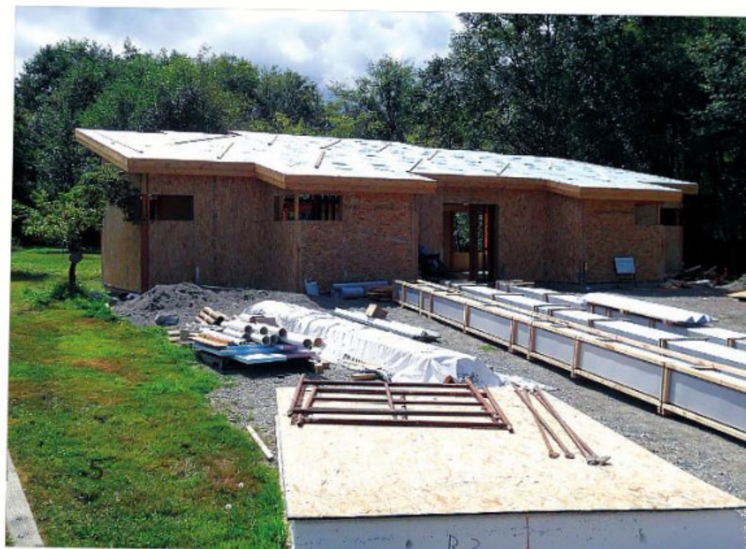
3. Once the frame is raised, it's ready to be enclosed with exterior walls and roofing. The frame will remain visible on the inside of the finished home.
