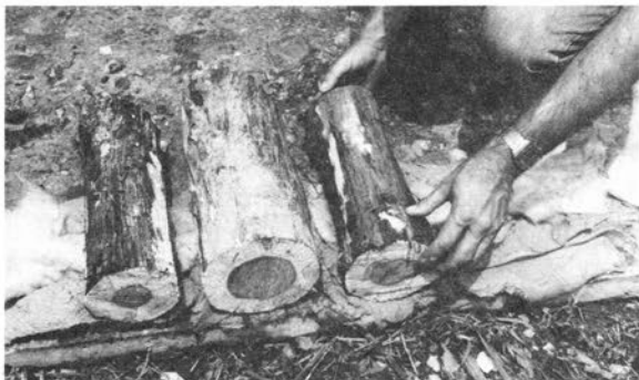
Step 2. Bed the short logs across the mortar.
