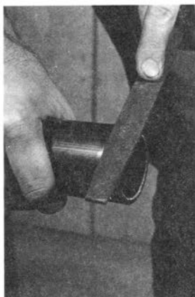
Remove burrs on the end of pipe with a file or knife, or with sandpaper. Lightly touch up the outside edge.
