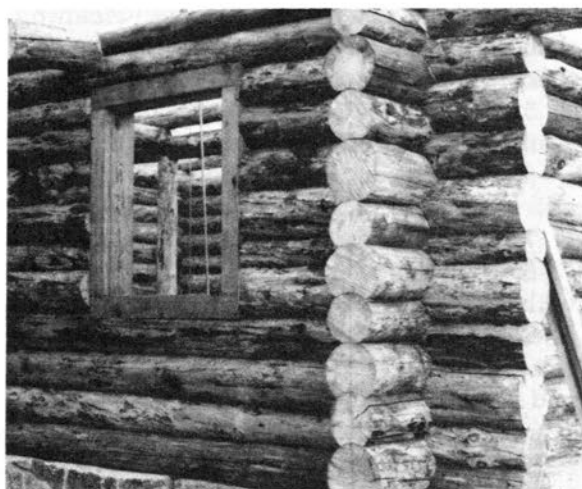
This is a student-built house at Pat Wolfe Log Building Courses.
