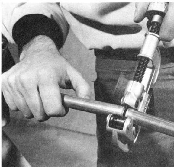
Step 1. Copper tubing is easily cut with a special pipe-cutting tool.
