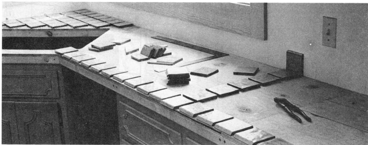
If you cover a counter with ceramic tile, the plywood top must be installed first. The ceramic tile laid into a bed of mastic and then grouted. Then the sink installed. (Photo courtesy American-Olean.)
