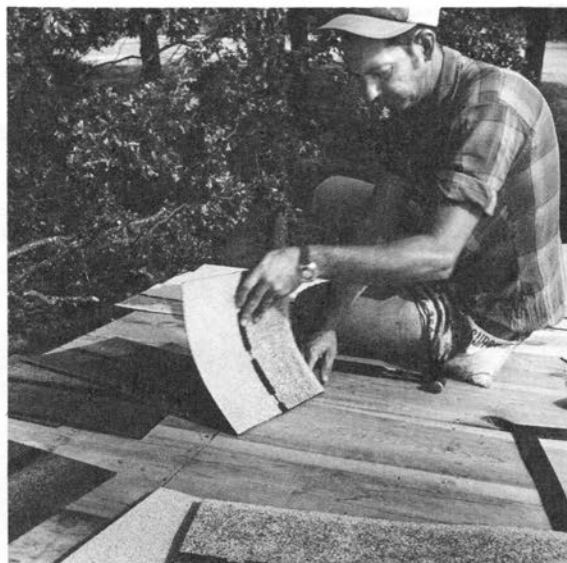
After scoring the shingle, tear it apart.
