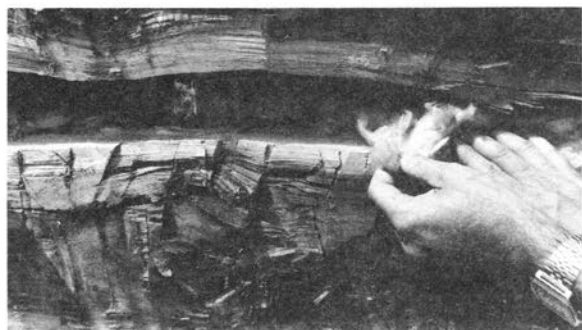
Step 1. For modern mortar chinking, fill the space between the logs with fiberglass.
