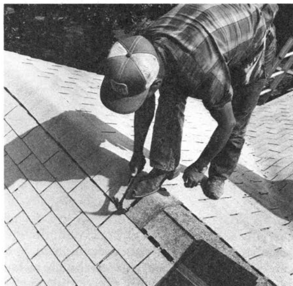
The roof peak is finished by cutting individual tabs from a shingle and overlapping them.
