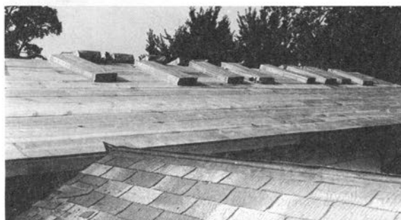
Place bundles of asphalt shingles and other roofing materials on the roof in convenient locations.
