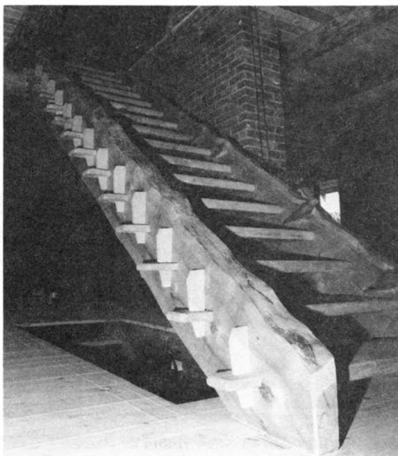
Milled slabs allow pegging of mortises and tenons, shown in these stairs by Building with Logs Ltd.
