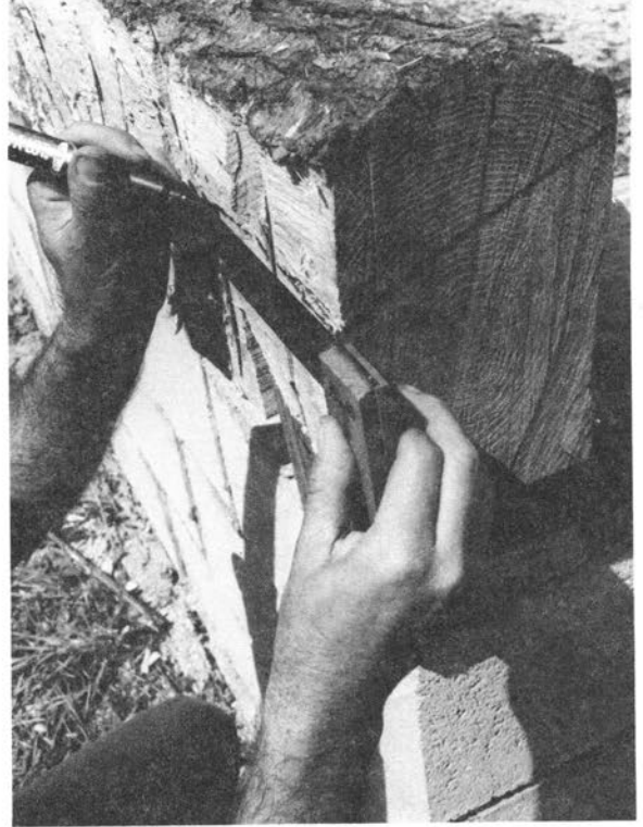
Step 12. Continue the rest of the marking to match and cut.
