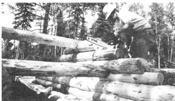
Purlins help hold the gable end logs in place. (Photo by Minnesota Trailbound School of Log Building.)
