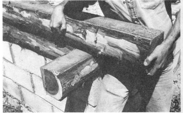
The second course overlaps and butts in the opposite direction. All logs are anchored with spikes.
