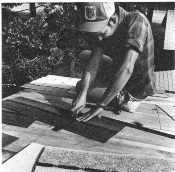
To cut a shingle, score across the back with a sharp utility knife using a carpenter's square as a guide.
