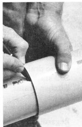
Check the fit before you weld. Mark both fitting and pipe so you can align them properly.
