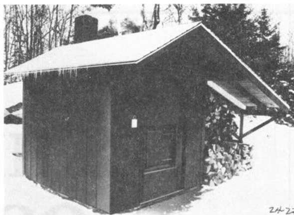
One alternative that many are considering these days is a HAHSA, (heating and heat storage apparatus), which is a furnace hut that sends heated air into your home. (Photo courtesy HAHSA Co.)
