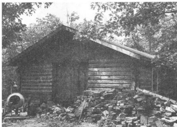
A tremendous pile of stones goes into the construction of a fireplace and flue.
