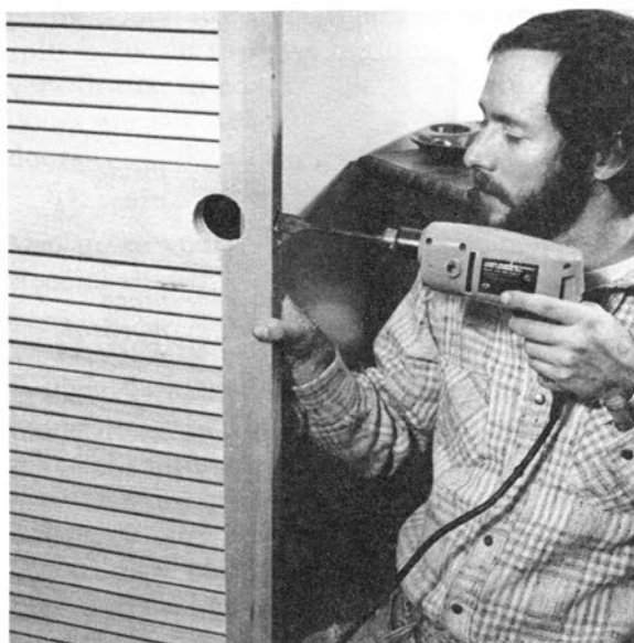
Step 9. Bore the side hole with a paddle bit.
