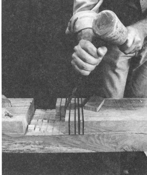
Large chisels remove the wood between the cuts.
