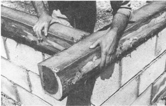
Here is a simple butt joint.
