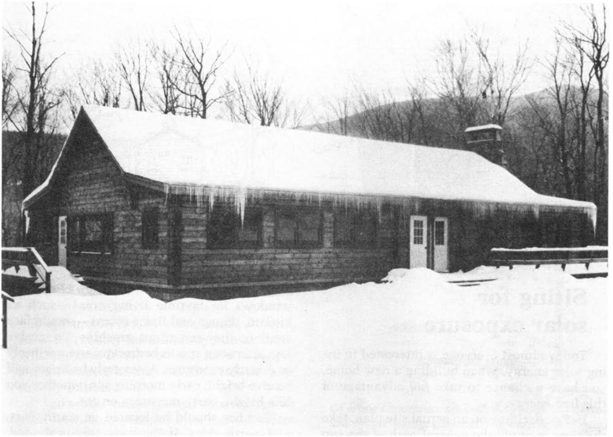
Knowing about local weather conditions helps you choose the correct roof design. Areas that receive heavy snowfall tend to require more steeply pitched roofs than shown here. (Photo courtesy Alta Industries, Ltd.)
