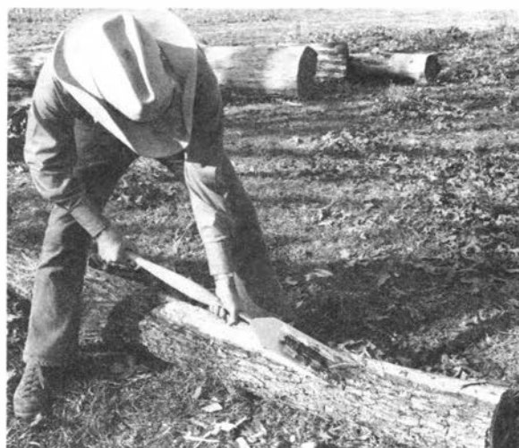
The logs should be peeled. This is best done after they have been hauled to the building site. During hauling the bark will protect the surface of the log from hauling damage. Peel with a peeling spud.
