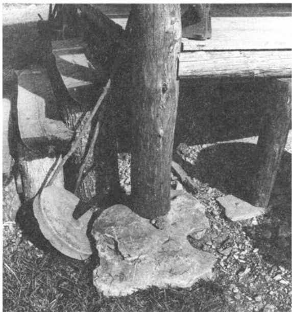
Decks and porches have been built simply with flat rocks for supports.
