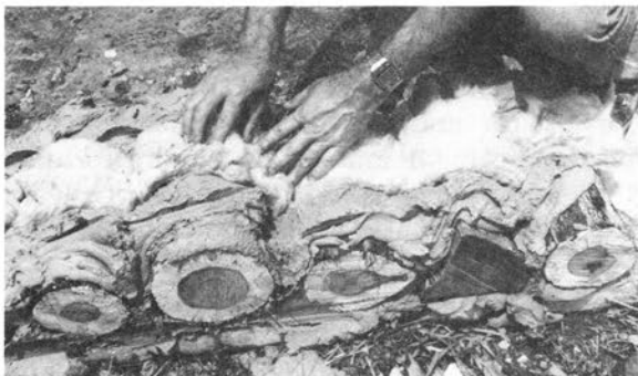
Step 3. Place more mortar and insulation around the logs as you go.
