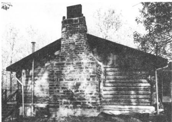
A competent mason with a knowledge of fireplace design can construct a full masonry fireplace. It's not a job for the average do-it-yourselfer.
