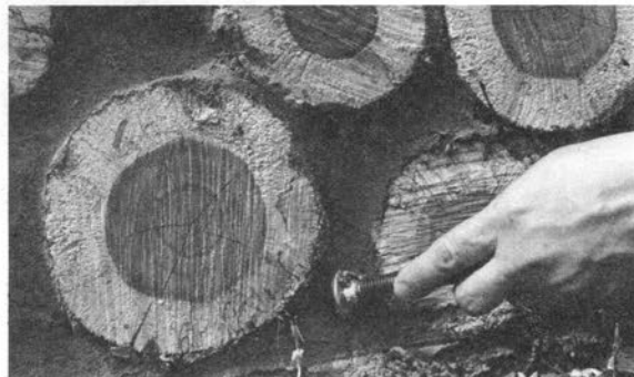
Step 4. After the mortar has somewhat set, it's tuck-pointed, or smoothed back, around the log ends.
