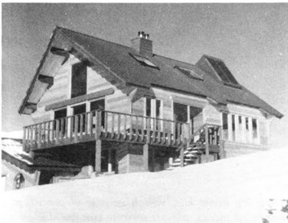
Many modern kit models take full advantage of the heat-retaining mass of logs and passive solar engineering. (Photos courtesy Justus Log Homes, Inc.)
