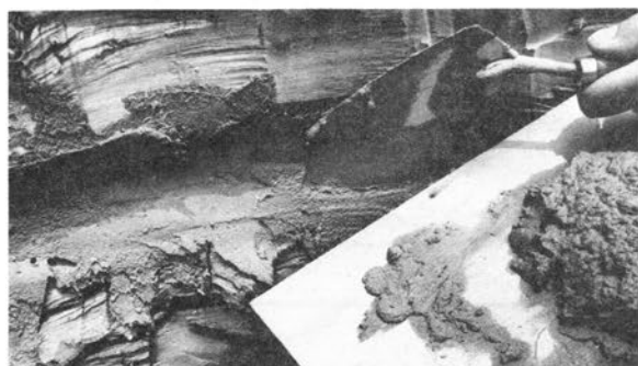
Step 3. Apply the mortar through and onto the mesh.
