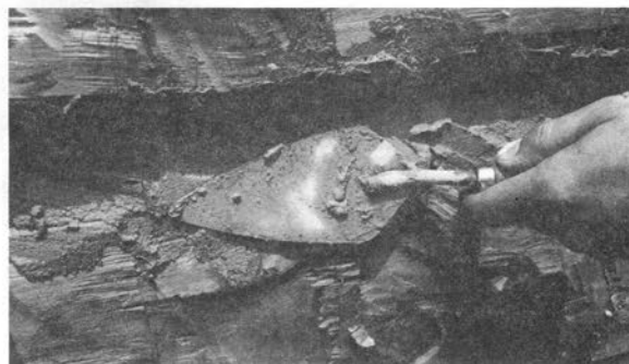
Step 4. Trowel the mortar to finish the job.
