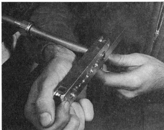
Step 3. A flaring tool readies flexible tubing for fitting. Note: The fitting's flare nut must be installed first.
