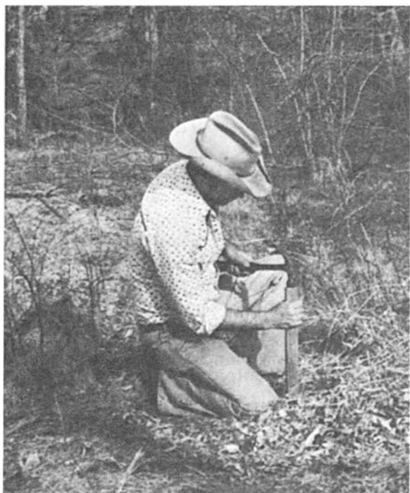
Once your site is leveled and cleared you can temporarily stake out the rough outlines of your home.
