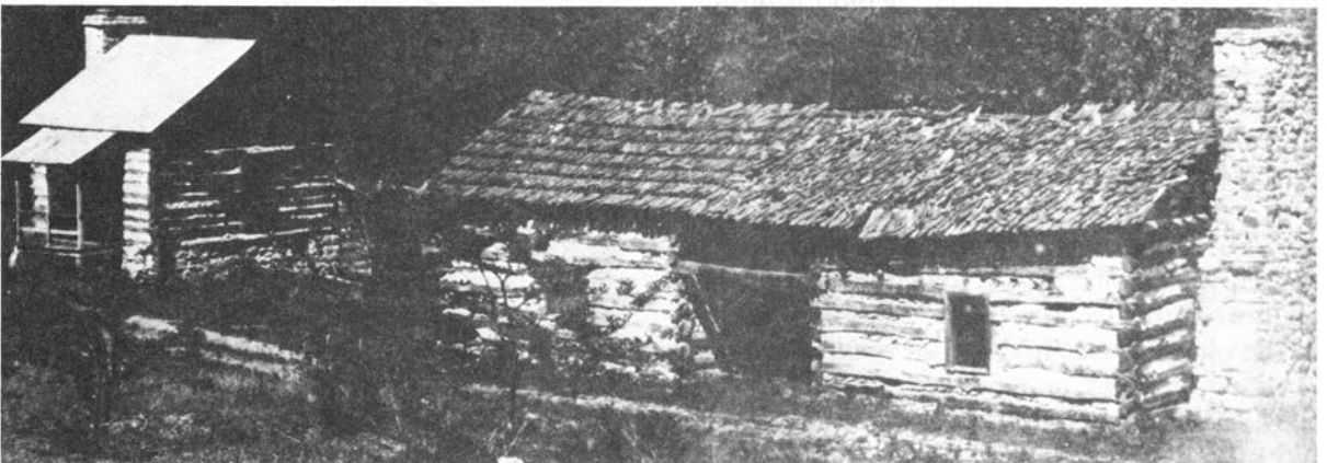
Above, many fine examples of this hewed log style are scattered across North America. Below, the dogtrot log home was once common. This consisted of two small log rooms joined by a breezeway. (Photo courtesy Historical Society of Missouri.)
