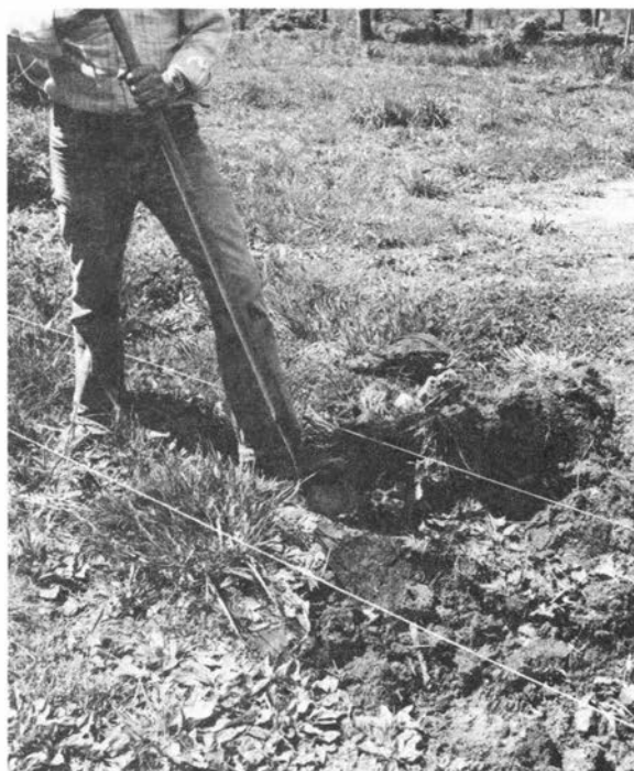
Small foundations, even water or sewer lines, may be dug by hand, soil and locality permitting.
