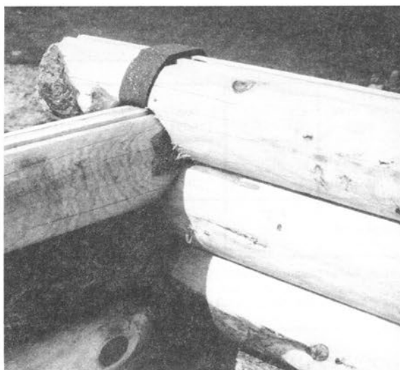
The foam sealer may run into the corner joint. (Beaver Log Homes)
