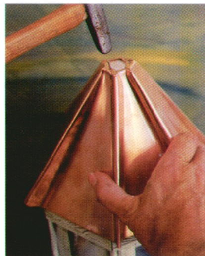
The dowel will need to be trimmed slightly so that the roof can be hammered over it.
