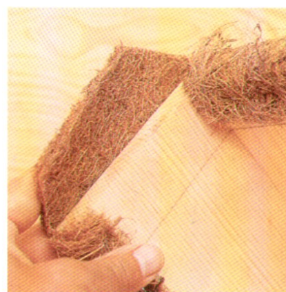
Notch the mat, trim it to the pencil lines, and staple on the underside of the eaves.
