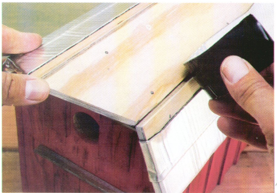
Roof your barn with flashing material cut into strips and laid in an overlapping pattern.
