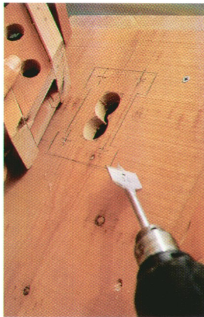
Drill overlapping 1¼-inch holes inside the ventilator "footprint" to form a figure 8.
