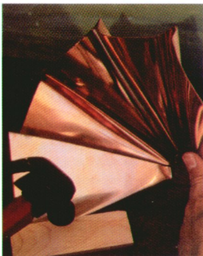
When bending and shaping the roof, use a scrap block to cushion the hammer blows.
