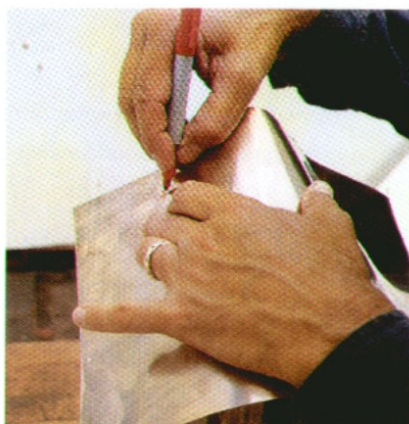
At the midpoint of each roof hollow, mark the location of the brass screws.
