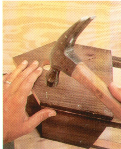
Use 3d galvanized finishing nails to attach the front of the house to the side walls.
