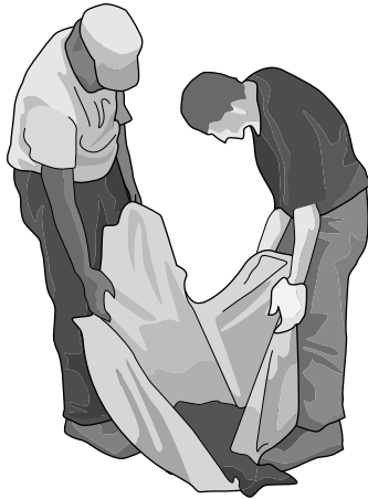
Figure 6-7: The Cretesheet is a tool-free way to mix concrete and pour it where you want it.
