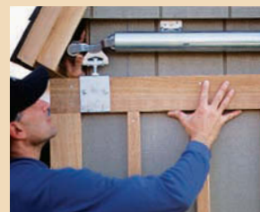
Door Installation p. 141
