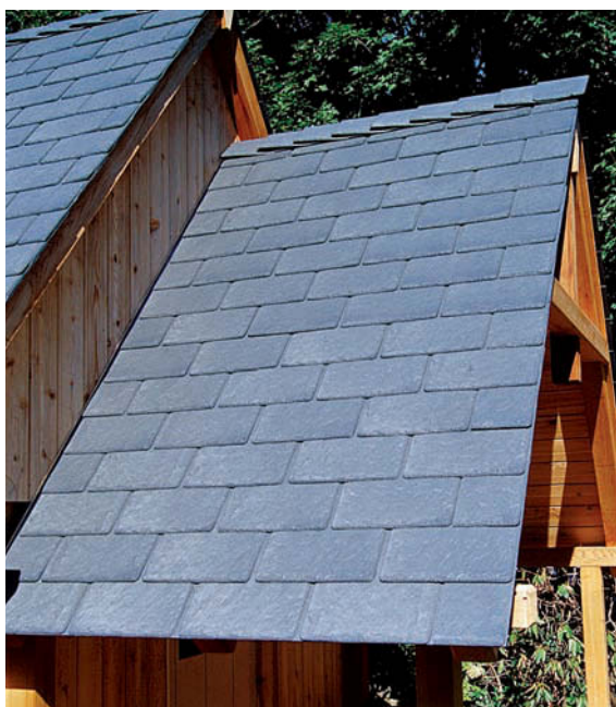
The realistic muted gray colors and embossed surface of this faux-slate roof are almost indistinguishable from real slate.
