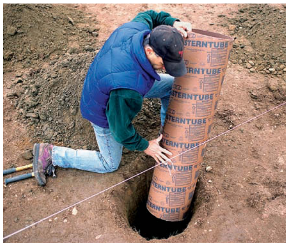
Fiber-form tubes are commonly used to build permanent, frost-proof foundations. Each tube is set in a hole dug below the frost line, then filled with concrete.
