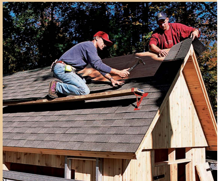
Lay a sound 2×8 plank across the three roof brackets and continue nailing shingles all the way to the peak.
