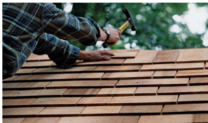
Shingles are uniformly sawn to about \frac{3}{8} in. thick, resulting in a stylish, low-profile roof that casts very thin shadow lines.
