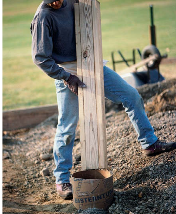
Pole-barn frames consist of round poles or square posts set in deep holes. Here, a pressure-treated 4×4 post is used.
