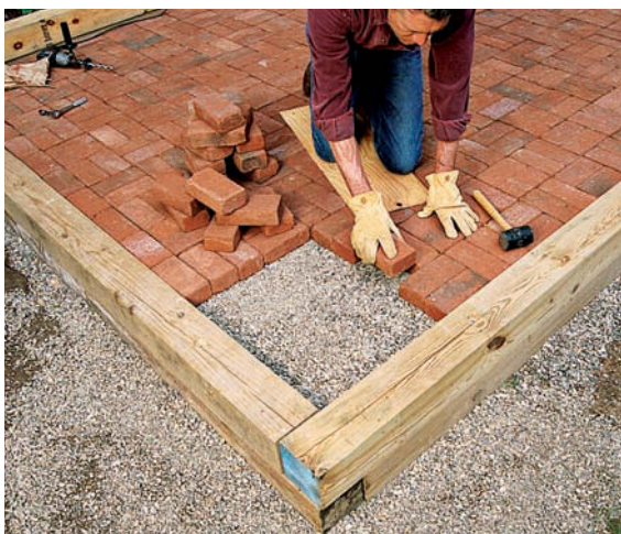
A timber-frame foundation provides a chance to lay a beautiful brick floor. Set the bricks in a bed of gravel or sand.
