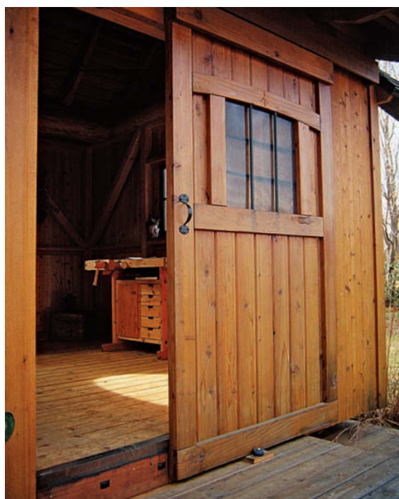
The sliding batten door on this woodshop features a large window that sports a decorative grille made of 5/8-in.-dia. rebar.
