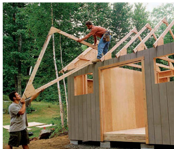
Speed the job of framing the roof by prefabricating the roof trusses on the ground. Then lift each truss into place and screw it to the walls.
