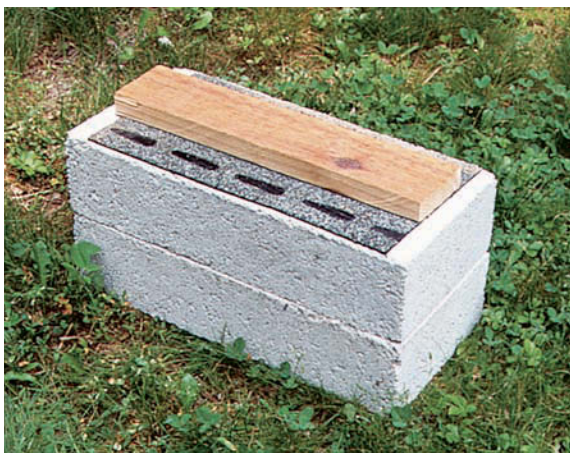
In most cases, you'll need both 2-in.-thick patio blocks and 4-in.-thick solid-concrete blocks to build an on-grade foundation.
