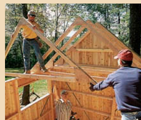
Roof Framing p. 106
