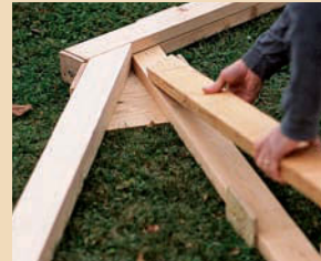
Roof Framing p. 132
