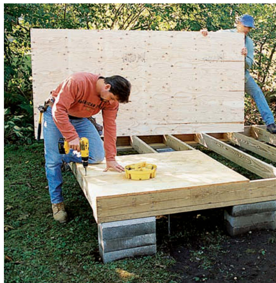
Use decking screws or ring-shank nails spaced 8 in. to 10 in. apart to attach the plywood decking to the floor frame.
