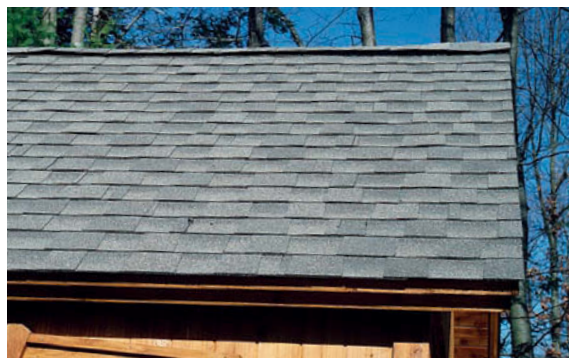
The variegated gray and black tones of these architectural-style roof shingles were designed to look somewhat like a traditional slate roof.
