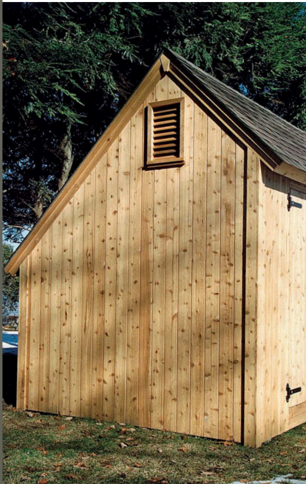
This shed is sided with tongue-and-groove, V-jointed cedar 1×6s. The knotty boards are finished with clear wood preservative.
