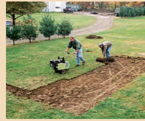
Site Prep and Footings p. 122
