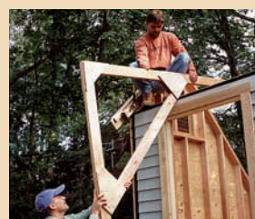
Roof Framing p. 79
