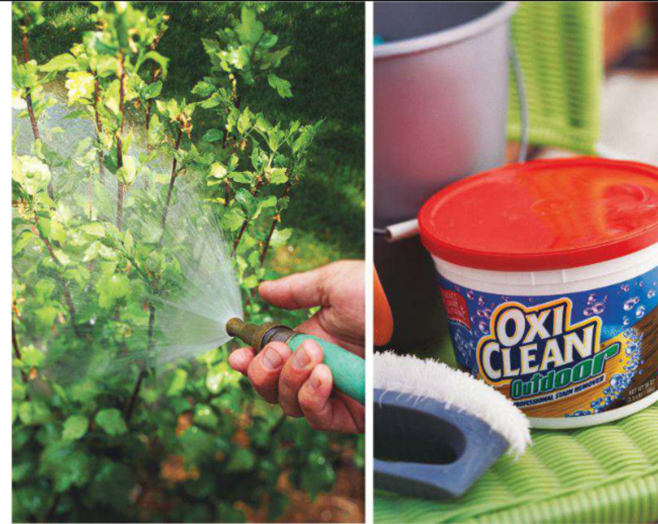
Wet nearby foliage before using deck cleaner or stripper to reduce chemical damage, above. After cleaning the deck, spray plants again to wash off any chemical residue. Oxygenated cleaners, such as the one pictured above right, are less harsh than those containing chlorine bleach.
