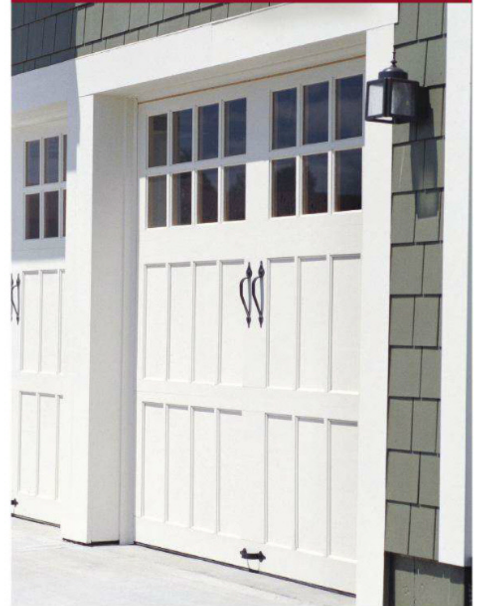
UPGRADE THE GARAGE DOORS
