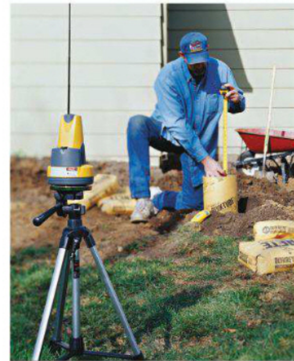
Setting concrete footings for your deck is a critical early task your builder will undertake when preparing the deck site. A laser level, like the one shown above, ensures that footings are plumb and properly placed.
