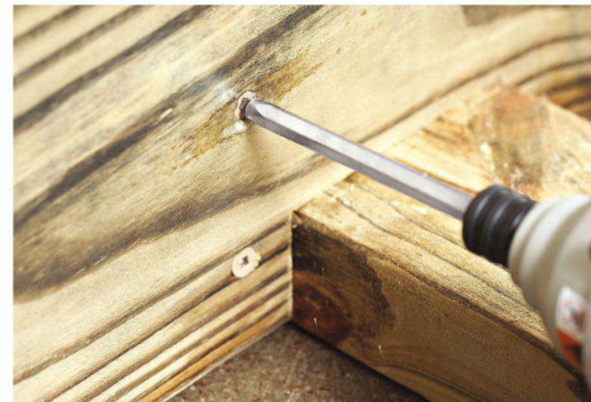
Some freshly pressure-treated lumber holds so much moisture that discolorations form around the heads of driven fasteners.
