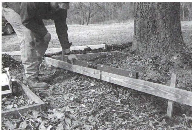
It should also be level and temporarily staked in place.
