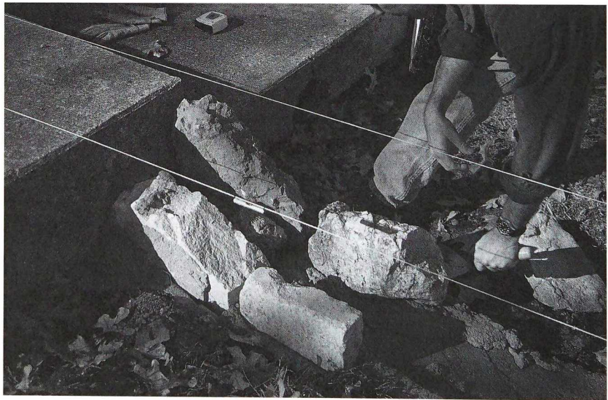
When building a mortared wall, stones are laid with an outside and inside layer, or course.
