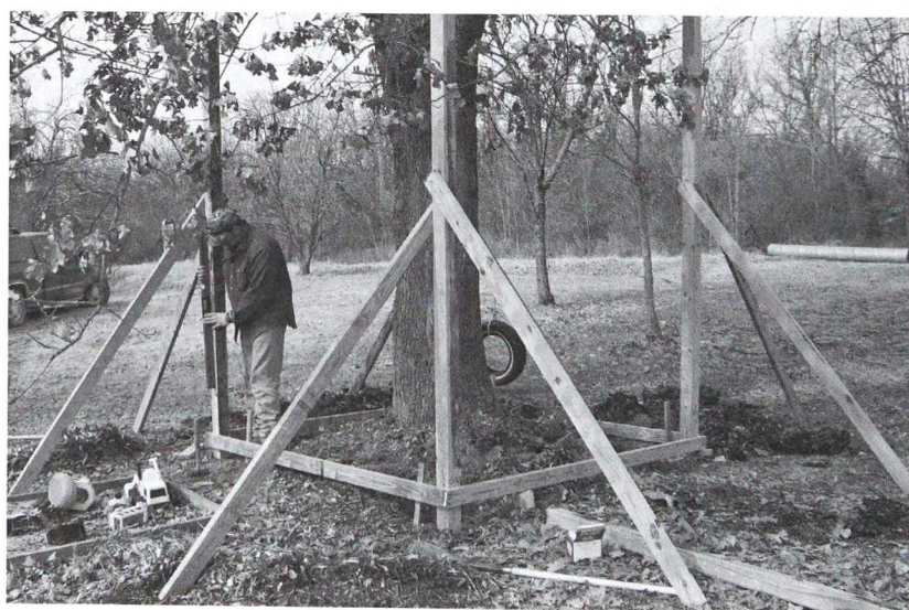
Make sure all posts are braced plumb.
