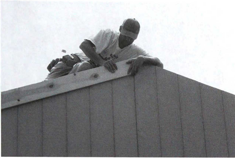
The gable rake boards installed.
