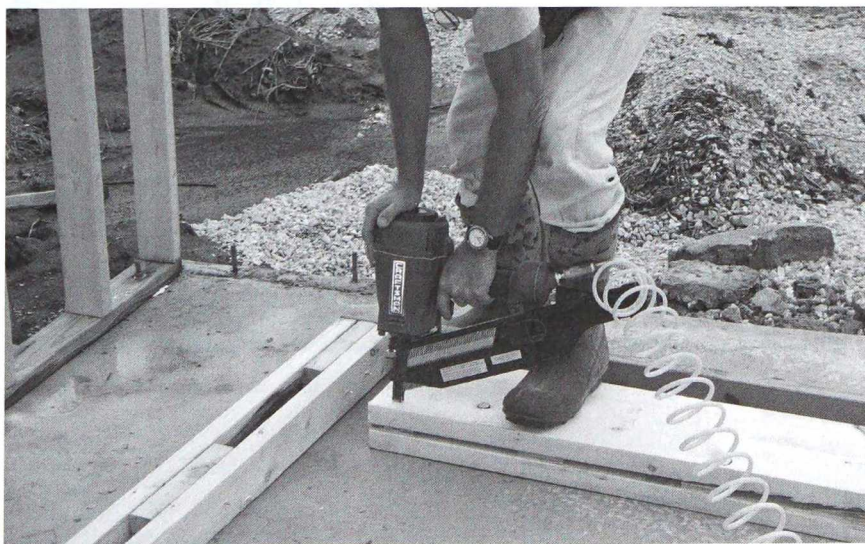
The header boards are then fastened together.
