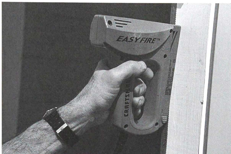
With framing complete, the porch is stained and finished or painted. Screening is then stapled in place and battens applied over the edges.
