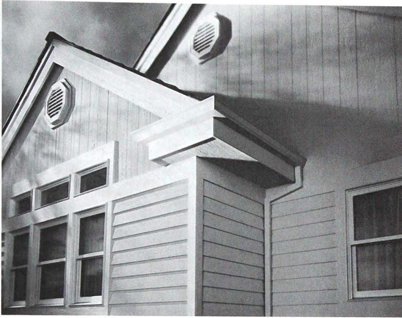
A variety of siding materials may be used for projects, including many solid wood products. Even better is engineered wood such as SmartLap Treated Engineered Wood Siding from Louisiana-Pacific. (Photo courtesy Louisiana-Pacific)
