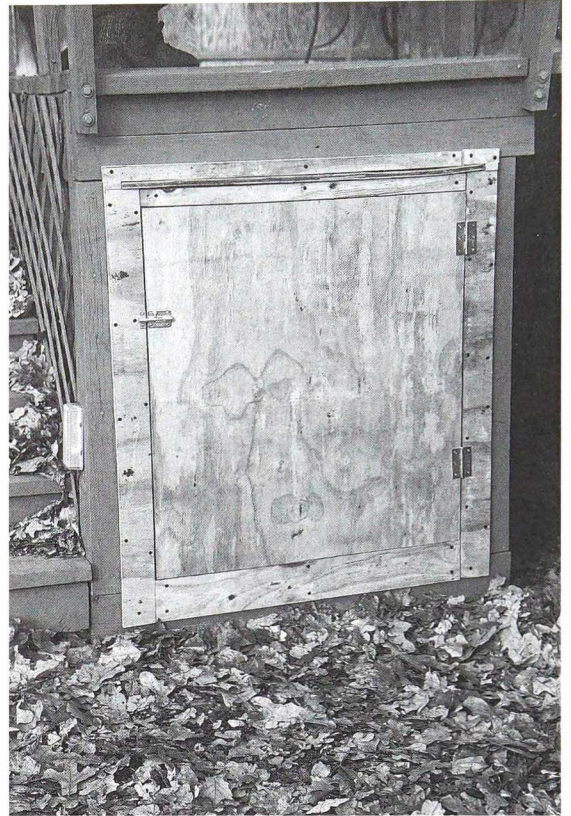
Under-deck pool and deck storage provides handy space for pool chemicals and deck objects. Made of pressure-treated wood, the unit is fastened to the deck and supported in the rear on 4-inch solid concrete blocks.
