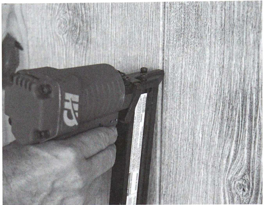
An air brad stapler makes it a cinch to attach siding.
