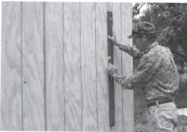
The angled cuts and door openings are marked from the inside using a small drill bit. A straightedge is used between the holes on the outside to mark the cuts.
