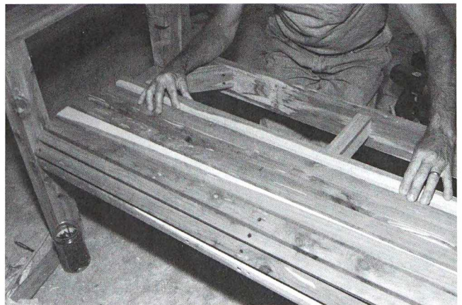
Then the seat slats are placed in position on the seat supports, spacing them properly.
