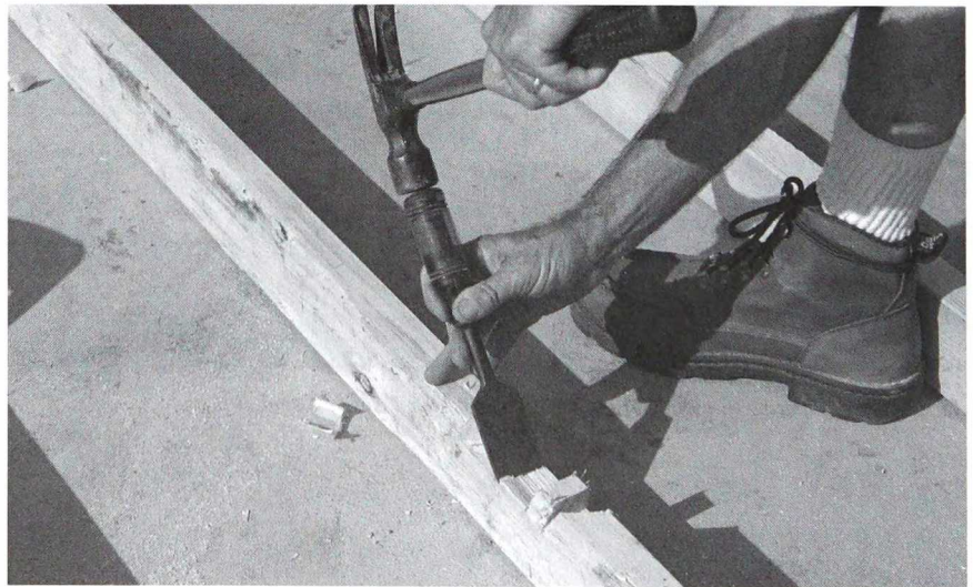
Then use a chisel to remove the material between the notches.
