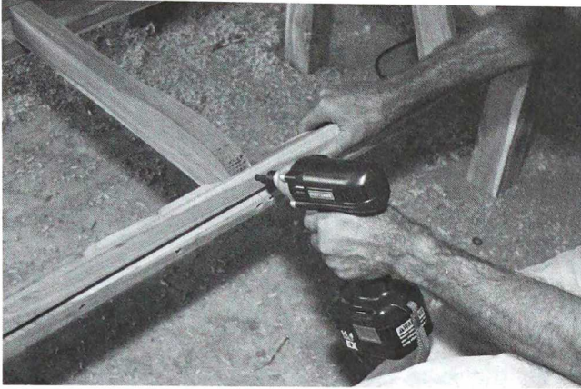
Slats are installed over the seat supports following the front curve of the seat supports.
