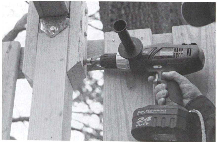
Bolt the monkey bars assembly and swing supports in place.
