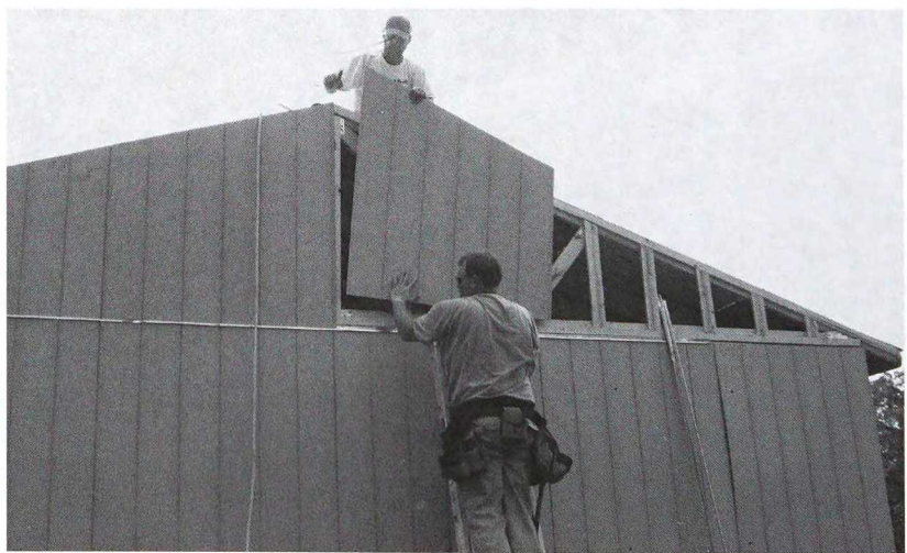
Siding is installed.
