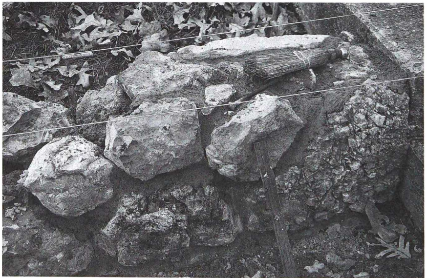
Before the mortar sets completely, excess mortar is removed with a round bolt head and a whiskbroom.
