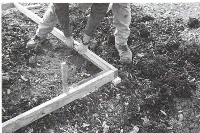
A temporary 2-x-4 bottom frame is used to lay out the project and locate the position of the four corner posts. It must be square.
