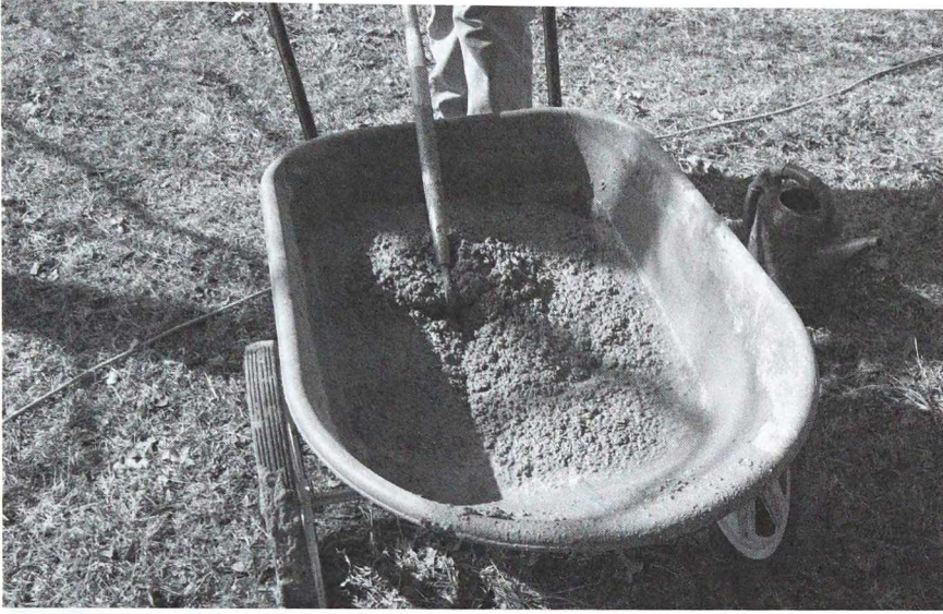
Pre-mixed bagged concrete such as Sakrete is mixed and poured around the posts.
