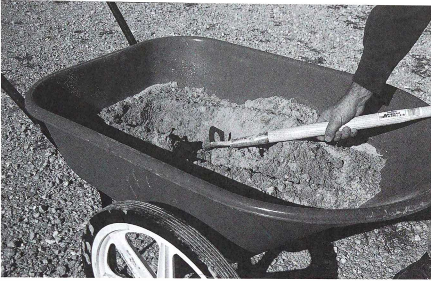
For mortared projects, such as a wall, mortar is mixed in a wheelbarrow using a mortar hoe.
