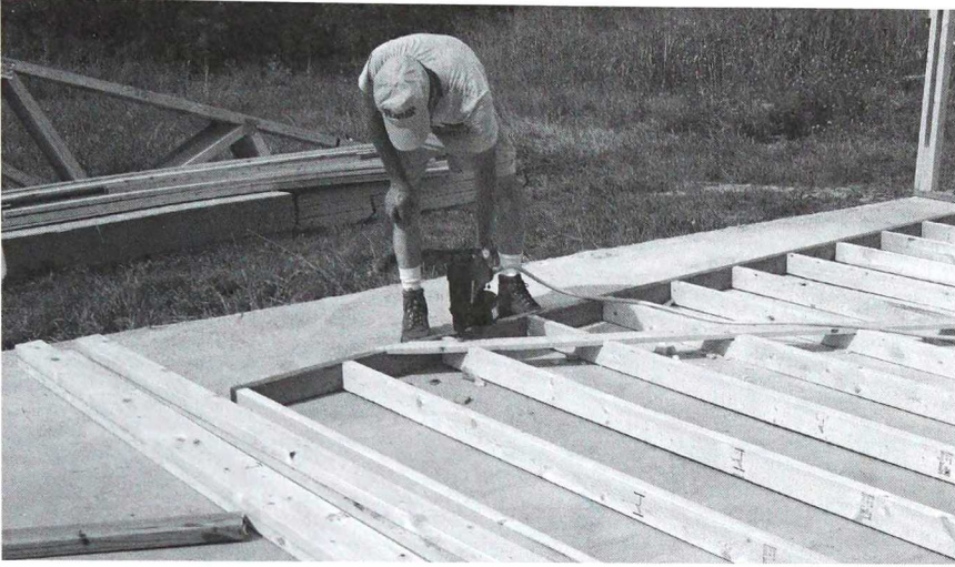
Make sure the wall section is square again, then fasten the wind bracing in place.
