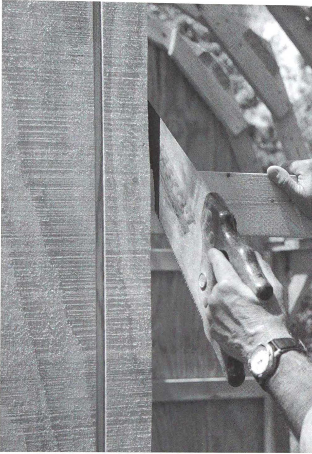
Complete the cuts on the girts with a handsaw.
