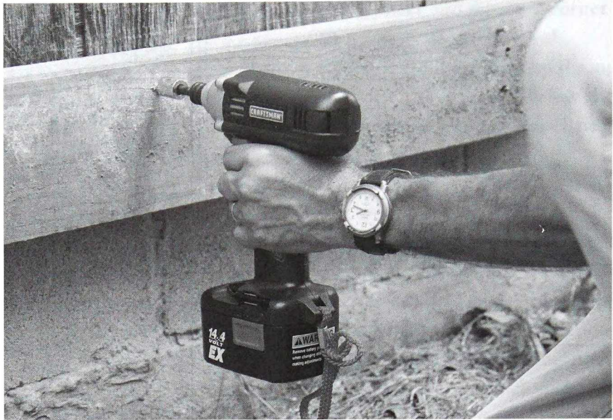
The Craftsman 14.4-Volt EX Impact Driver makes short work of driving lag screws to fasten ledger boards or beams in place. The variable-speed 1/4-inch reversible driver revolves and impacts simultaneously and delivers up to 850 pounds of torque.
