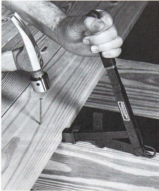
The BowJak from Vaughan makes it easy to install twisted, warped decking boards. (Photo courtesy Vaughan & Bushnell Mfg.)
