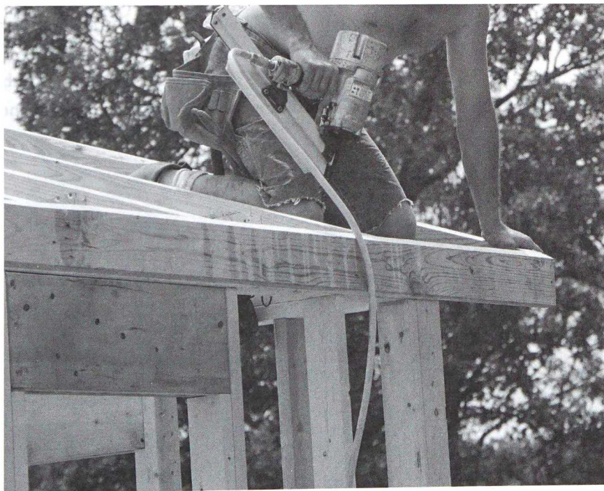
Rip 2-x-6 truss end supports to match the angle of the trusses and fasten in place. Then install the fascia.
