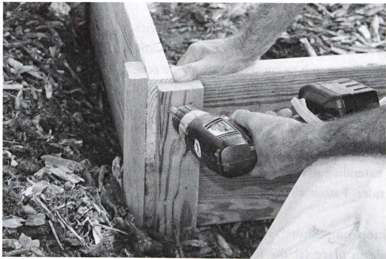
The corner blocks are used to fasten the sandbox corners together.
