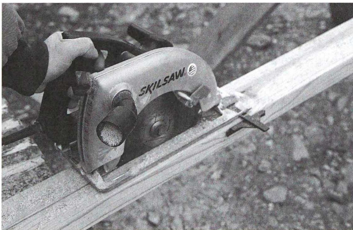
Some portions of the interior framing utilize 2 x 2s ripped from 2 x 4s. A portable circular saw and rip guide makes the chore easy.
