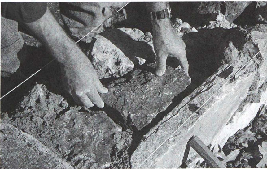
Rubble stones are used to fill out the center of the wall.
