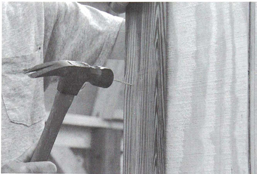
Finish details include adding the trim ripped from 1 x 12s.
