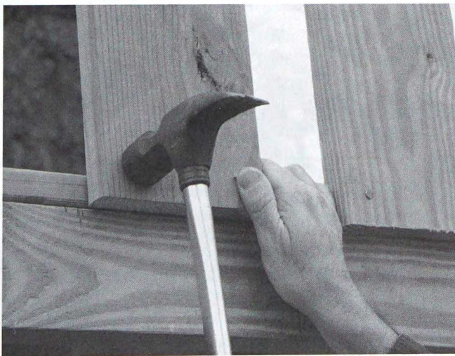
Assemble the upper rails and supports and nail on the sides.
