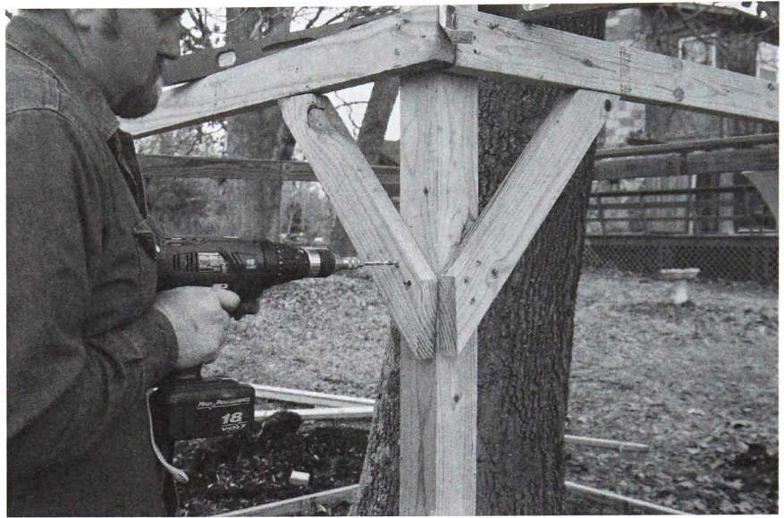
Once the poles have set, fasten the joist headers and braces in place with lag bolts.
