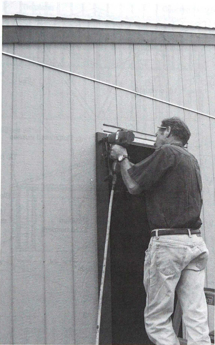
Trim is painted and installed.
