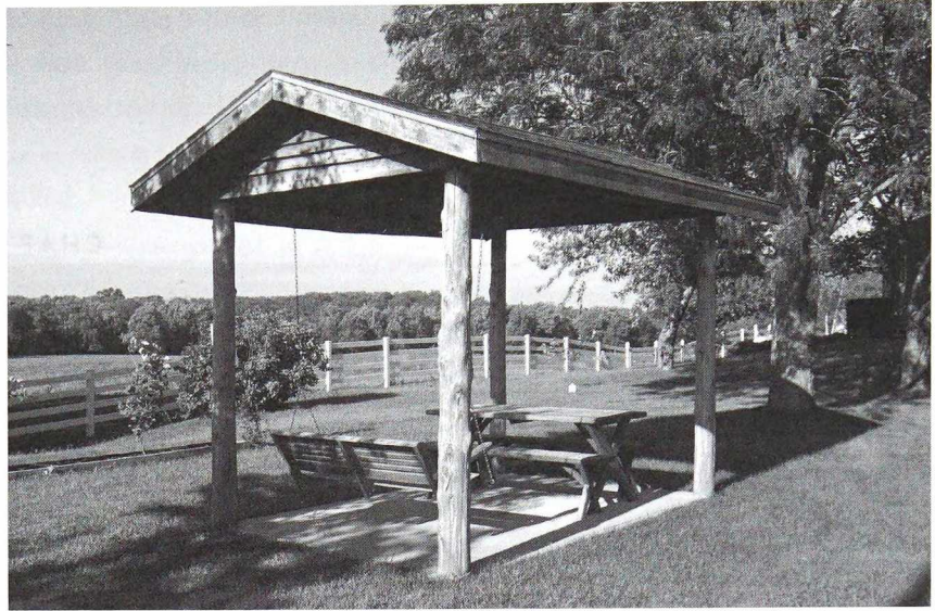
Picnic shelter shown is made of cedar log supports and rough-sawn cedar. It has a place for a picnic table, barbecue grill, and even has a porch swing support.
