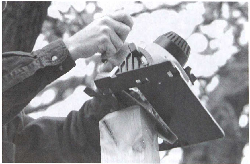
Cut 45-degree edges on all exposed posts, sand all edges, round all corners, and de-burr all metal.
