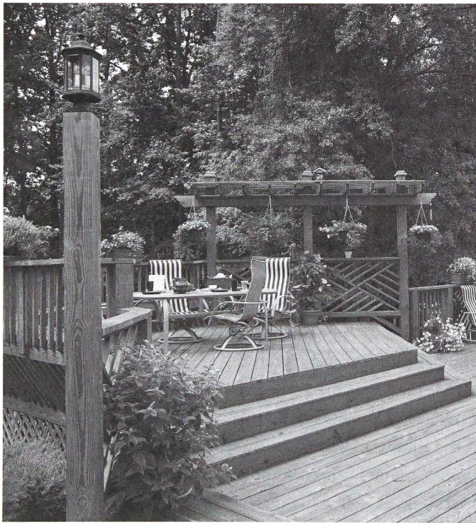
Decks must be constructed of a long-lasting material. Pressure-treated wood, such as Wolmanized Natural Select, is a good, long-lasting, economical, and readily available decking material. (Photo courtesy Wolmanized Natural Select wood)
