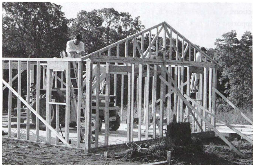
The first end truss is erected, fastened in place, plumbed and well braced.
