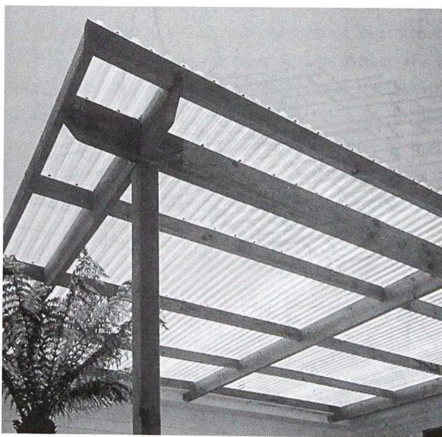
Sunshades can also provide water and weather protection if the framing is covered with materials such as Suntuf Sun 'N Rain PVC panels. (Photo Courtesy Suntuf, Inc.)
