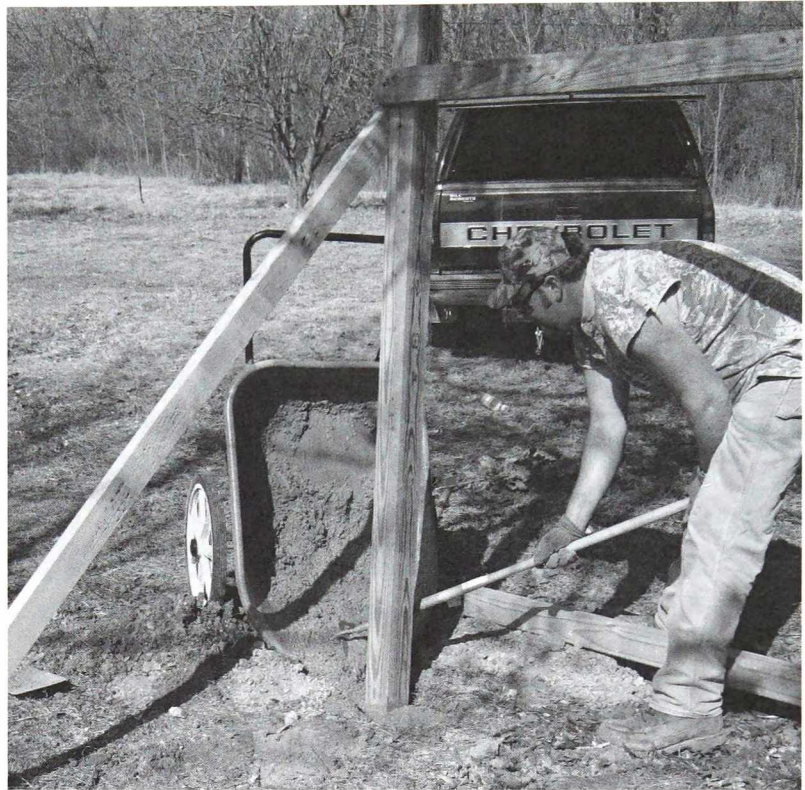
The posts are located for the monkey bars and swings. Holes are dug and concrete used to secure the posts.
