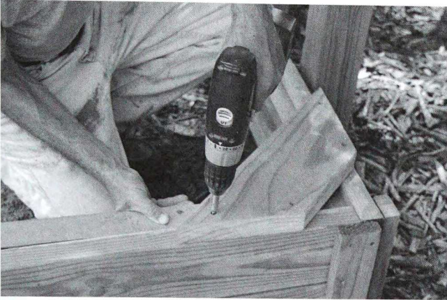
Seat boards also provide additional strength at each corner.
