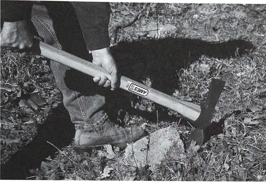
The first step in constructing a dry-laid patio or walk is to lay the stones in position and then dig a shallow depression to seat them.
