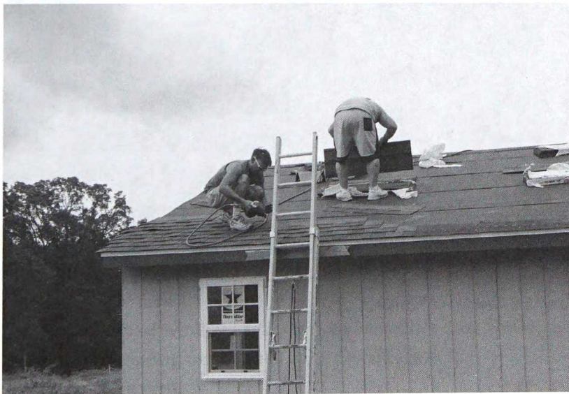
And the roof shingled.
