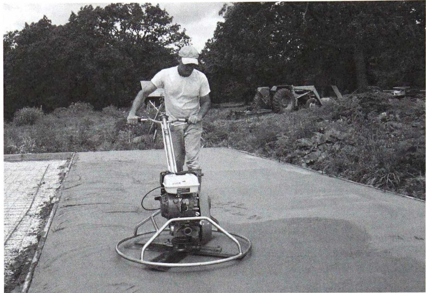
You can also rent a power trowel for finishing large surfaces.
