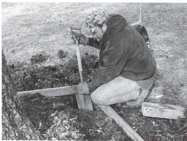
The support poles are located in each corner. Mark for the locations and dig the holes.
