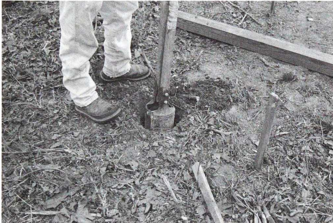
Dig the holes to the depth needed for your particular soil and region.
