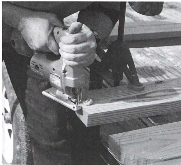
Construct the monkey bar. The first step is to round the ends of both the vertical and horizontal supports that attach to the fort.
