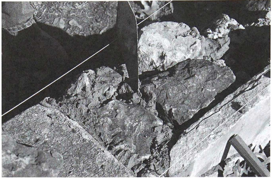
Mortar is applied over the rubble stones. Normally, only one course of stones is laid at a time.
