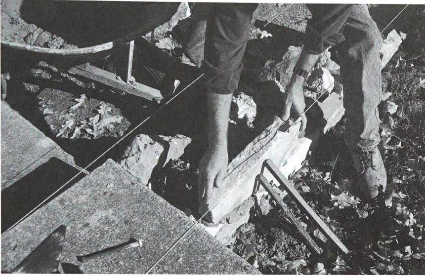
Thin stones are used as face stones. They are propped in place until the mortar sets.
