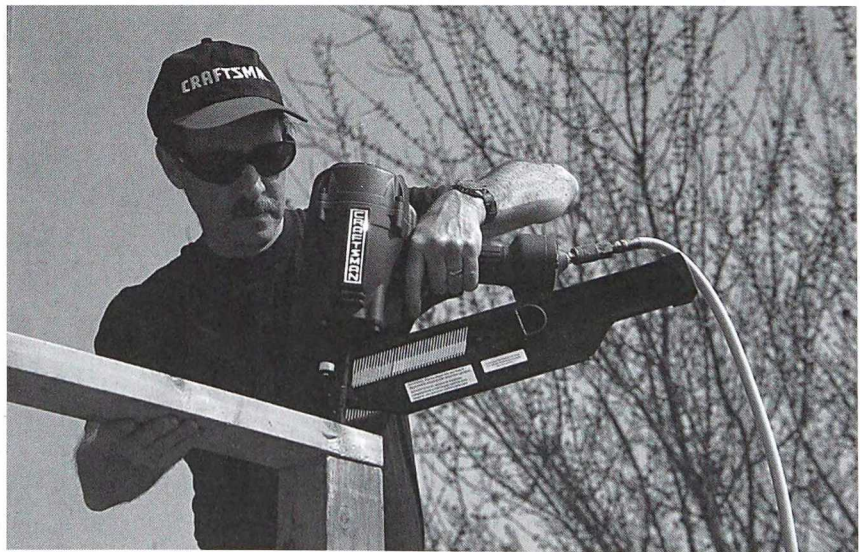
Craftsman lightweight 3½-inch magnesium framing nailer makes quick and accurate work of constructing the porch framing.
