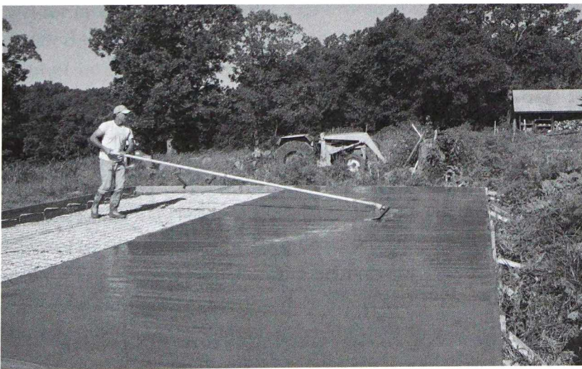
A bull float is used on larger pours.
