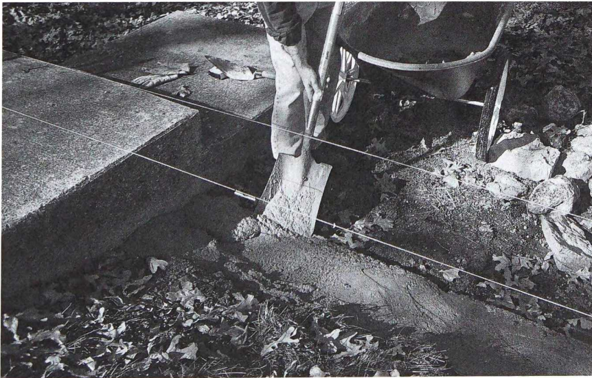
String lines are used to outline the wall and a layer of mortar troweled in place.
