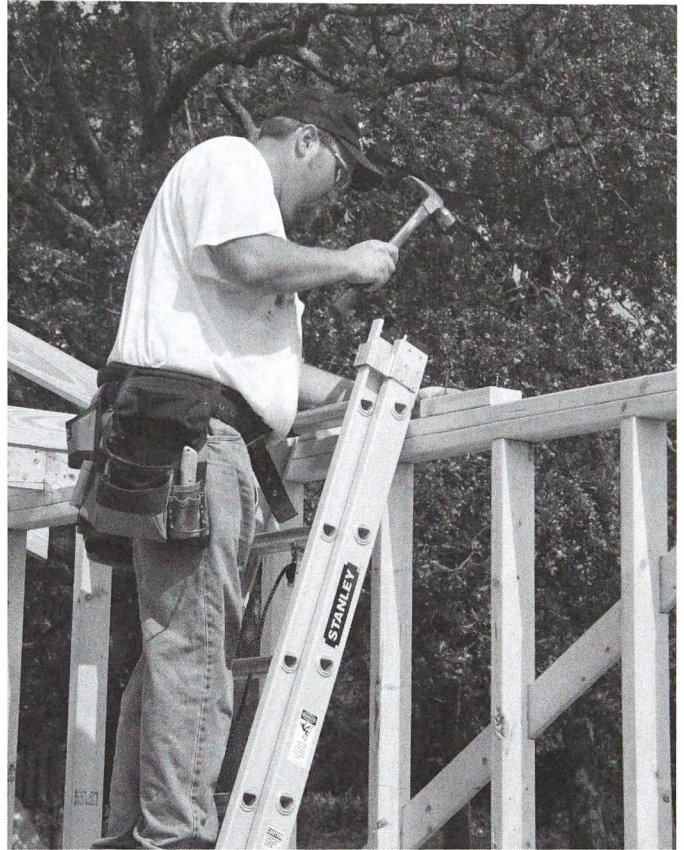
Blocks are nailed on the tie plates as a nailer and locator for the truss ends.
