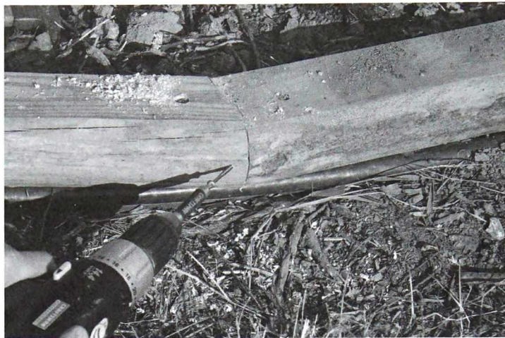
Joints can be further strengthened by fastening with brass deck screws.
