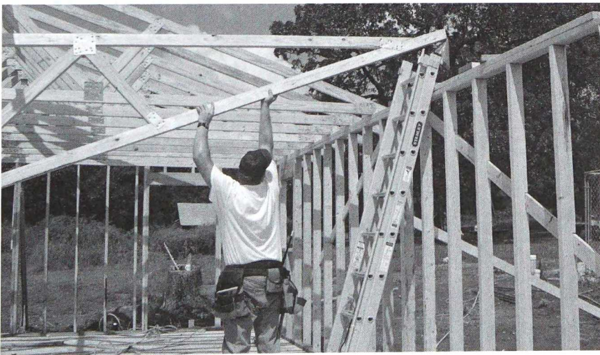
Trusses are heavy and you'll need at least three people to erect them. The truss ends are positioned up on the walls with the toe hanging down.
