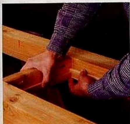
The inner faces of the stops are offset by \frac{3}{8} " to accommodate the overlapping lattice strips.
