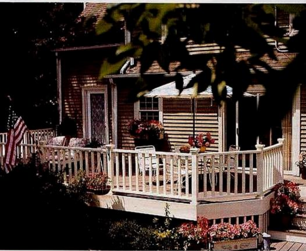
Decks that go beyond the concept of a basic platform are shown above and above right . Replacing the builder's obligatory concrete steps down to the yard, these elevated decks incorporate lattice to cover crawlspaces, stairs, and railings chosen to match the style of the house.
