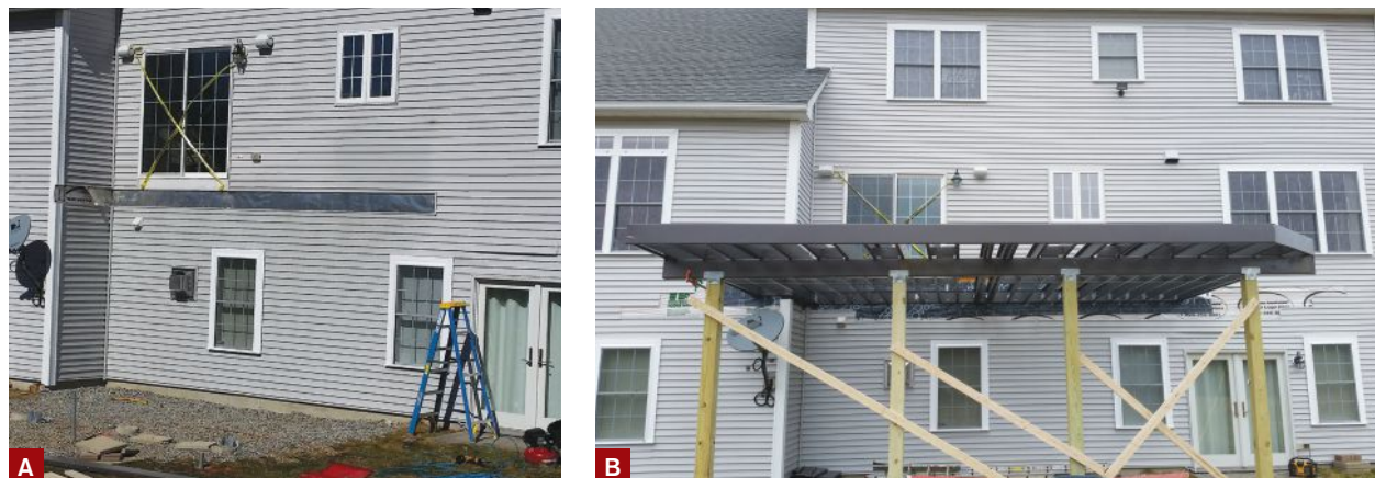
Figure 1. In the first phase of the project, workers removed the existing deck and installed new helical piles (A). The new deck was framed with Trex Elevations light-gauge steel, supported by 6x6 PT posts that bear on the helical piles (B). On the right-hand outside corner of the deck, the framing has been clipped at a 45-degree angle to accommodate the stairs leading to the upper level.
