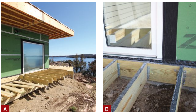
Figure 3. In the slab-on-grade areas, the wider grade-level deck section was framed with beefier 2-by stock (A). Threaded rod set in adhesive attached the ledgers to the top of the frost walls (B). Peel-and-stick capped the 2-by stock.
