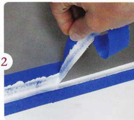
Carefully peel off the painter's tape, pulling away from the caulk to create a smooth bead.
