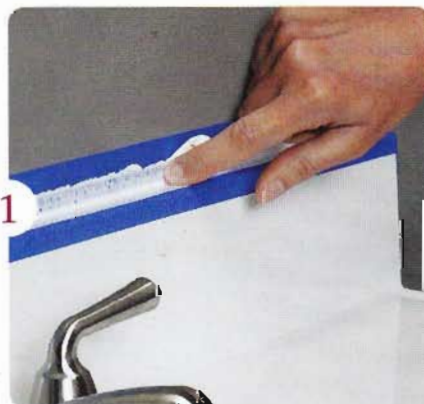
Smooth the bead of caulk with your finger. Get your finger wet first to prevent sticking.
