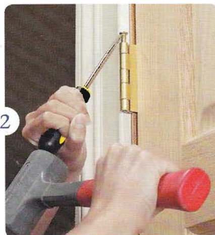
2 Pop the hinge pins out to take down the door and make it easier to work on.
