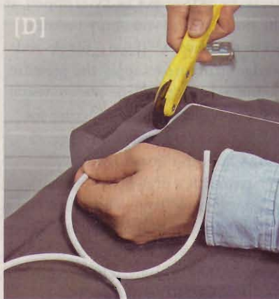
At the bottom of the frame, you'll need to remove the temporary spline a few inches at a time and then roll the permanent spline in right behind it.
