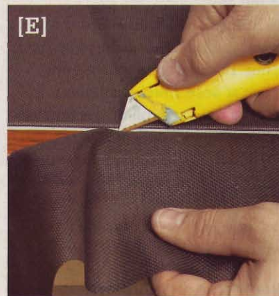
Use the inside edge of the spline channel to guide the utility knife when trimming the excess fabric. Be careful not to cut into the spline.
