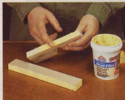
3] Fill the Edges. Just use your finger to fill any cracks or gaps on the edges with an exterior-grade wood filler.
