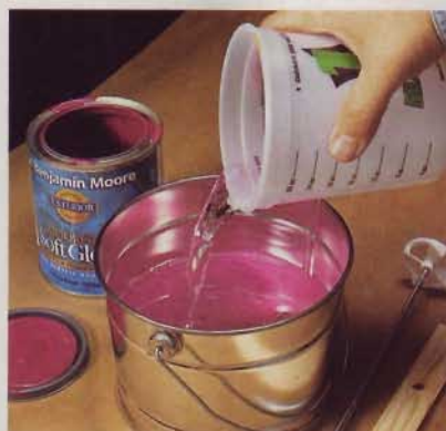
1] To thin latex paint for spraying, pour one quart of paint into a measuring pail. Then mix in four ounces of water.
