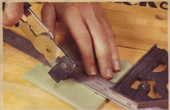
1] Using a combination square, measure 1\frac{1}{4} " from the bullnose edge and mark with a grease pencil. Hold the square on the marks and score a line with a tile tool.
