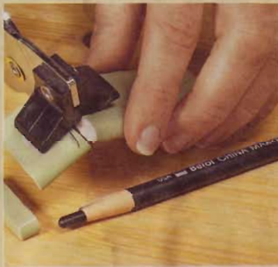
3] Score and break off a narrow piece on each end of the tile. Then score and break the strip into \frac{3}{4} "-wide pieces.
