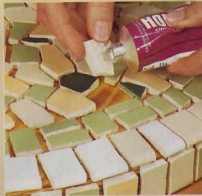
7] After completing the layout, start at the outside edge and glue each tile piece in place one at a time.
