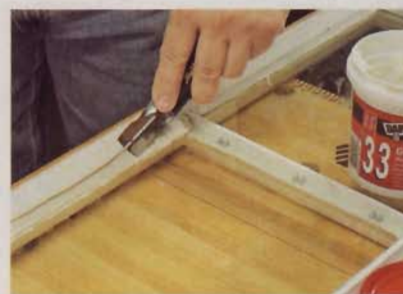
3] Pull a putty knife or glazier's tool along the compound to compress and smooth it into a consistent, beveled bead.
