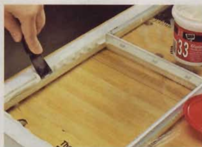
2] Secure the glass with glazing points. Then overfill the perimeter with glazing compound and press it into place.
