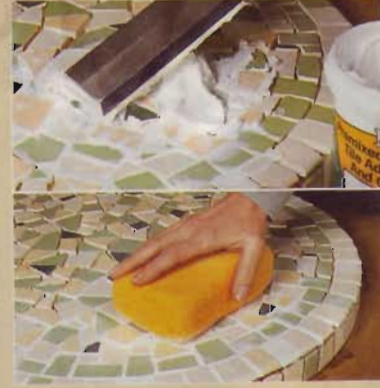
8] Apply grout to a small area. Let it set for about 10 minutes, and then lightly sponge off the excess.
