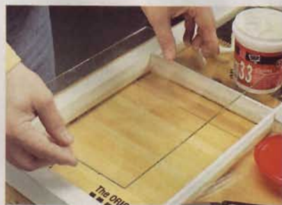
1] After priming, lay a thin bead of glazing compound on the glass stop, and then gently press the glass into the compound.
