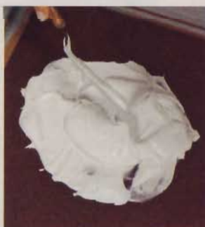
2] Mix drywall compound and primer together in a 3:1 ratio to thin it out.
