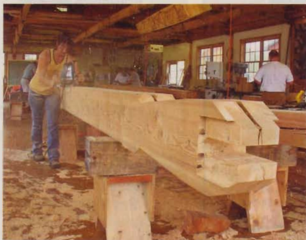
After cutting the intricate stepped mortises that will lock this massive timber in place, a student adds the finishing touches by rounding the sharp edges with a router.
