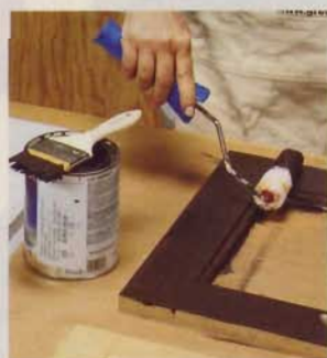
2] Apply a second basecoat with a 1/8" nap roller to create a smooth surface.
