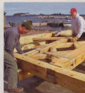
Students assemble a gable wall above. A timber frame gets raised below.
