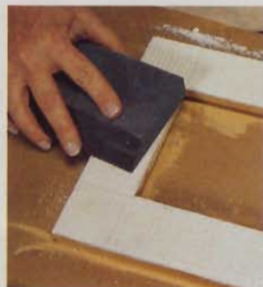
5] When the compound dries, use 220-grit sandpaper to knock off any high spots.
