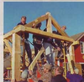
Students assemble a gable wall above. A timber frame gets raised below.
