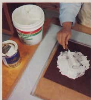
2] Thin three parts joint compound with one part primer to form a thin paste.
