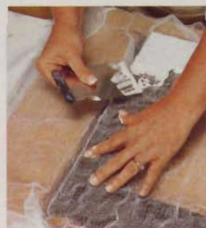
4] Apply an even coat of thinned drywall joint compound with a putty knife.
