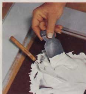
3] After mixing, load a Japanese scraper (shown) or a putty knife with compound.
