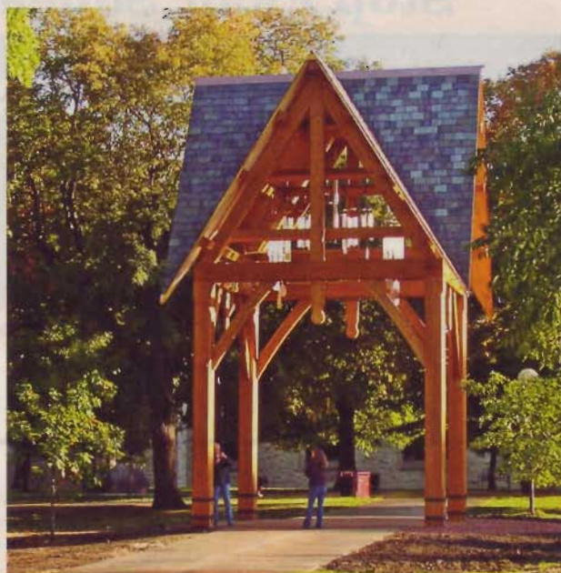
This timber-framed bell tower was built by students in a workshop at North House Folk School. Then it was transported to St. Olaf College in Minnesota and erected on-site.
