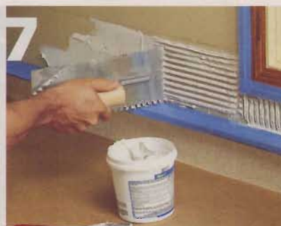
7] Use a notched trowel ( \frac{1}{4} " or \frac{3}{8} " should be fine) to spread an even bed of tile adhesive along the walls.
