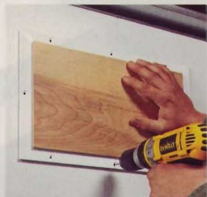
10] Position the inner window trim with the jig. Then use the mounting holes as a guide when drilling the pilot holes.
