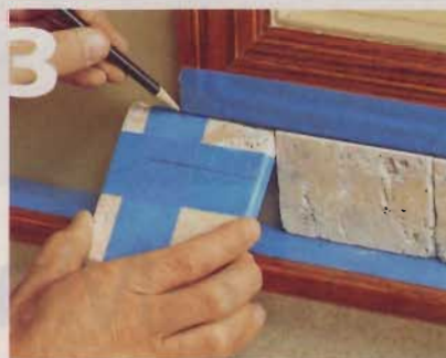
3] Now mark the tile to match the remaining space between the adjacent tile and the edge of the window trim.
