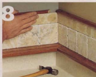
8] After the tile adhesive has dried, miter the cap pieces and nail them in place over the top of the tile.
