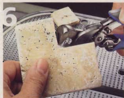
6] The tile saw won't be able to cut a perfectly clean corner, so you'll need to square up the corner with hand nippers.
