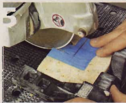
5] Now go to the tile saw, and cut the notch in the tile to fit around the corner of the window.
