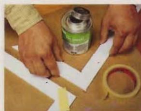
3] Glue and tape the miter joints on the trim pieces.
