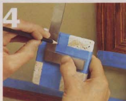
4] After marking the width of the cut, you'll need to extend this line to meet the other cut line.
