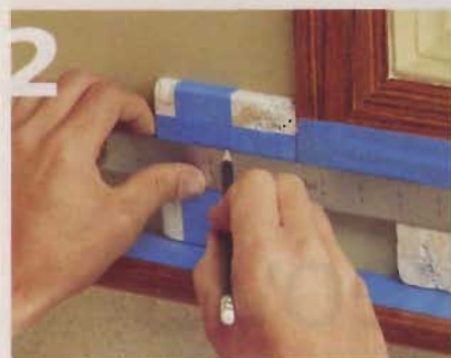
2] To lay out the corner cut, first mark a tile to match the space between the bottom of the window and the plate rail.
