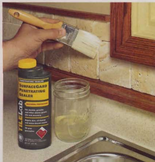
Porous tile and the wet conditions in the kitchen mean a couple coats of tile sealer are in order.
