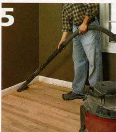
5 VACUUM DUST Once the entire floor is sanded, vacuum the dust using a
