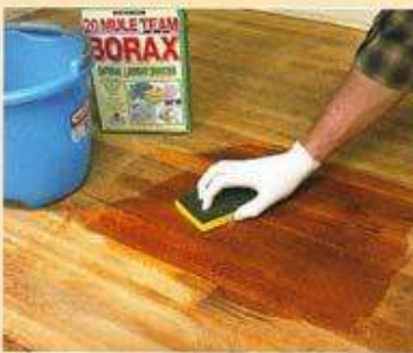
2] Once the stain is removed, scrub the area with a borax and hot water solution to neutralize the acid.
