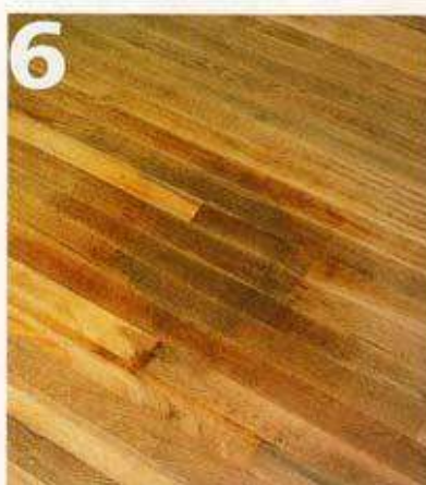
6 REMOVE STUBBORN STAINS If any stains remain after sanding, use wood bleach to remove them (see page 63).
