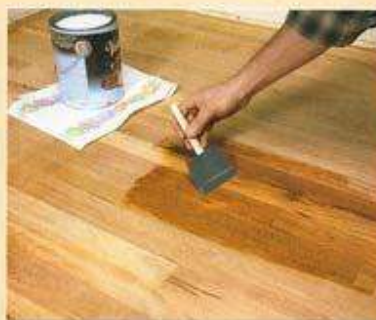
3] To make sure acid residue won't react with the finish, brush on a thin test coat of finish.
