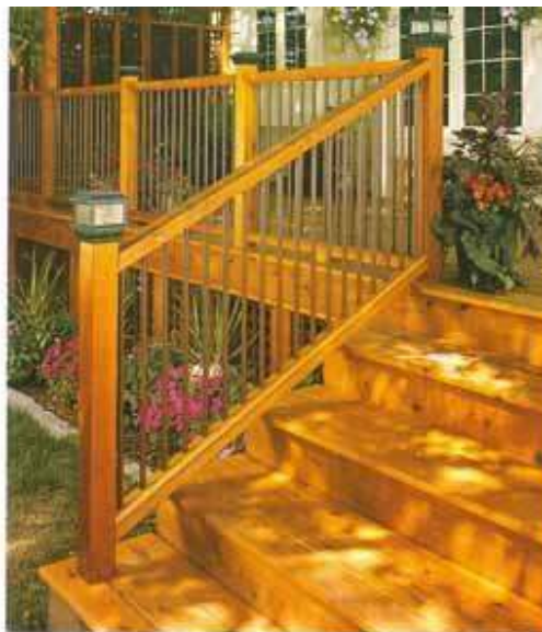
When mounting the stair rails, align the upper ends with the rails on the deck. Then drive screws into the posts to secure the rails.
