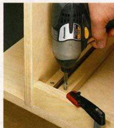
Use a piece of scrap to set the guides back the perfect distance from the front of the case.
