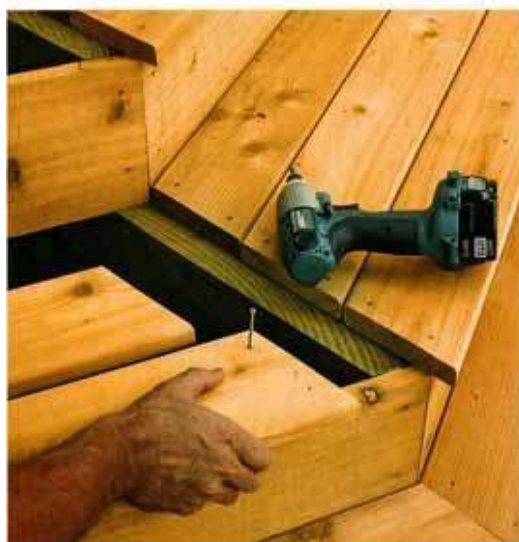
The treads are mitered at 22\frac{1}{2}^\circ to wrap around the corner and secured with almost-invisible trimhead screws.
