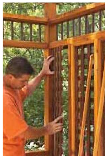
Lattice screens fit between the pergola posts to add privacy to the deck. Mitered frames secure the screens.
