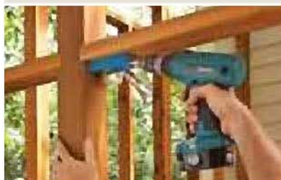
The balusters get mounted between the rails (above). Pocket holes in the rails accept mounting screws (below).
