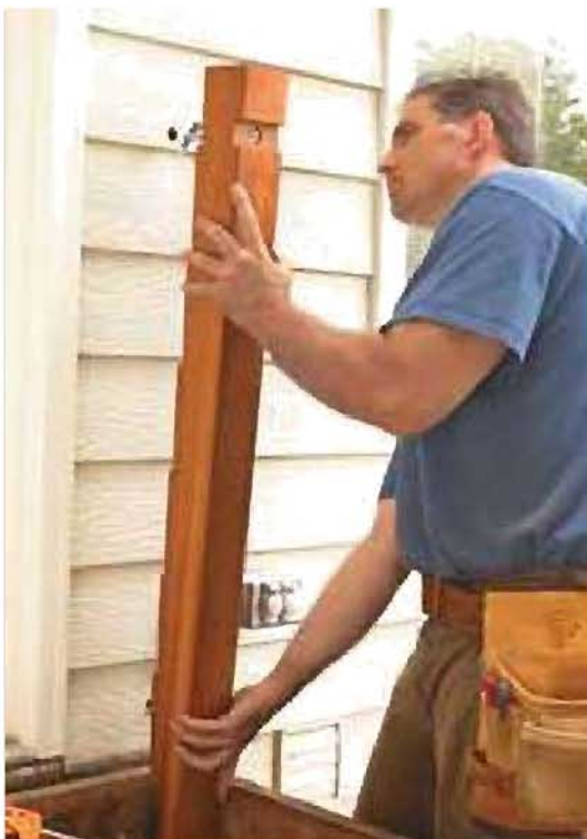
The posts that sit against the wall get bolted in (above). The others mount in dadoed "saddles" (below).
