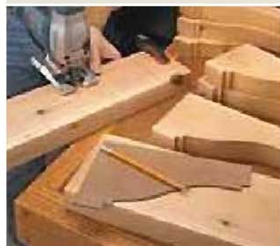
The decorative tails on the pergola make it look like the beams and rafters are notched to fit together ( above ). But the tails are simply cut to shape ( below ), and then attached.
