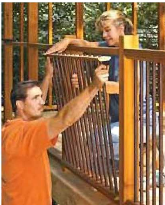
The balusters get mounted between the rails (above). Pocket holes in the rails accept mounting screws (below).
