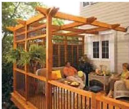
The decorative tails on the pergola make it look like the beams and rafters are notched to fit together ( above ). But the tails are simply cut to shape ( below ), and then attached.
