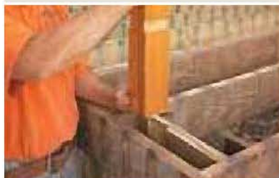
The posts that sit against the wall get bolted in (above). The others mount in dadoed "saddles" (below).
