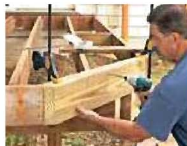
After cutting off the the corner, screw on two 2x8s to form the 45° angle and reconnect the joists.
