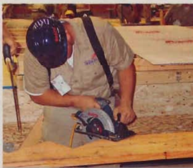
A SkillsUSA participant cuts a stair stringer that will lead to the second story of a partial home.
