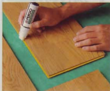
▲ Moisten the plank tongues with tap water and watch for the glue color to change.
