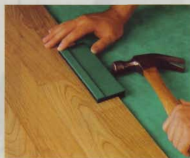
▲ Use a hammer along with Pergo's tapping block to tap the planks into position.
