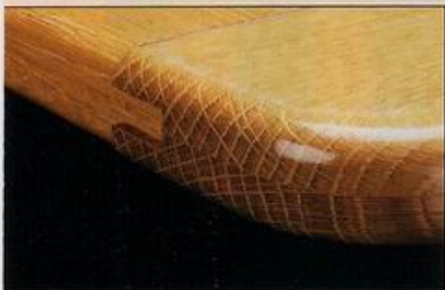
▲ During dry winter months, a solid-wood panel will shrink, recessing the tongue in the breadboard end.
