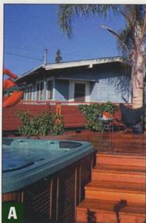
▲ The elevation of the deck is used to integrate a spa without the need for additional structure.
