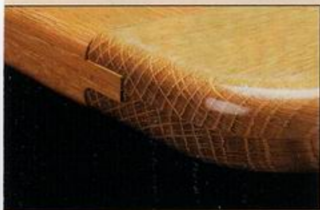
▲ A solid-wood panel will swell during humid months, causing the tongue to extend past the breadboard end.
