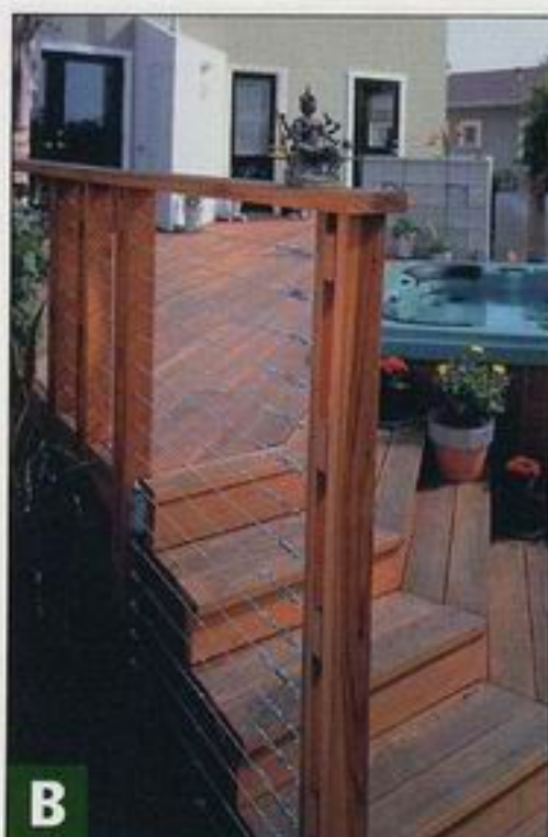
▲ Cables strung between redwood posts and secured with turnbuckles create a striking border to the deck.
