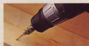
Drill pilot holes
