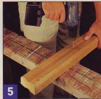
5 Layout the centers of the slats (every 3") along the groove in the screen cap. Drill a \frac{1}{8} " pilot hole at the marks.
