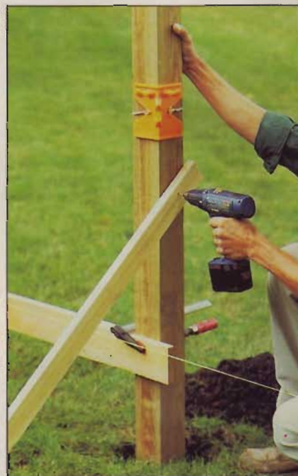
Setting Fence Posts - 34
