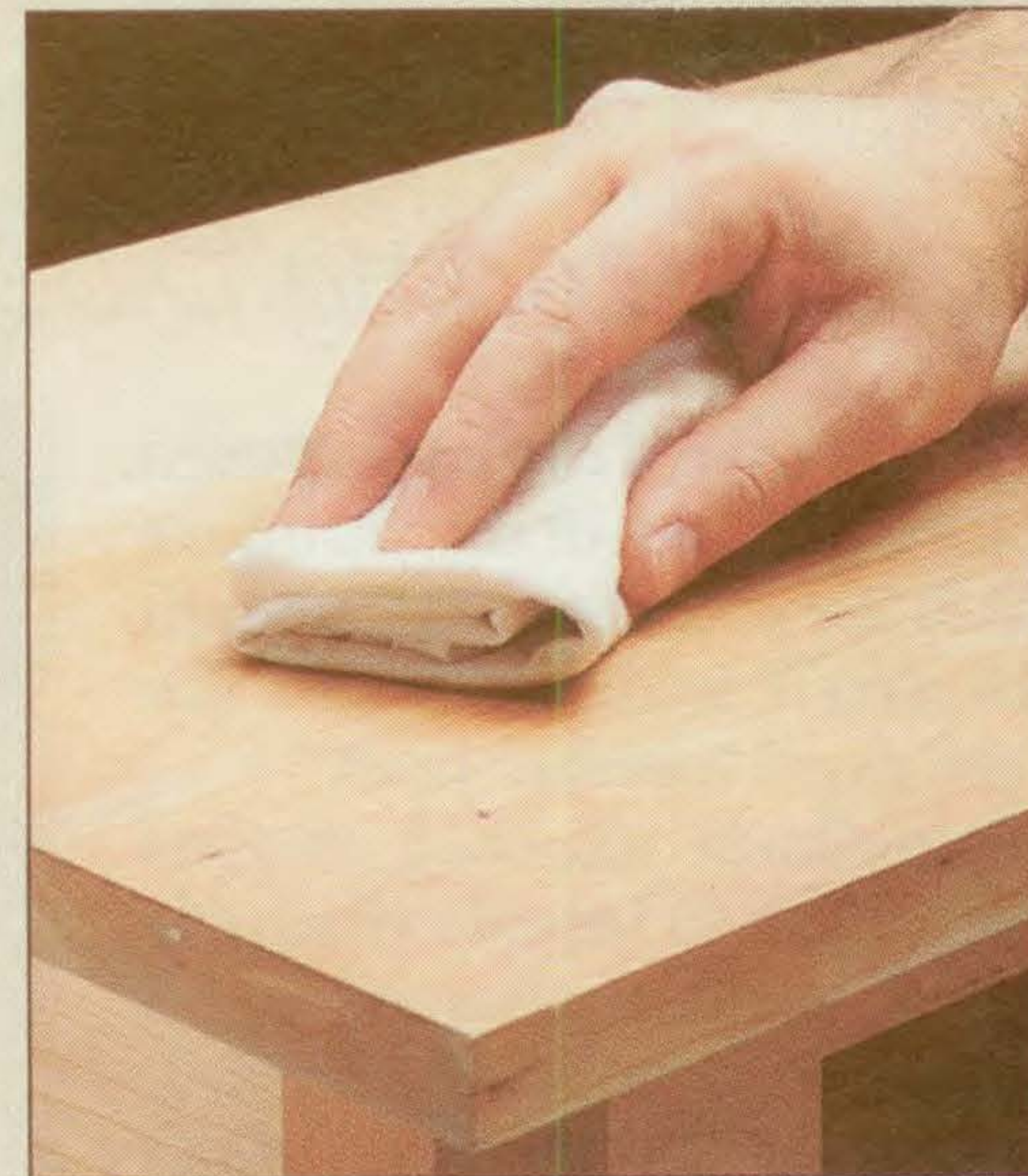
F. Wiping down the surface with a rag soaked in mineral spirits reveals stray glue smudges.
