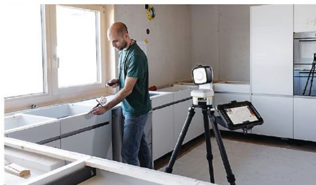
The Leica iCON, combined with a vPen, produces a digital template that can be used to program a CNC machine.
