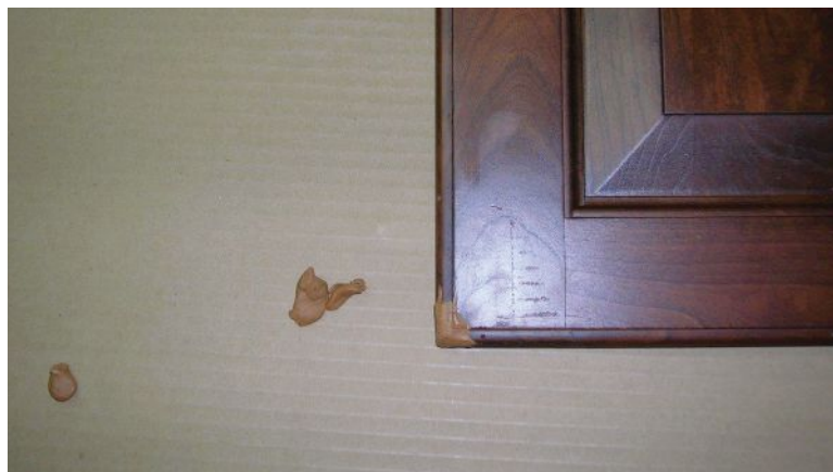
Epoxy stick can be shaped or smoothed with your finger or a tool moistened with water.
