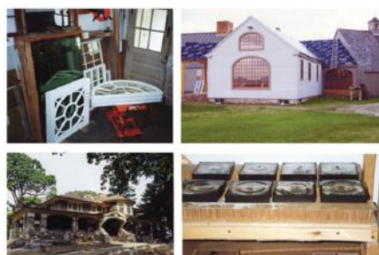
Clockwise from top left: Shaped sashes being restored, residential windows, residential sash replacement, and bullseye insulated units by Green Mountain Glass.
