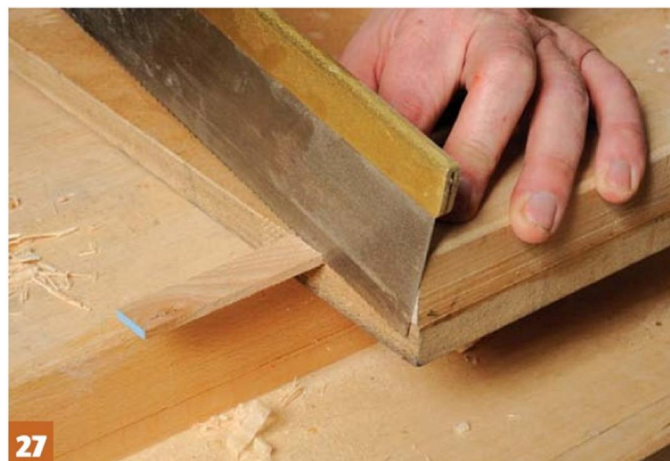
27 I cut the upstands to length on my back saw
