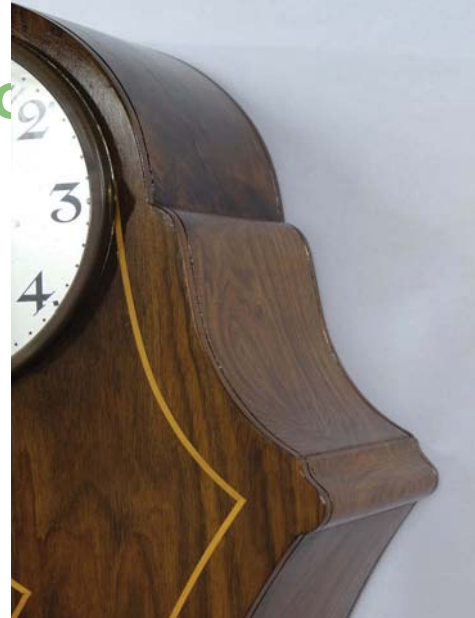
Stringing detail and case profile showing the applied moulding
