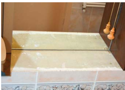
Ready for the sill to cover the exposed tile edges
