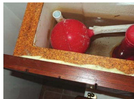
To bond the framework to the varnished tank boxing, PU glue was used
