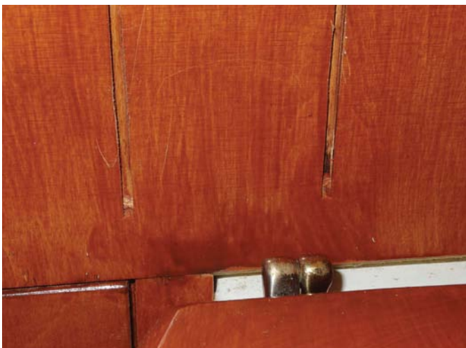
Shallow slots were cut into the ply
