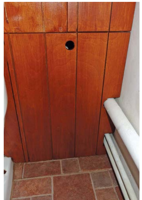
The panels were then cut to fit around the pipework
