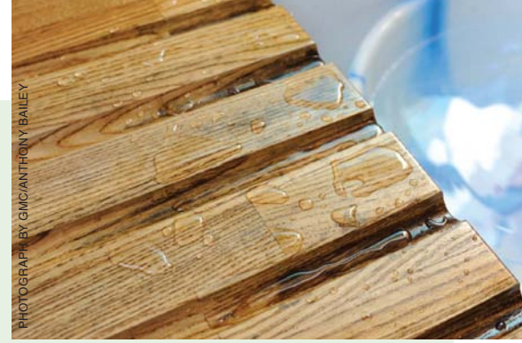
A wooden sink top surface with drip grooves
