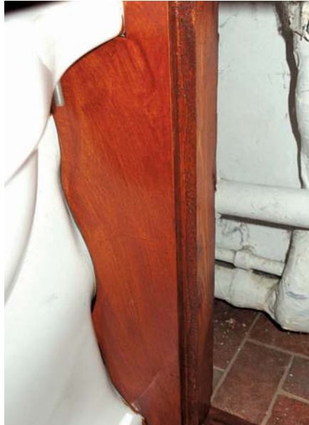
Two pieces of ply were cut to fit around the rear of the bowl
