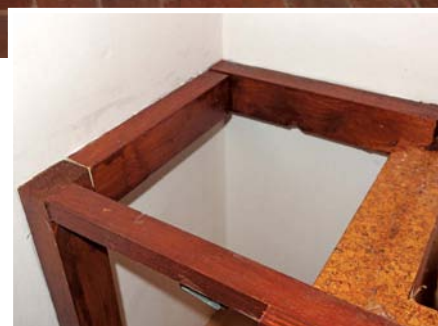
The framework was bonded to the walls using a builder's mastic adhesive
