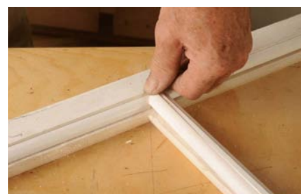
Here I am fitting a glazing bead into the rebate
