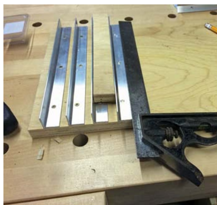
A block was used to get the correct spacing
