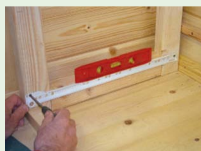
Attach the bottom drawer runner component in place on the frame
