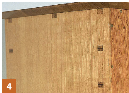
Through-tenoned top and bottom drawer and centre rails are unconventional, but are in keeping with the wedged-through tenons
