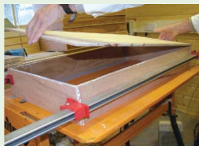
Cramp the drawer frame, run a bead of adhesive around its bottom edge, then position a 9mm drawer bottom
