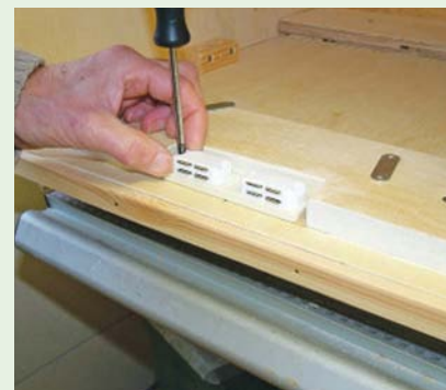
Magnetic catches provide an easy, effective closing mechanism
