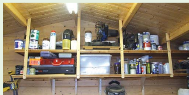
Even greater support is achieved by attaching shelves to braces that are themselves attached to the ceiling members
