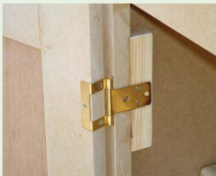
Cranked hinges provide a secure fitting – especially useful when used with MDF
