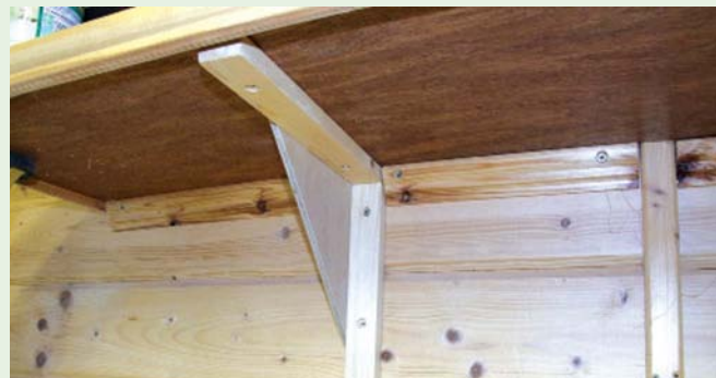
For larger shelves, an effective bracket can be made using a pine 'L' and braced using a plywood triangle
