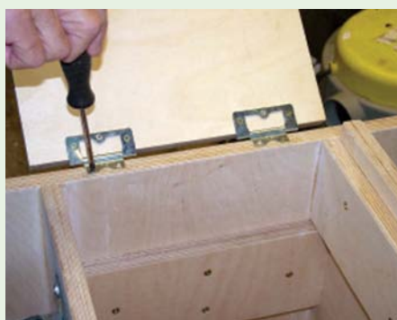
The door is attached to the carcass using flush hinges. Simple handles can be made by sticking spacers to a handle bar
