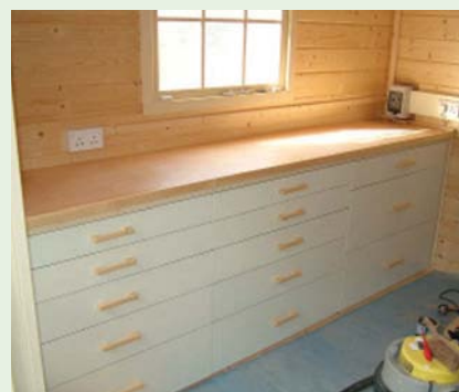
The 18mm plywood panel is attached to the top of the unit using screws. A pine edging is attached to the front, and three coats of water-based clear floor varnish are applied
