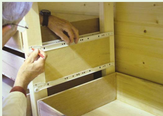
Continue to attach the drawer runners using a temporary ply spacer
