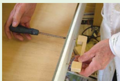
Attach to the drawer or door with screws that extend through to the bar
