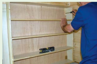
The unit is screwed to the wall
