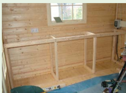
The frames are attached at the required drawer length using cross members. The whole assembly is attached to the walls for built-in units
