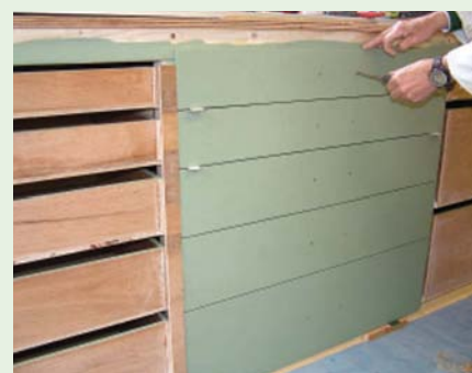
False fronts can be added. Ensure adequate spacing by using 2mm spacers. Use screws through the holes that will be used for the handles
