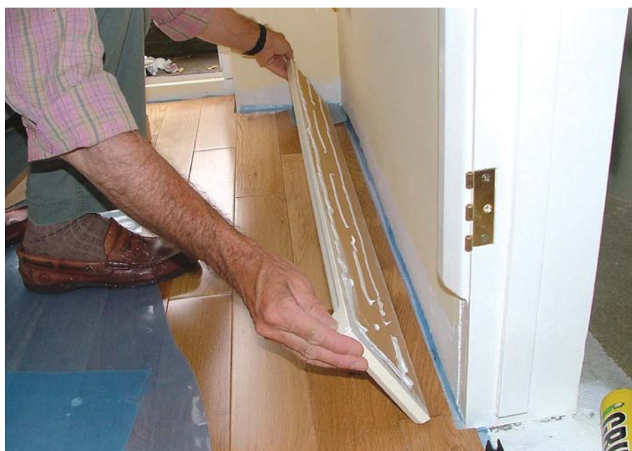
Fix in position by pressing the lengths against the wall, then give a slight side-to-side movement to bed in place
