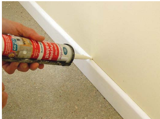
Finish the job with a neat seal using polymer sealant ■
