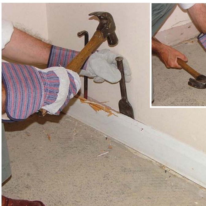
A bolster chisel and hammer can be used to lift any gripper...
