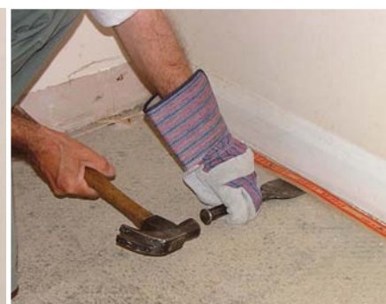
A bolster chisel and hammer can be used to lift any gripper...
