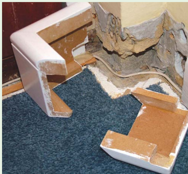
The sections are formed and attached to the wall using a grip adhesive
