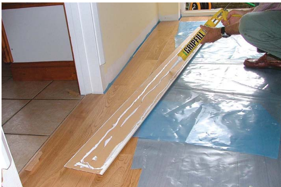
Apply gap-filling adhesive to the rear of each length of skirting in turn
