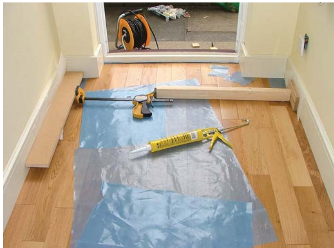
You may find it necessary to hold the skirting in place, especially if the wall is uneven or bowed
