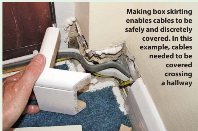
The sections are formed and attached to the wall using a grip adhesive
