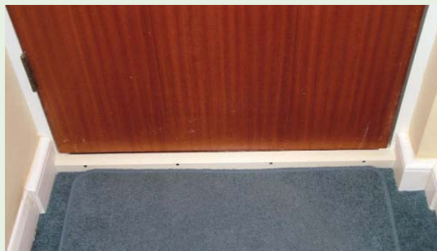
The end result provides a safe route for services, and gives a smooth transition
