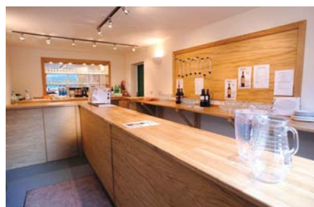
The village hall bar fit in solid oak and oak-veneered MDF, finished with two part clear lacquer
