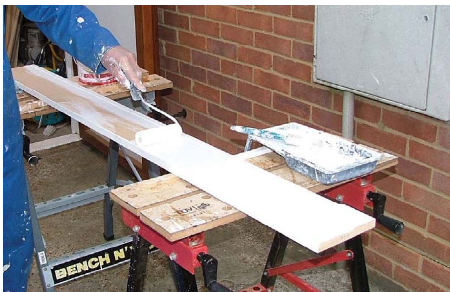
When all the lengths are cut to size and dry checked, apply sealer, primer, undercoat and the required finish
