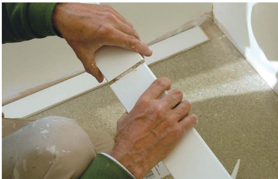
If longer lengths are required, skirting can be joined using biscuits and adhesive
