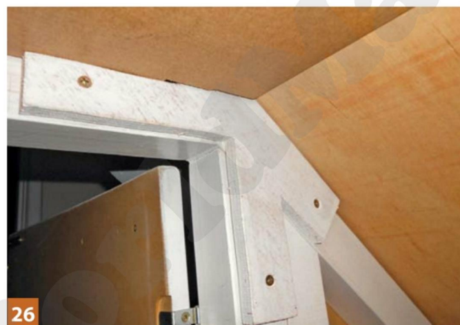
26 A look at the support plate used in the under-stairs cupboard
