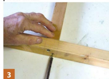
3 Screw and adhesive joints are adequate
