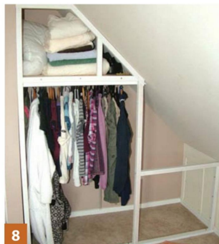
8 The frame is fitted into position
