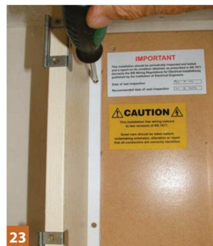
23 Attaching the box frame to the mounting board
